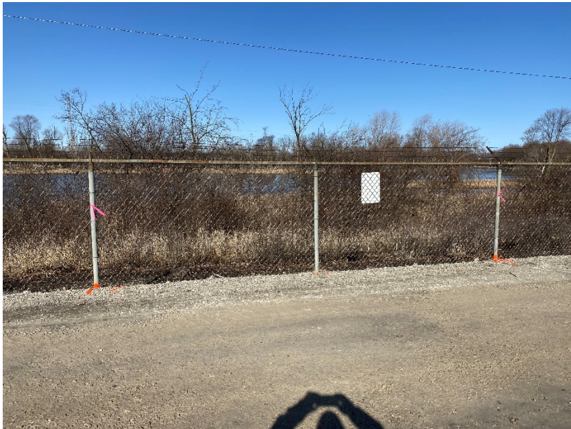
3. Slope protection near Pond 3S west
