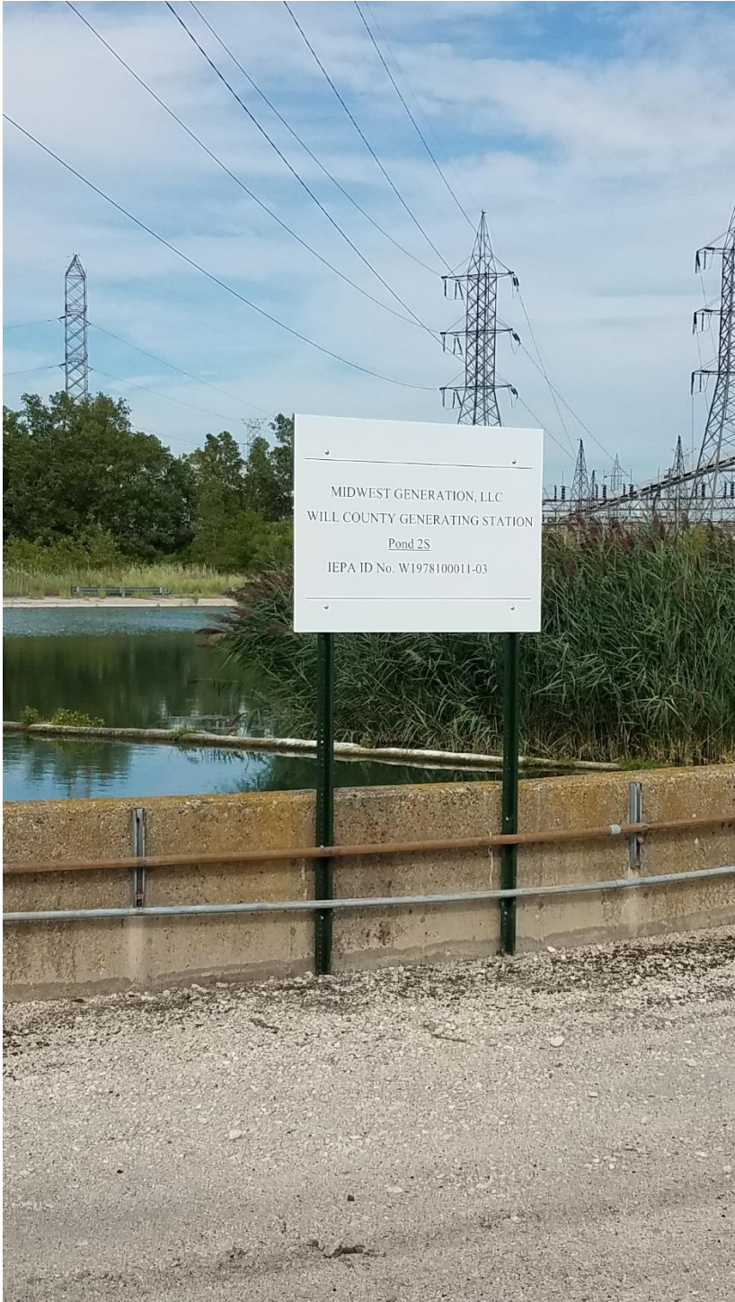
1. Ash Pond 2S Posted IEPA ID Sign
