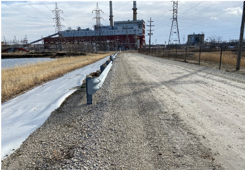
1. Slope protection Pond 3S south
