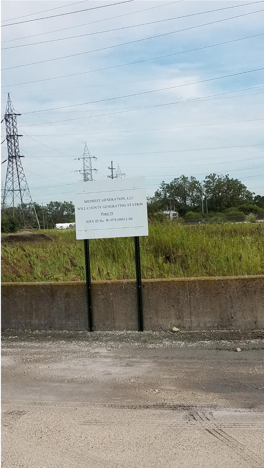
1. Ash Pond 3S Posted IEPA ID Sign
