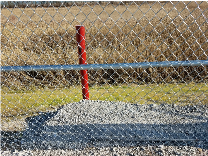
7. Slope protection near MW-4
