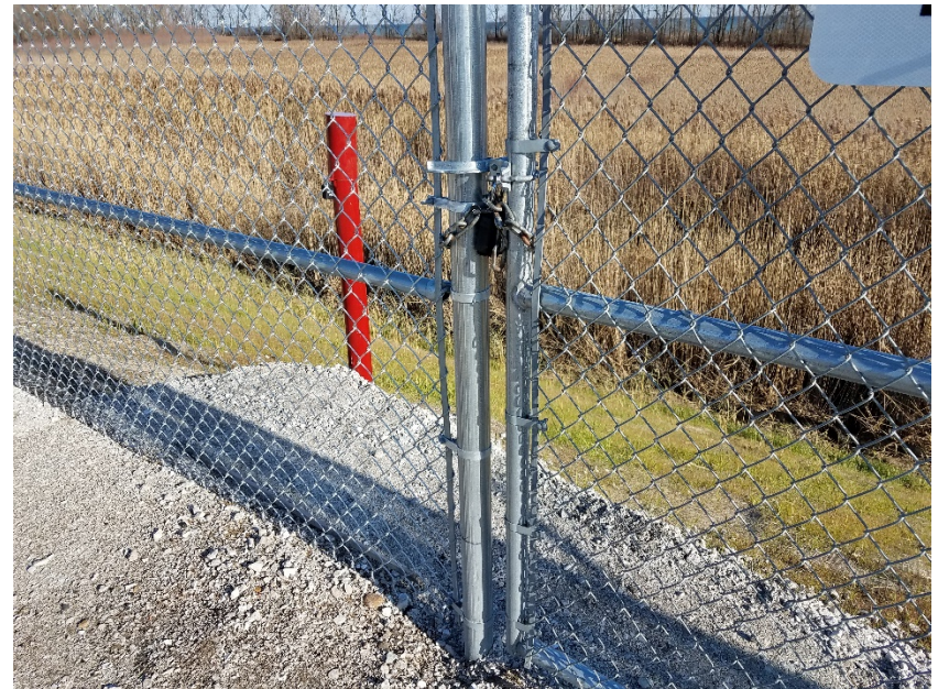
8. Slope protection near MW-4
