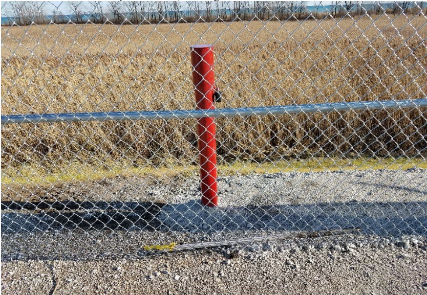
5. Slope protection near MW-3
