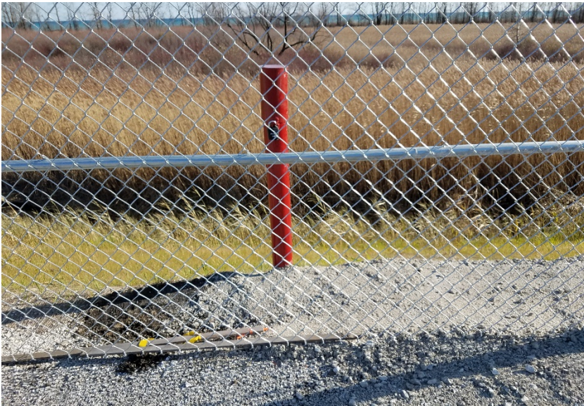
1. Slope protection near MW-1
