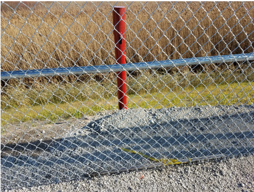
3. Slope protection near MW-2
