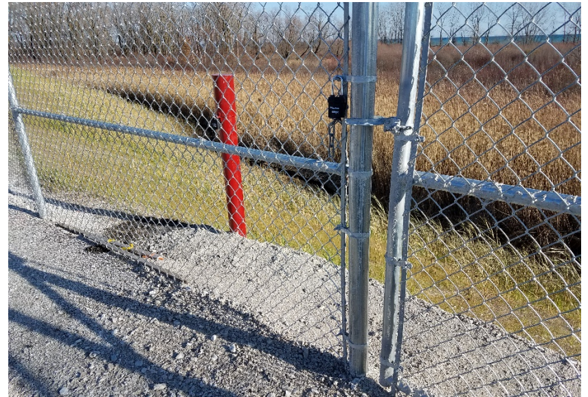
2. Slope protection near MW-1
