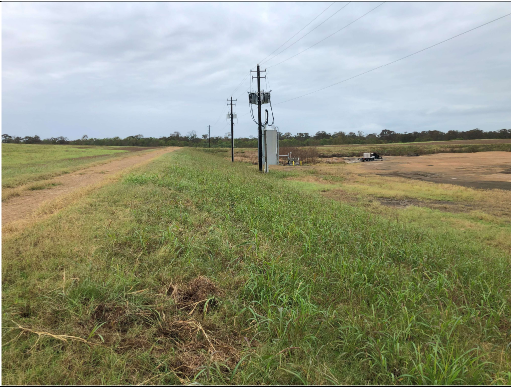
Photograph P-5: View looking west along the interior of the southern berm Cell 2A. This interior slope is well vegetated without erosion issues.
