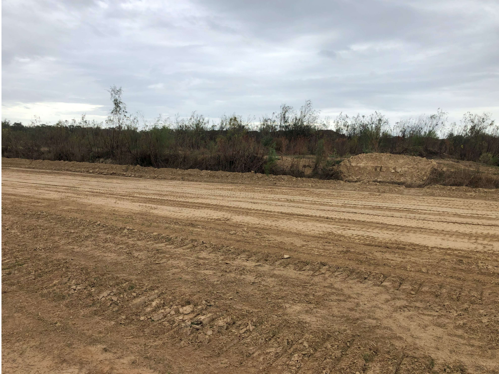
Photograph P-10: View looking southeast along the northern berm of Cell 2B. The tan material visible here is scrubber sludge.
