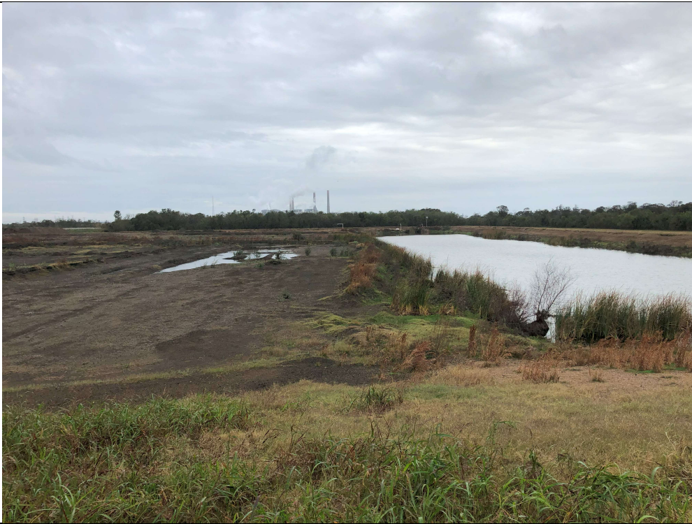
Photograph P-1: View looking south at Cell 3 from top of its north berm. This view is directly of an area where bottom ash material has been excavated and sold as road base. The Cell 3 storm water pond is visible to the right. The interior slopes and crest roads of the berms are either vegetated (slopes) or have been stabilized with a cemented fly ash mixture.
