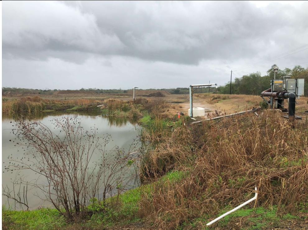
Photograph P-2: View looking east from Cell 3's southwest interior corner. The crest road was well maintained, exterior slopes well vegetated without erosion issues, and interior slope either improved with stabilized CCR material or vegetated.
