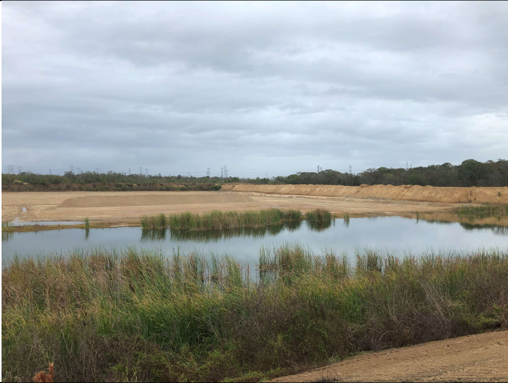
Photograph P-11: View looking north across contact water pond from Cell 2B's southern berm. The vegetation in the pond is controlled on an as needed basis. Stockpiled fly ash is visible to the north of the pond.
