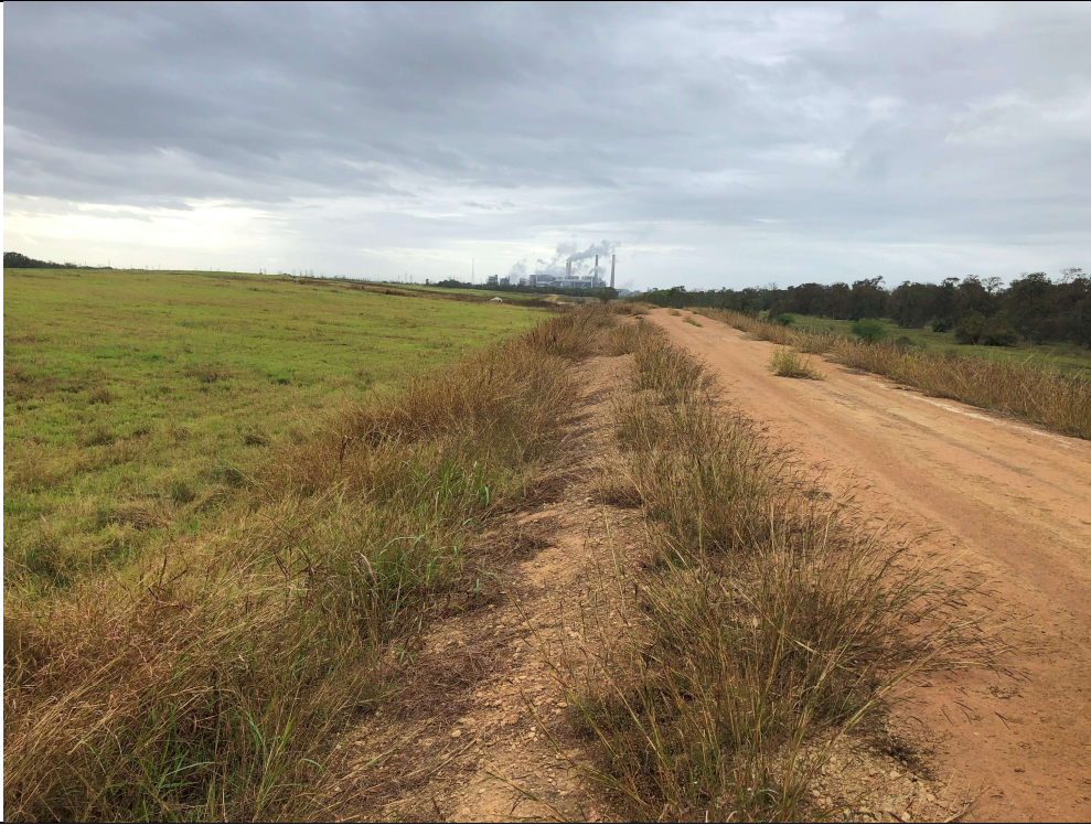
Photograph P-9: View looking south along the western berm of Cell 1C. The area closed in 2022 is visible to the left, and the berm crest road visible to the right. No significant rutting was observed.
