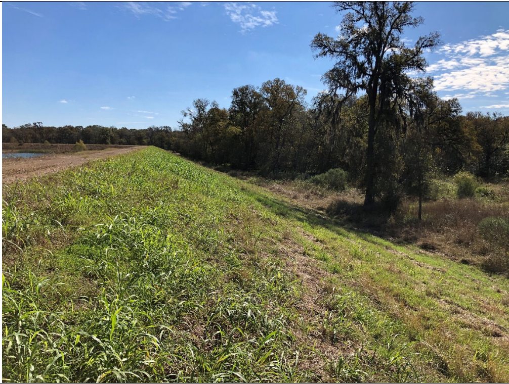
Photograph P-11: View looking southeast of the exterior slope of Cell 2B's southern berm. The exterior slope is well vegetated.
