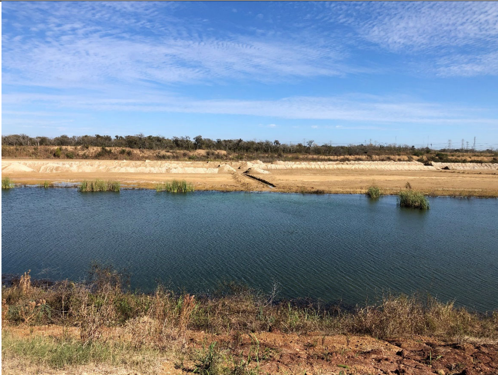
Photograph P-12: View looking northeast from southern berm across storm water pond at waste stored in Cell 2B. Stockpiled fly ash is visible in the center of the photograph, while CCR waste from the Flue Gas Desulfurization system is visible beyond the fly ash.
