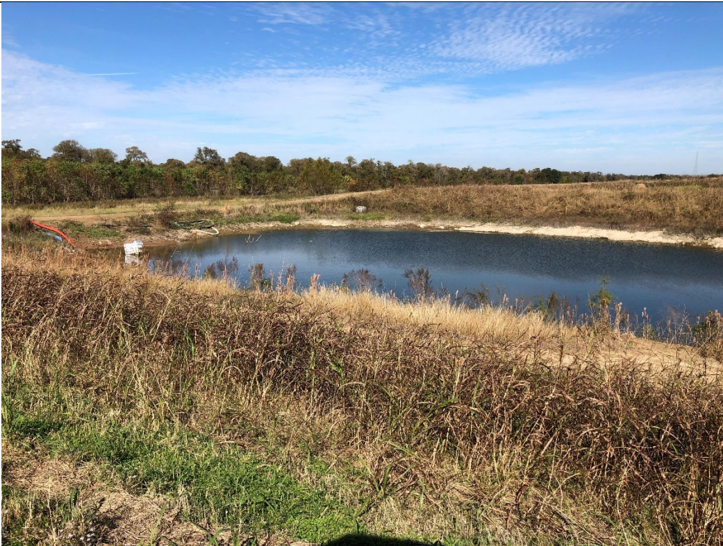
Photograph P-6: View looking north across the contact water pond in Cell 2A. Slopes were either stabilized or well vegetated.
