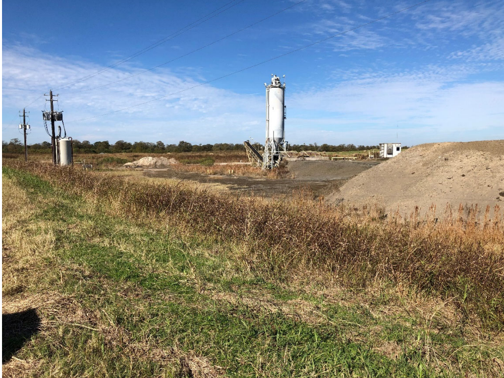
Photograph P-4: View looking west along the south berm of Cell 2A (the Pugmill Area). Stockpiled, salable CCR material is visible on the right side of this photograph.
