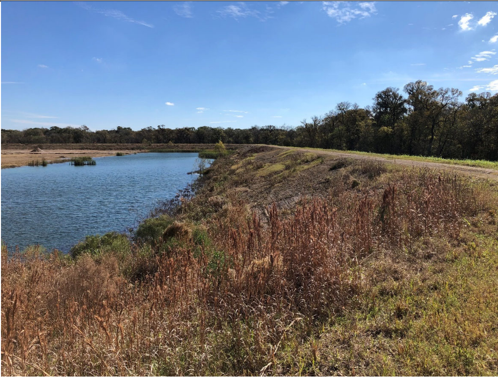
Photograph P-10: View looking southeast of Cell 2B's southern berm from southwest corner of landfill. The Cell 2B stormwater pond is visible to the left.
