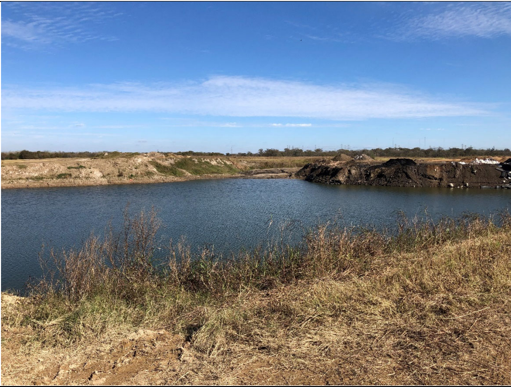
Photograph P-9: View looking northeast of the contact water pond in Cell 1C. Picture was taken from berm at southwest corner of Cell 1C.
