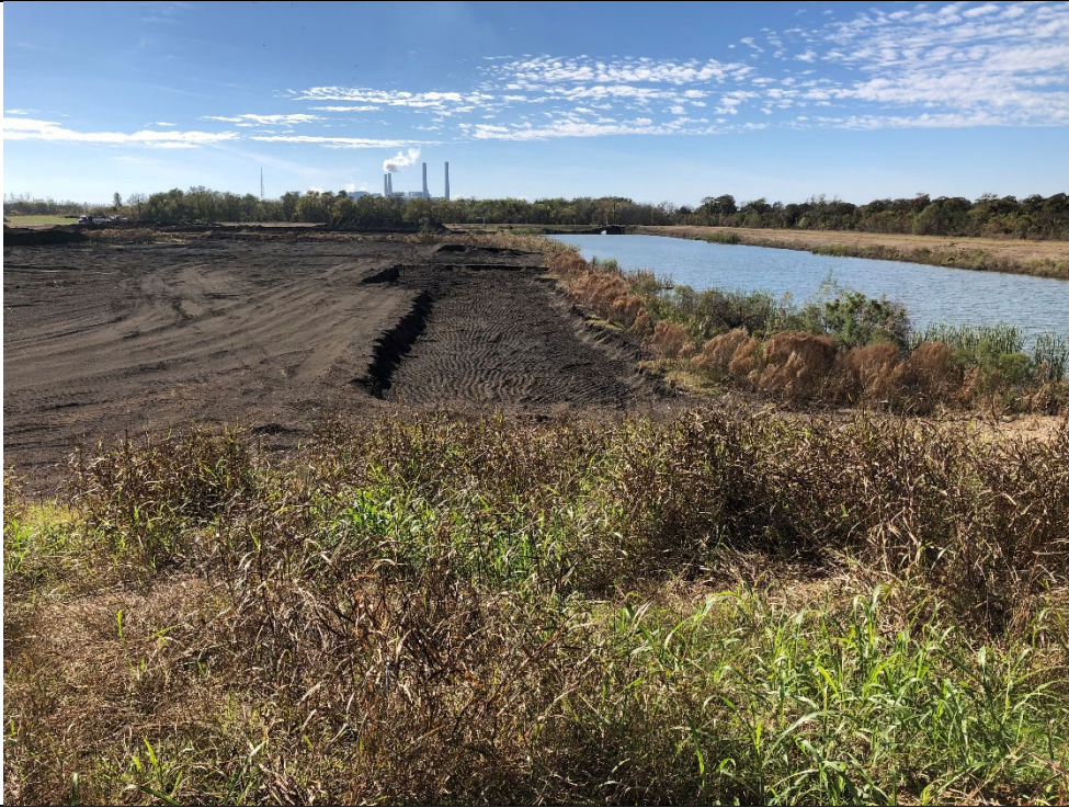
Photograph P-1: View looking south-southwest of Cell 3 from top of north berm. Bottom ash material is visible to the left; the area where bottom ash is being excavated from the landfill is visible in the center of the photograph, and the Cell 3 storm water pond is visible to the right. The interior slopes and crest roads of the berms have been stabilized with a cemented fly ash mixture. The remainder of the berms are well vegetated.
