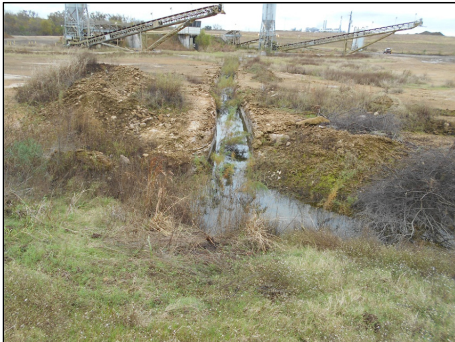
Photograph P-38 – Taken December 1, 2015 by David E. Nielson Landfill Cell 2A: Looking south into the active portion of Cell 2A along a vertical wall ditch cut in the stabilized material that has cured in place. These vertical walls demonstrate the long-term properties of the stabilized CCR materials.
