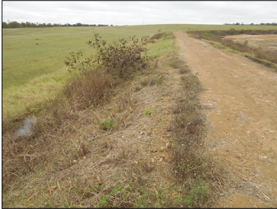
Photograph P-29 – Taken December 1, 2015 by David E. Nielson Landfill Cell 2A: Looking north along the outside slope and crest of the western berm. Note the standing water is from precipitation prior to the inspection not seepage.
