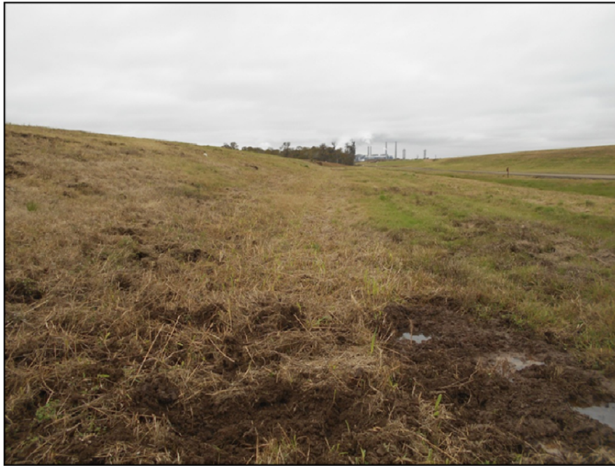
Photograph P-71 – Taken December 1, 2015 by David E. Nielson Landfill Cell 2B: Looking south along toe of western slope with damaged vegetation in foreground. Standing water in some areas is from precipitation not from seepage.
