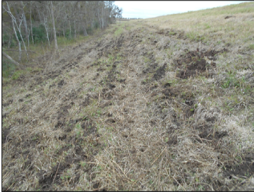
Photograph P-67 – Taken December 1, 2015 by David E. Nielson Landfill Cell 2B: Looking west along outside slope of southern berm/dike. Note significant damage to the vegetation by feral hogs.
