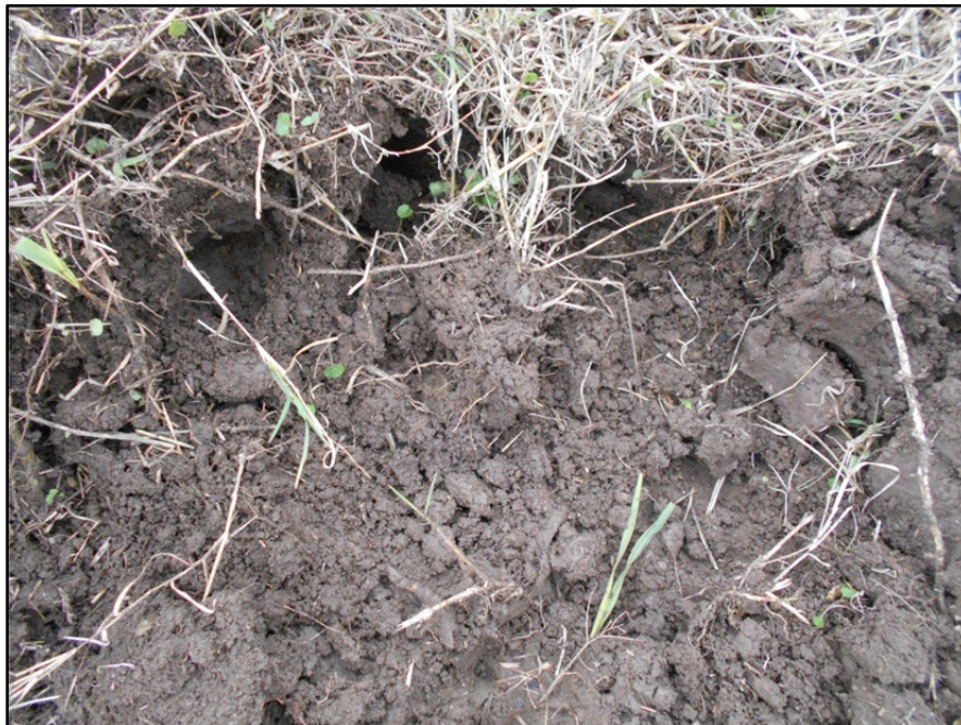
Photograph P-72 – Taken December 1, 2015 by David E. Nielson Landfill Cell 2B: Looking at damage to vegetation shown in Photograph P-71, which was caused by feral hogs. Note shallow depth of disturbance and likelihood of re-vegetation due to intact grass roots.
