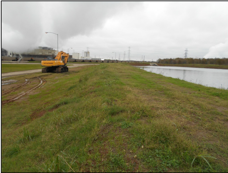
Photograph P-7 – Taken December 1, 2015 by David E. Nielson Air Preheater Pond: Looking northwest along exterior slope and crest of western dike. Note minor vegetation deficiencies as the recent seeding of grass becomes established. The grass vegetation has become well established since Photograph P-6 was taken.
