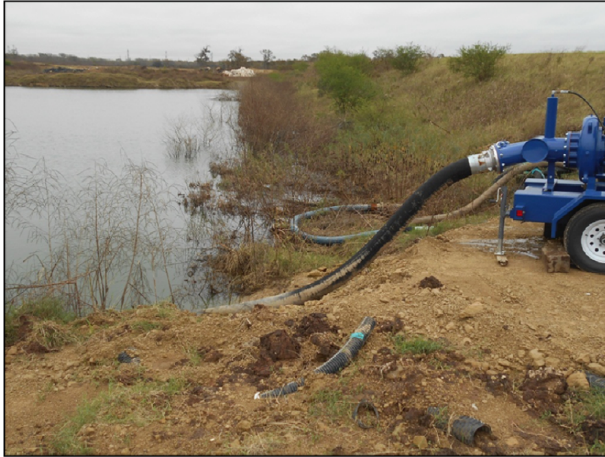
Photograph P-46 – Taken December 1, 2015 by David E. Nielson Landfill Cell 1C: Looking east along the inside slope of the southern dike of the stormwater pond. Note vegetation control is warranted.
