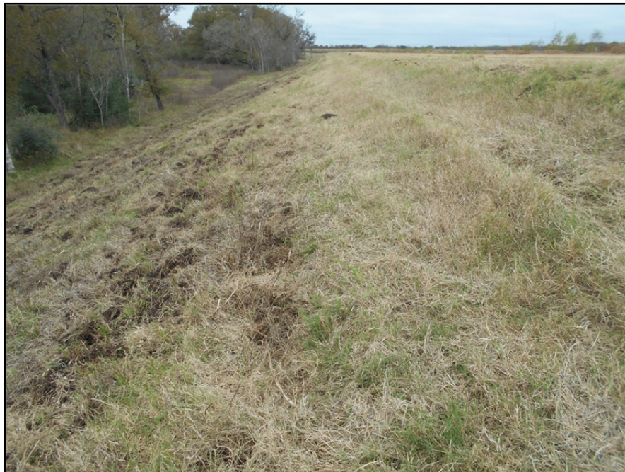
Photograph P-66 – Taken December 1, 2015 by David E. Nielson Landfill Cell 2B: Looking west along outside slope of southern berm/dike. Note ongoing feral hog damage to vegetation.
