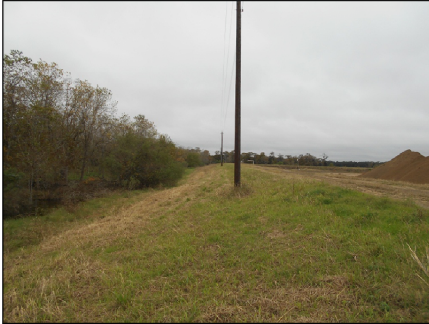
Photograph P-11 – Taken December 1, 2015 by David E. Nielson Landfill Cell 3: Looking west along the outside slope of the south slope of landfill berm. Note good vegetation.
