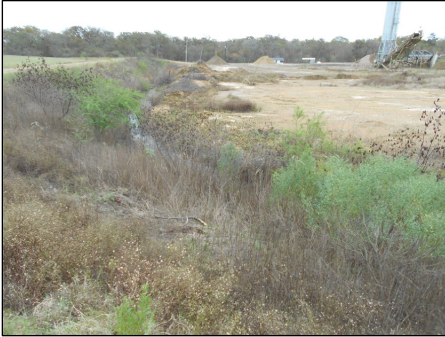
Photograph P-35 – Taken December 1, 2015 by David E. Nielson Landfill Cell 2A: Looking east along the inside slope of northern berm. Note small trees that should be removed.
