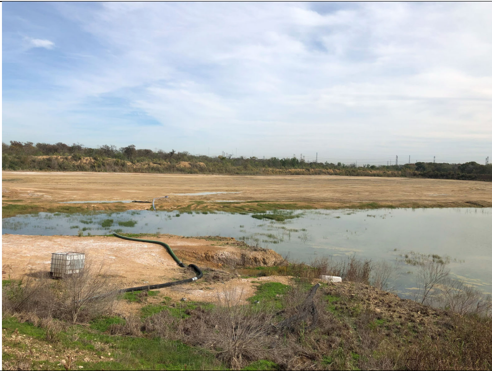
Photograph P-11: View looking northeast Cell 2B. The Cell 2B stormwater pond is visible in the foreground, the fly ash storage and loading area is visible in the middle background, and the Flue Gas Desulfurization (FGD) waste is visible in the far background.
