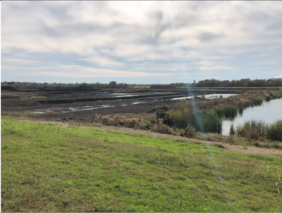
Photograph P-1: View looking southeast of Cell 3 from top of north berm. The darker bottom ash material is visible in this photograph, as is the area where the bottom ash is being excavated from the landfill and sold as road base. The Cell 3 storm water pond is visible to the right. The interior slopes and crest roads of the berms are either vegetated (slopes) or have been stabilized with a cemented fly ash mixture.
