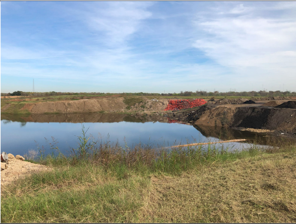
Photograph P-7: View looking north across the contact water pond in Cell 1C. This view is towards the area that was recently closed (located just to the north of the pond and left background of this photograph).
