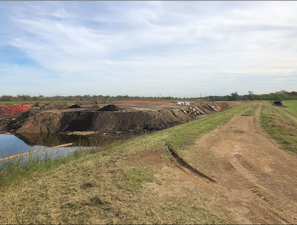
Photograph P-8: View looking northeast from the berm at the southwest corner of Cell 1C. The Cell 1C storm water pond is visible on the left side of this photograph, while waste piles are visible in the background.
