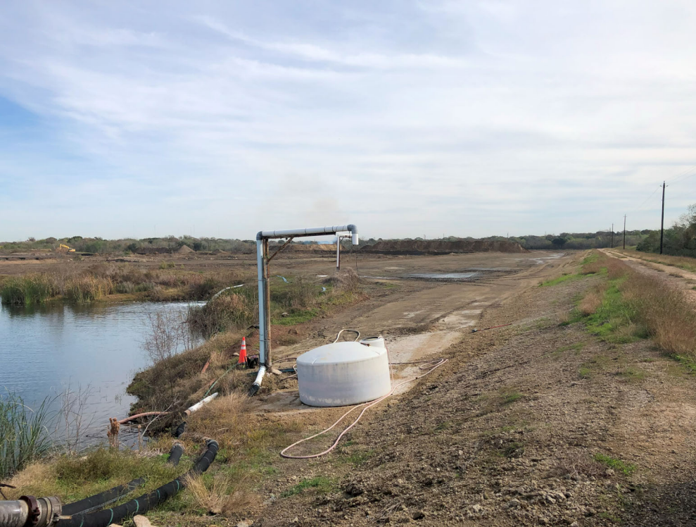
Photograph P-2: View looking east from Cell 3's southwest interior corner. The crest road was well maintained, exterior slopes well vegetated without erosion issues, and interior slope either improved with stabilized CCR material or vegetated.
