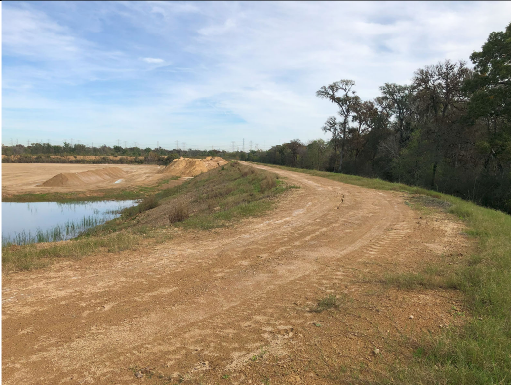
Photograph P-14: View looking northwest from the southeast corner of Cell 2B. The crest road is visible to the right, FGD system waste is visible to the left.
