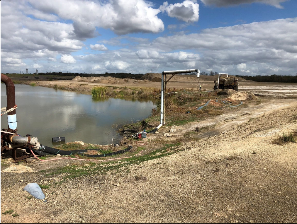
Photograph P-3: View looking northeast of Cell 3 Coal Combustion Residual (CCR) waste pile and of location where water from Cell 3's contact water pond is transferred to trucks.
