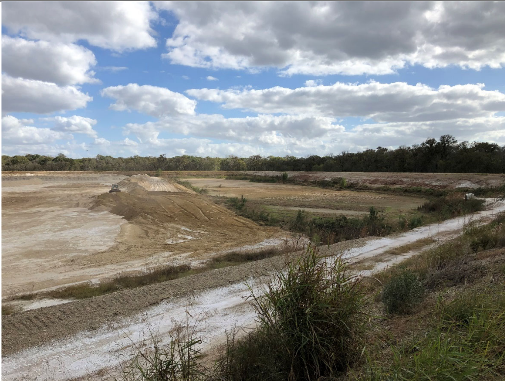
Photograph P-10: View looking east over an entry road of Cell 2B from western berm. This photograph shows the fly ash storage area on the left and center of the photograph. The dry contact water pond is visible on the right side of the photograph.
