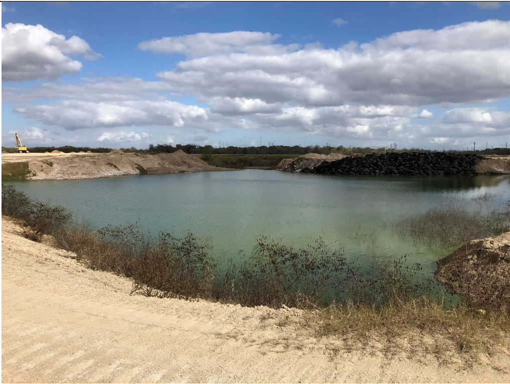
Photograph P-9: View looking northeast of the contact water pond in Cell 1C. Picture was taken from berm at southwest corner of Cell 1C.
