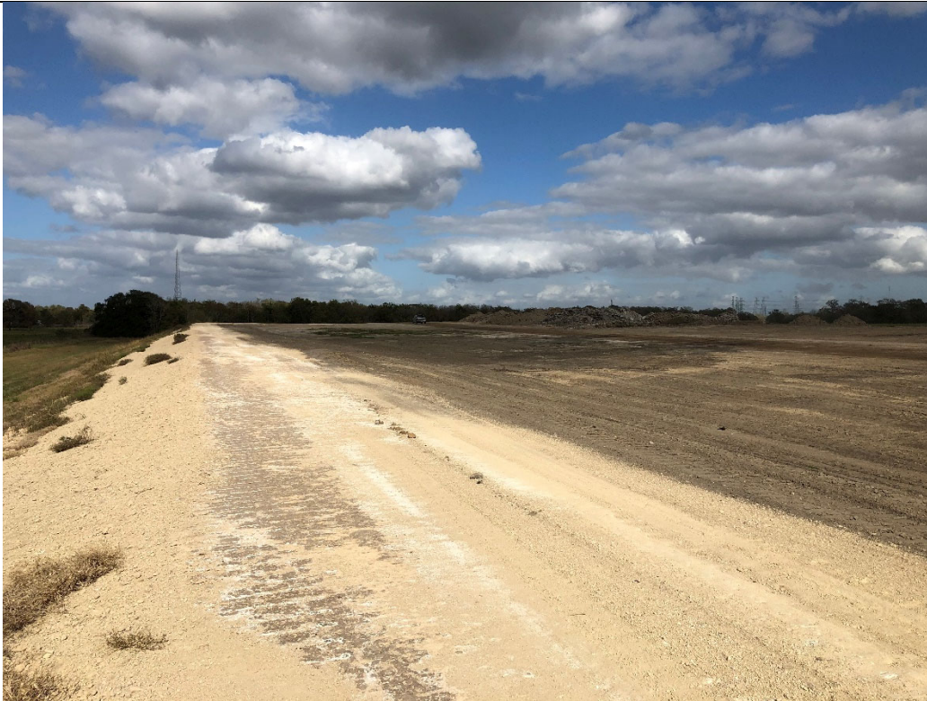
Photograph P-8: View looking north of the western berm of Cell 1C. This portion of the landfill is full – CCR waste material is visible to the right of the berm road.
