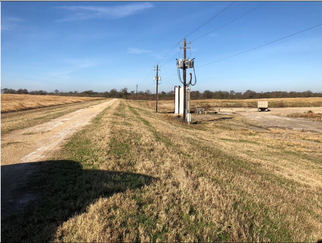
Photograph P-5: View looking north along the west berm of Cell 2A (the Pugmill Area).
