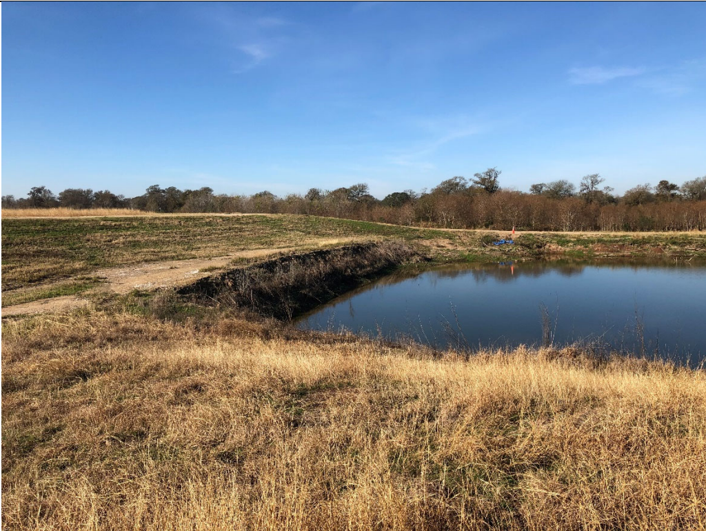
Photograph P-6: View looking west across the contact water pond in Cell 2A. Slopes were either stabilized or well vegetated.
