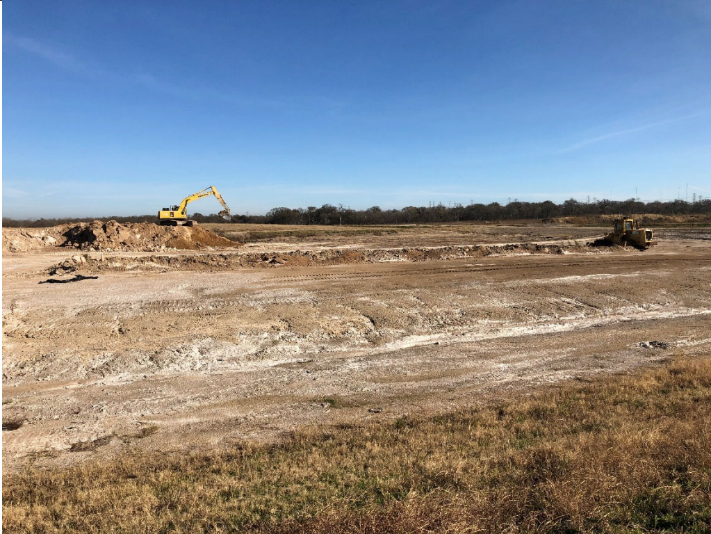
Photograph P-8: View looking north of waste CCR material in Cell 1C. Picture was taken from southern berm of Cell 1C.
