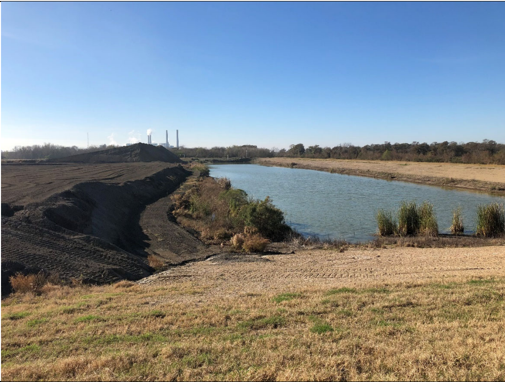
Photograph P-1: View looking south of Cell 3 from top of north berm. Bottom ash material is visible to the left; the Cell 3 contact water pond to the right. The interior slopes and crest roads of the berms have been stabilized with a cemented mixture of bottom ash and fly ash. The remainder of the berms are well vegetated.
