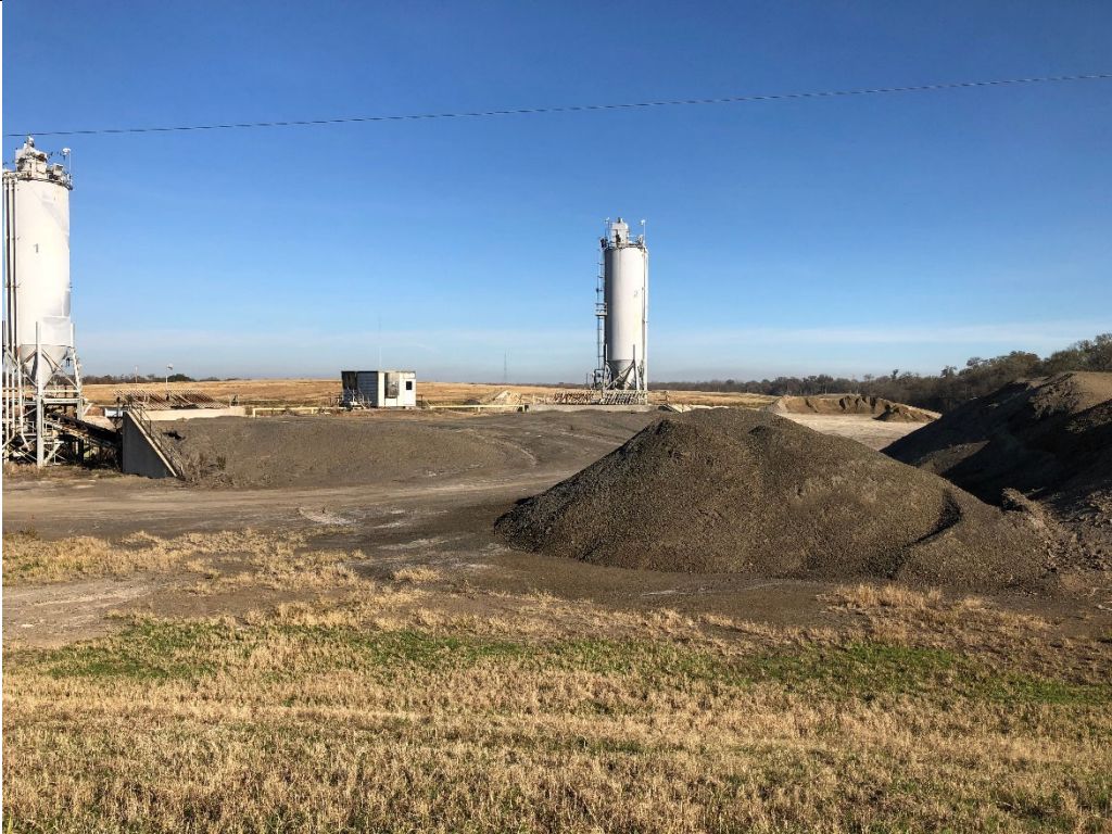
Photograph P-4: View looking north of Cell 2A, the Pugmill Area. Pugmill equipment and mixed CCR material are visible in this photograph.
