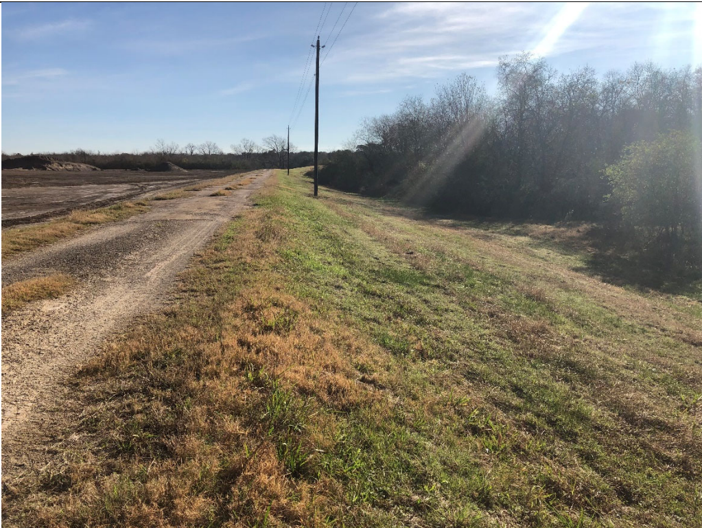
Photograph P-2: View looking east of Cell 3's south berm. The crest road was well maintained, exterior slopes well vegetated without erosion issues.
