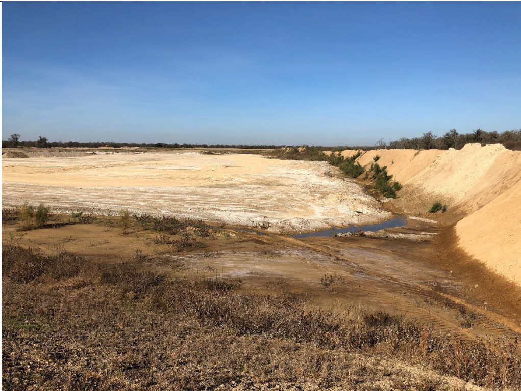
Photograph P-10: View looking west of Cell 2B from eastern berm. This photograph shows the fly ash storage area on the left, dried and stabilized Flue Gas Desulfurization (FGD) CCR waste material on the right, and a contact water ditch separating the two.
