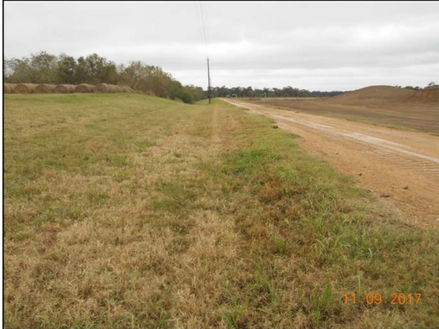
Photograph P-2 – Taken November 9, 2017 by David E. Nielson Landfill Cell 3: Looking west along the crest and outside slope of the south landfill berm. Note the well-established vegetation.
