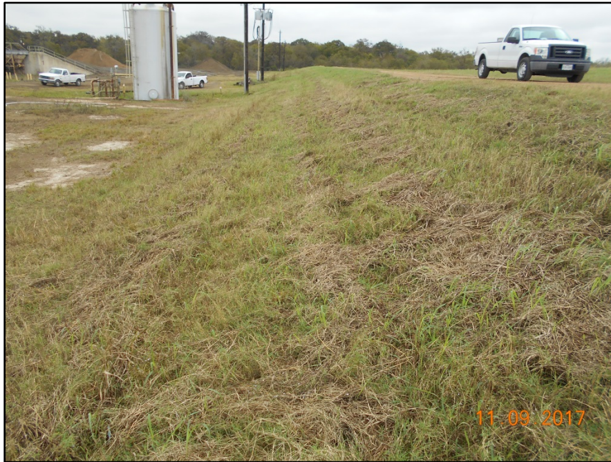
Photograph P-13 – Taken November 9, 2017 by David E. Nielson Landfill Cell 2A: Looking east along the inside slope of the southern berm. This berm abuts closed Cell 1B, which is higher in elevation. Note well established grass and uniformity of slope.
