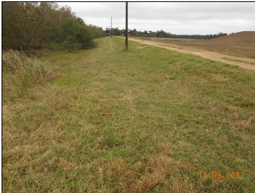
Photograph P-3 – Taken November 9, 2017 by David E. Nielson Landfill Cell 3: Looking west along the crest and outside slope of the south landfill berm Note the good vegetation.
