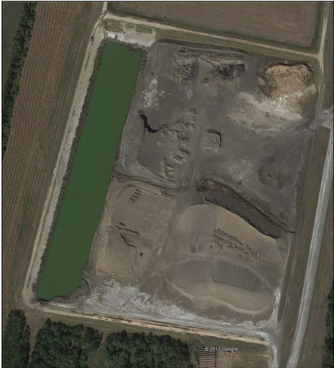
Photograph P-1 – From Google Earth Pro, dated October 28, 2017. Downloaded December 26, 2017. Landfill Cell 3: Aerial view of landfill cell and storm water runoff pond inside western edge of cell.
