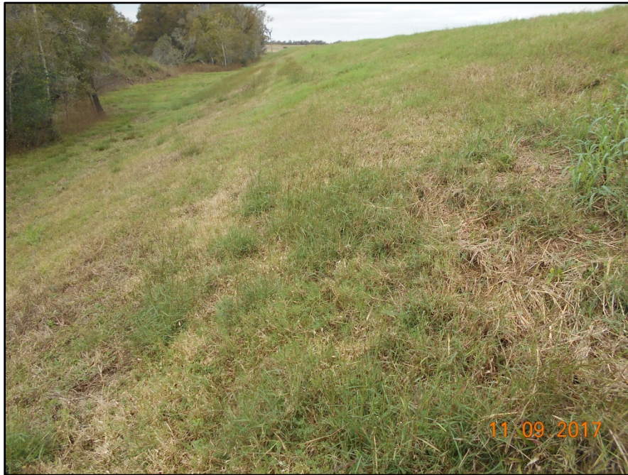
Photograph P-47 – Taken November 9, 2017 by David E. Nielson Landfill Cell 2B: Looking west along the outside slope of the southern landfill berm. Note good vegetation.
