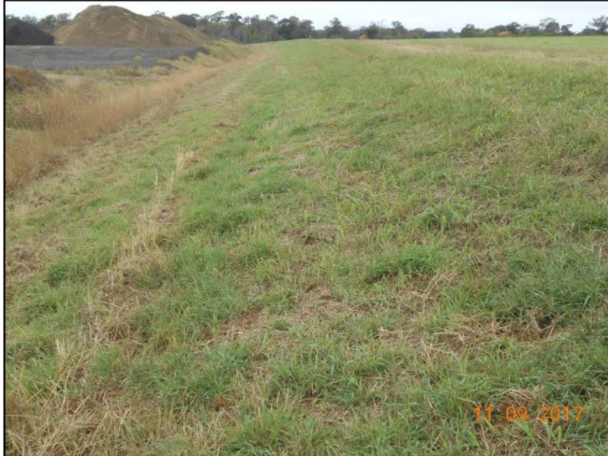
Photograph P-10 – Taken November 9, 2017 by David E. Nielson Landfill Cell 3: Looking west along inside slope of northern berm of the landfill. Note the good vegetation.
