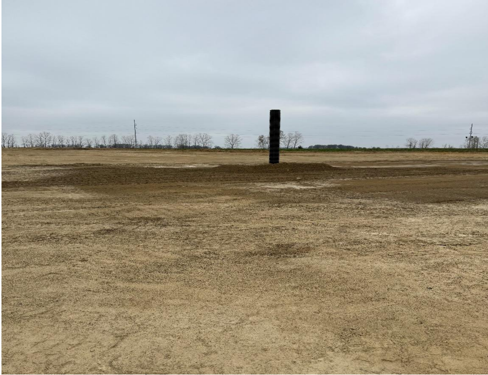
Photo 3. Active working face, bottom ash with chimney drain looking West (Cell 2).
