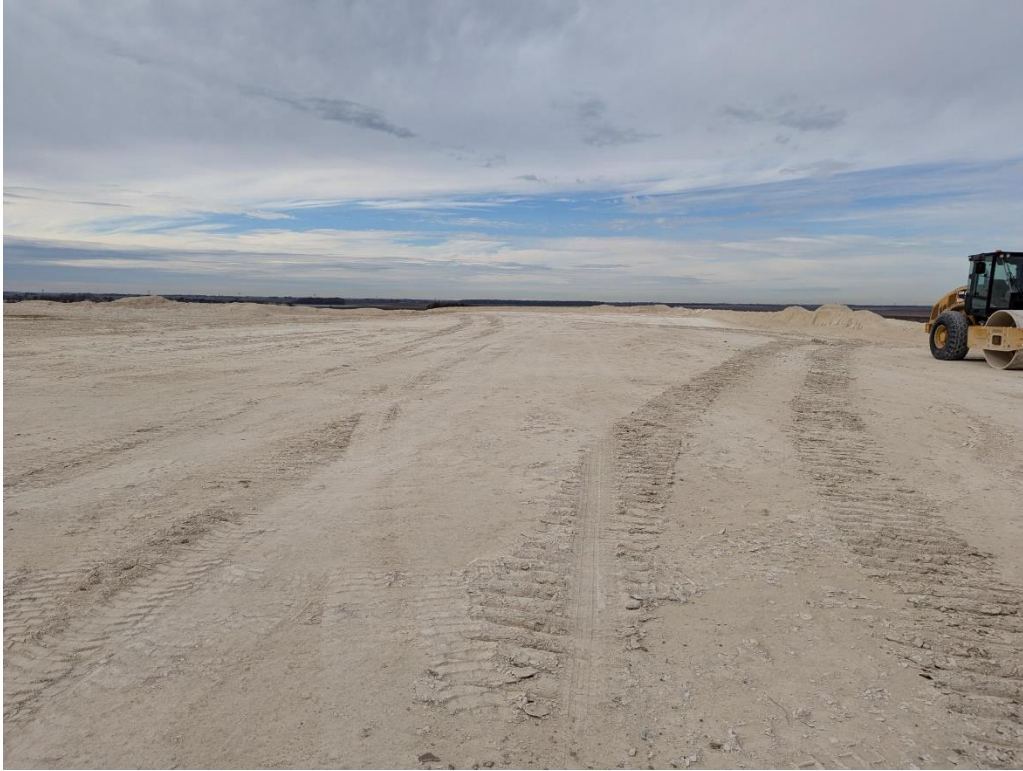
Photo 5. Open disposal area, Cells 1 and 3.
