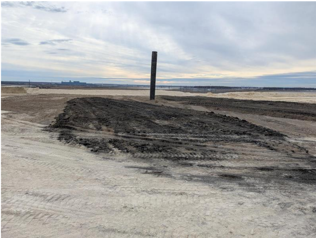
Photo 4. Active working face, bottom ash with chimney drain looking South (Cell 3).
