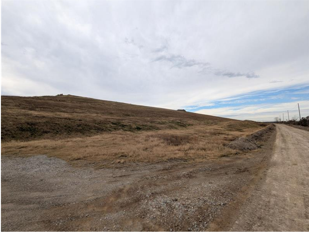
Photo 7. Typical perimeter side slope intermediate cover and vegetation.
