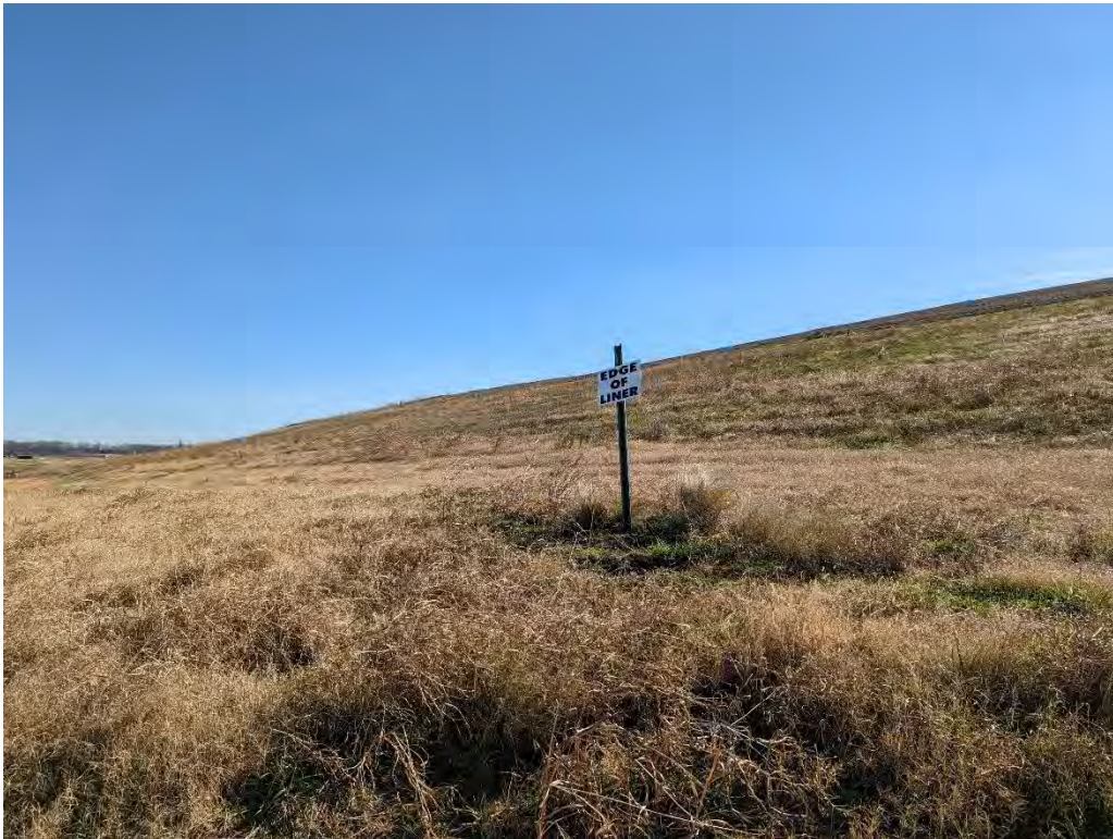
Photo 10. Side slope interim cover with edge of liner sign in foreground
