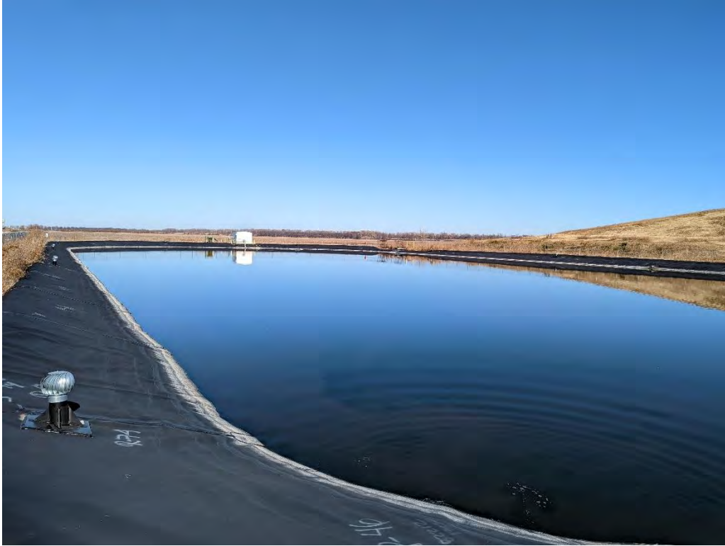
Photo 9. Leachate Pond from southwest
