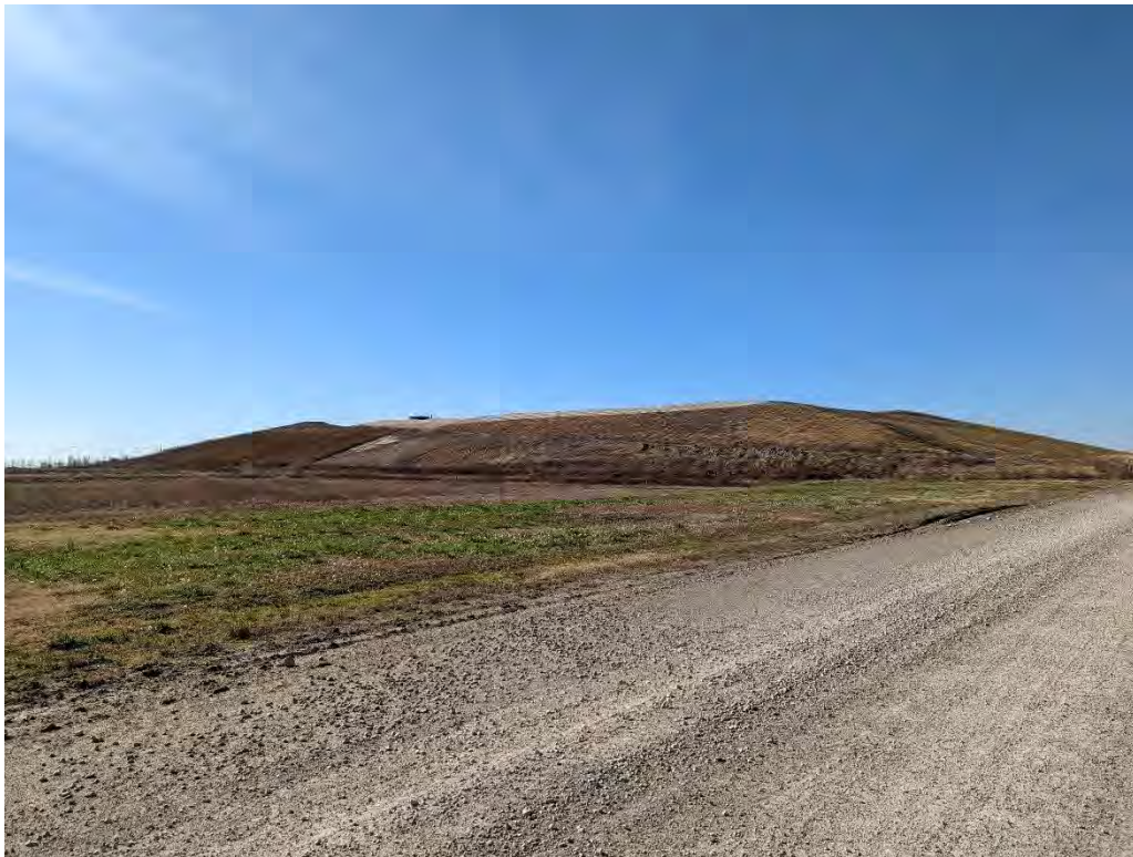
Photo 4. Haul road to landfill from East.
