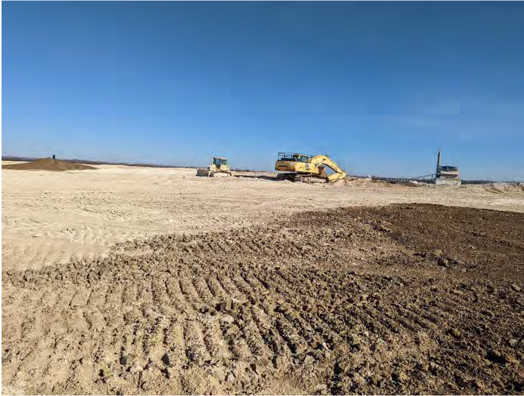
Photo 1. Active working area (Cell 3)
