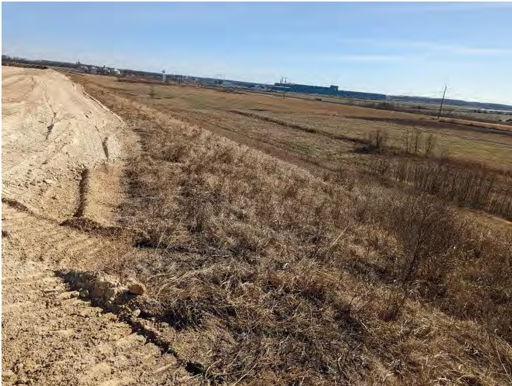
Photo 6. Cell 3 south slope interim cover.
