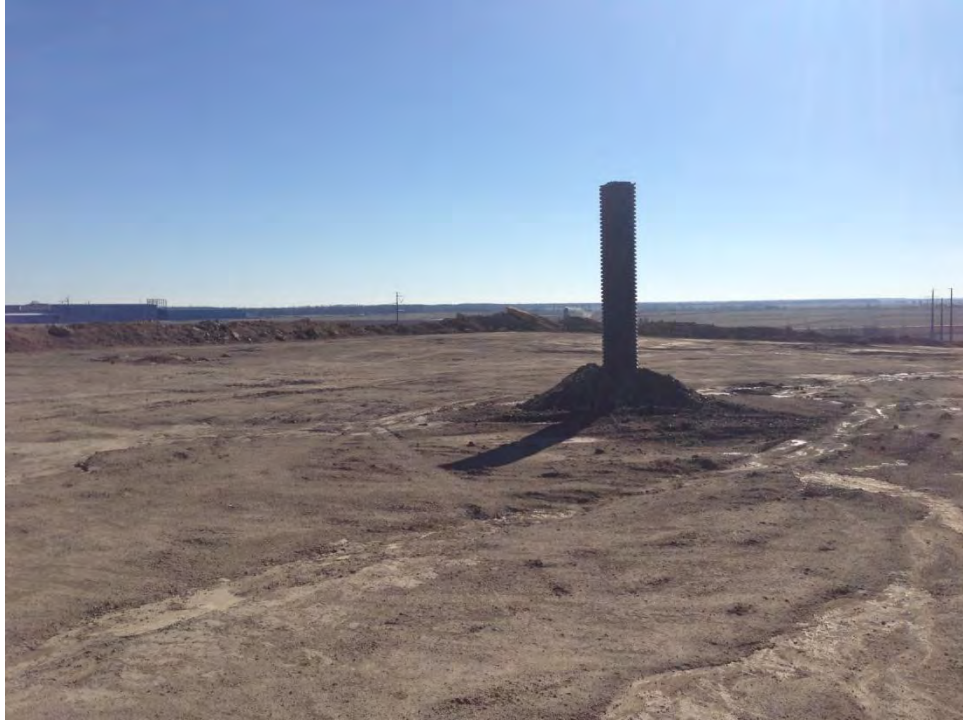
Photo 8: Top of Cell 1, edge berms and chimney drain
