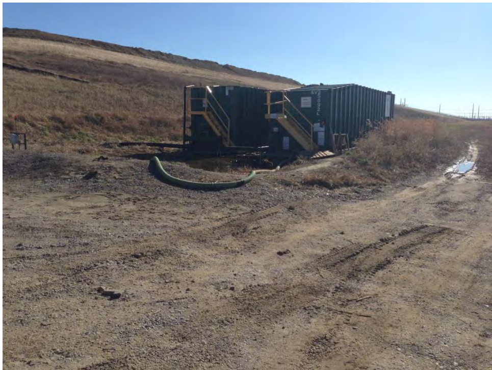
Photo 4: Leachate storage tanks
