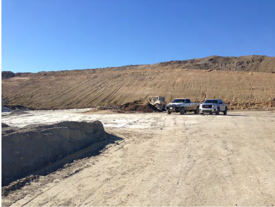
Photo 1: Cell 3 disposal area, Cell 1 from east
