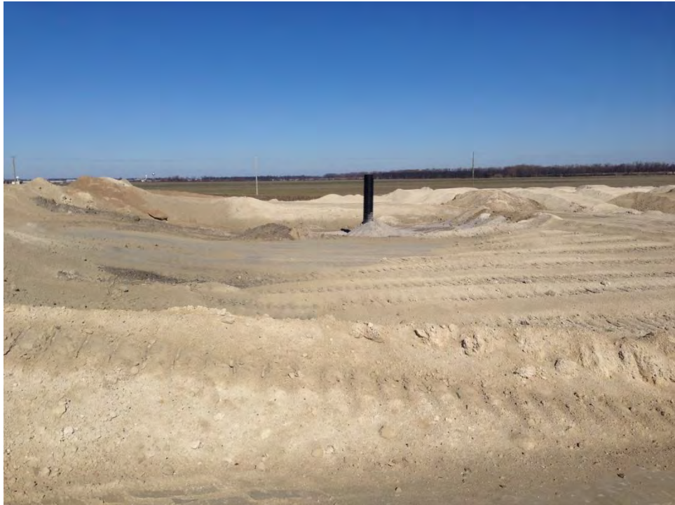
Photo 9: Cell 3 northwest chimney drain
