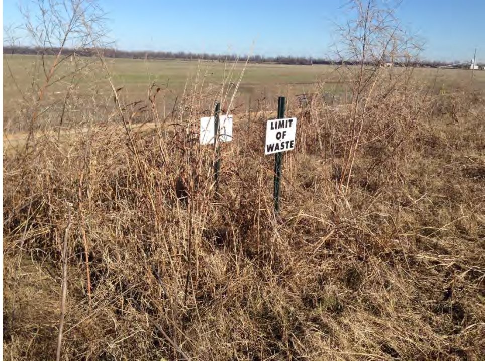
Photo 3: Typical 'Limit of Waste' and 'Edge of Liner' signage
