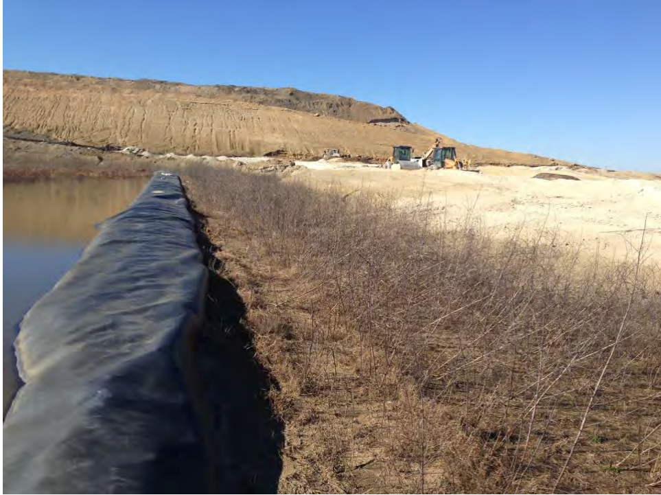
Photo 10: Cell 3 stormwater separation berm, from east
