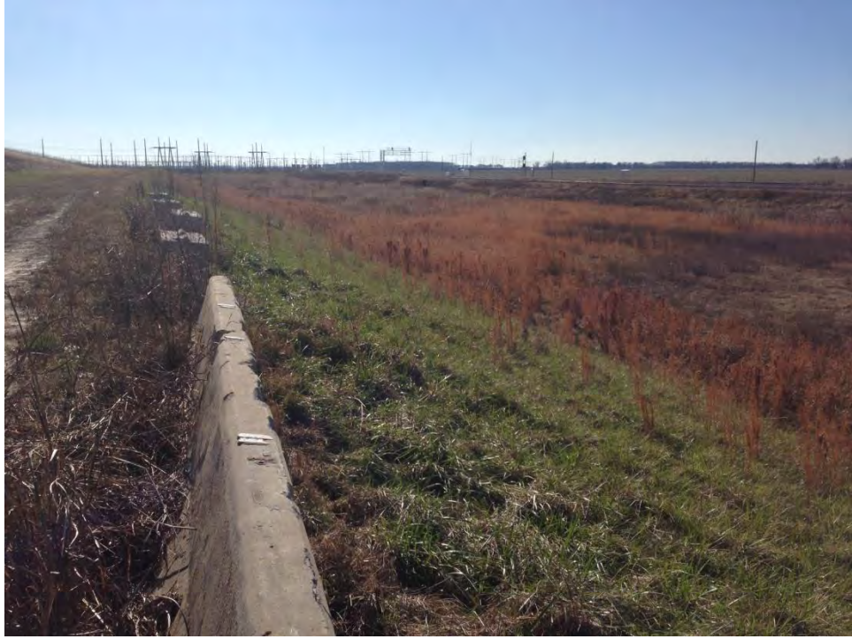
Photo 5: Stormwater pond from Northeast
