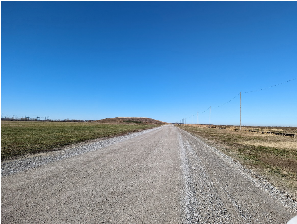
Photo 2. Haul road to landfill looking West.
