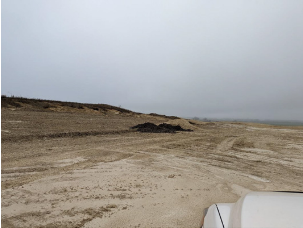
Photo 5. Working face looking northwest at Cell 1 top elevation.
