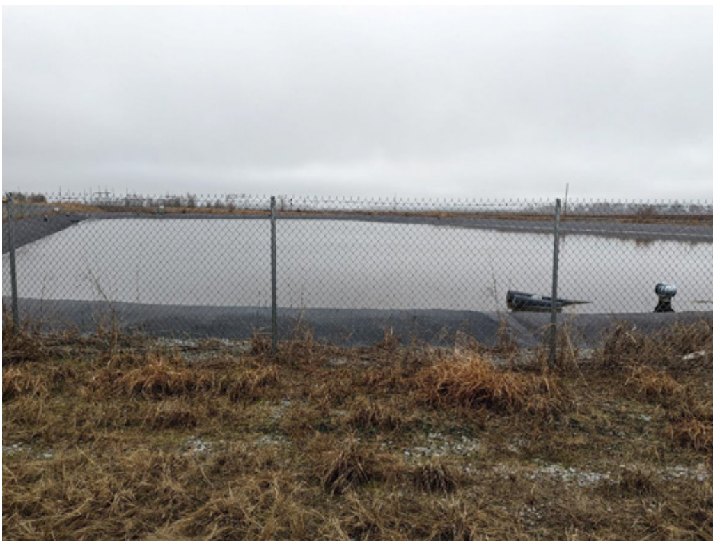
Photo 9. Leachate pond from north.
