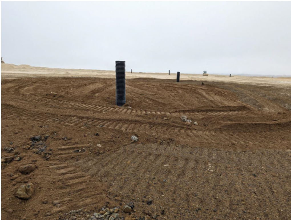
Photo 4. Active disposal area, bottom ash with chimney drains (Cell 3).
