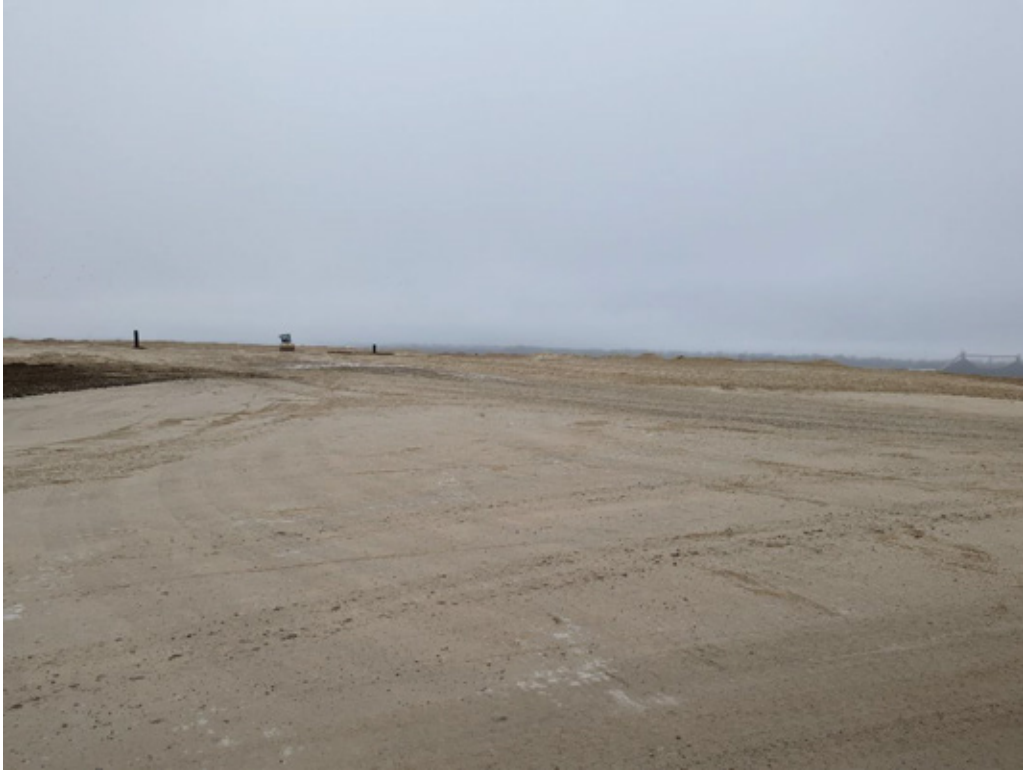
Photo 3. Active disposal area, fly ash (Cell 3).
