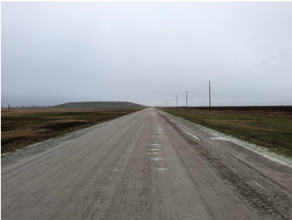
Photo 2. Haul road to landfill from east.
