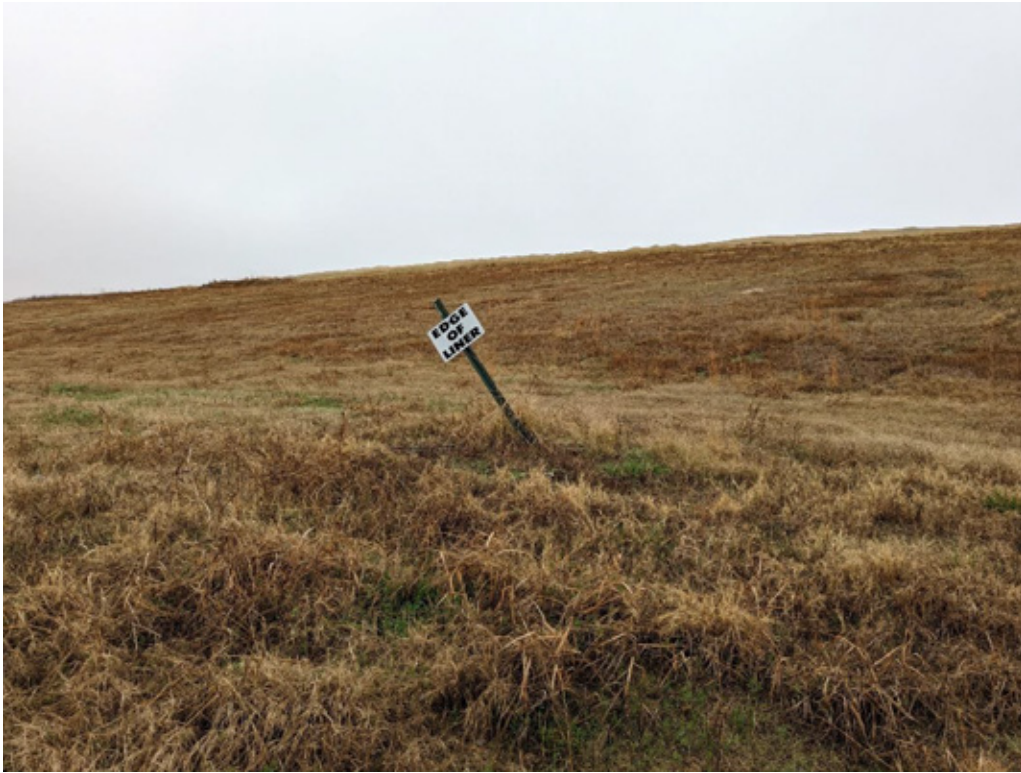
Photo 7. North slope intermediate cover with “Edge of Liner” sign.
