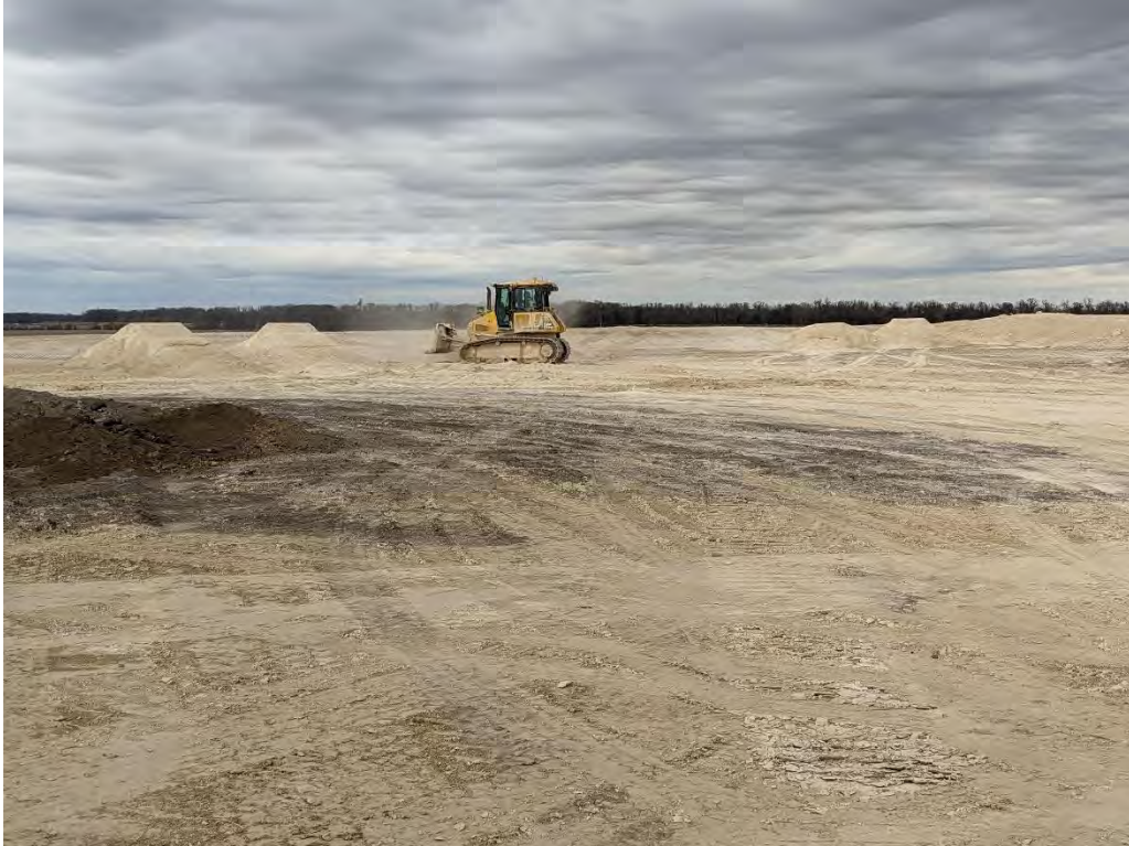
Photo 2. Active working face (Cell 3)
