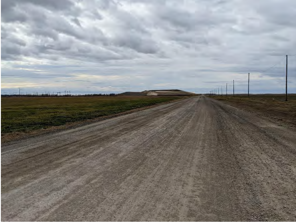
Photo 3. Haul road looking towards Landfill
