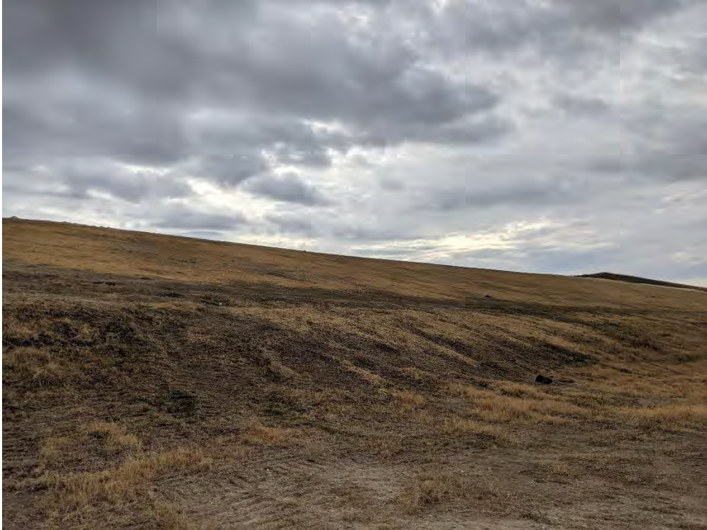
Photo 6. North slope Cell 3 with intermediate cover, seeding and mulch
