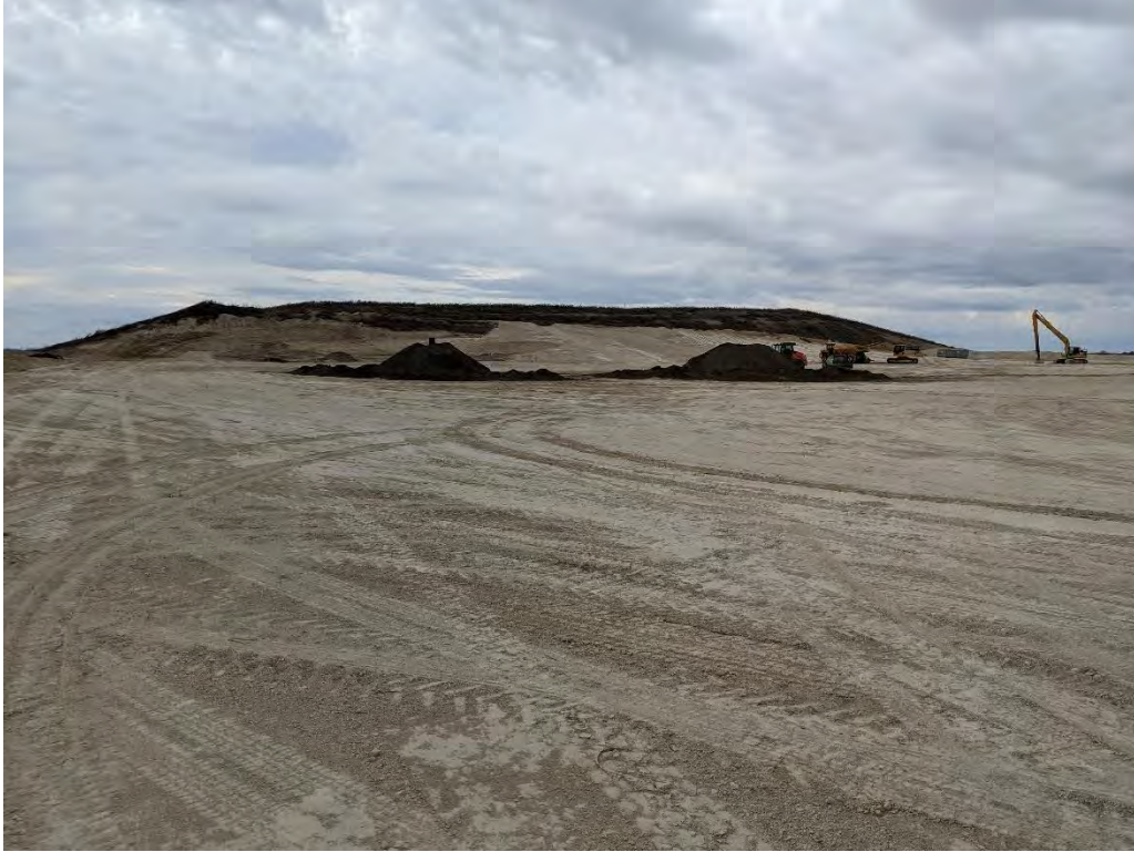
Photo 1. Rolled and sealed top of open disposal cell (Cell 3)
