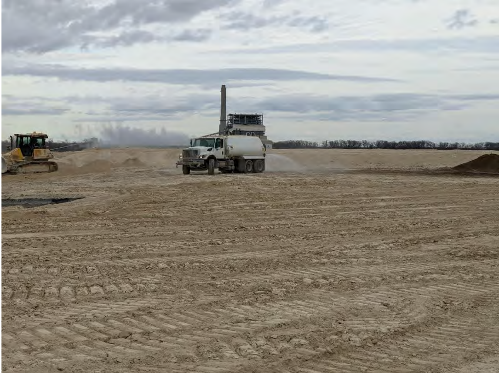
Photo 4. Water truck activities in active disposal area
