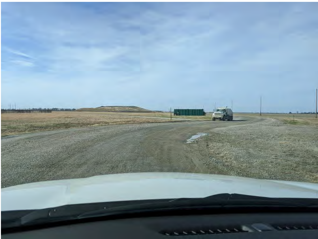
Photo 4. Water truck preparing to wet haul road
