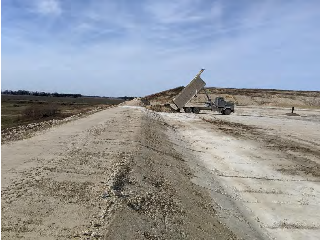
Photo 2. Active working face (Cell 3).
