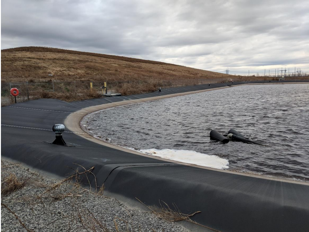
Photo 6. West slope Cell 1 under interim cover with leachate pond in foreground
