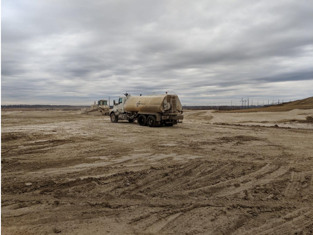
Photo 4. Water truck preparing to wet Cell 3
