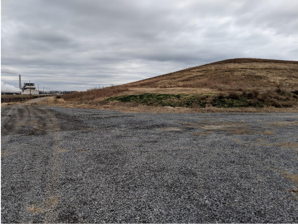
Photo 7. Cell 1 from northwest.
