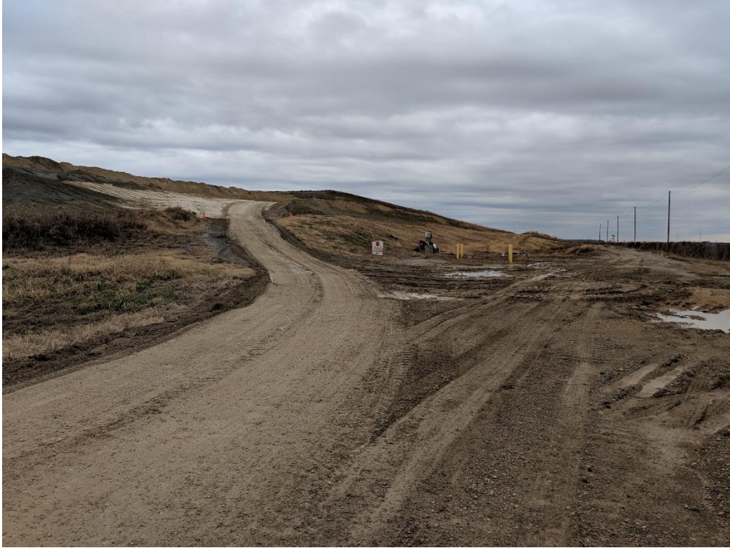
Photo 3. Haul road looking towards Cell 3
