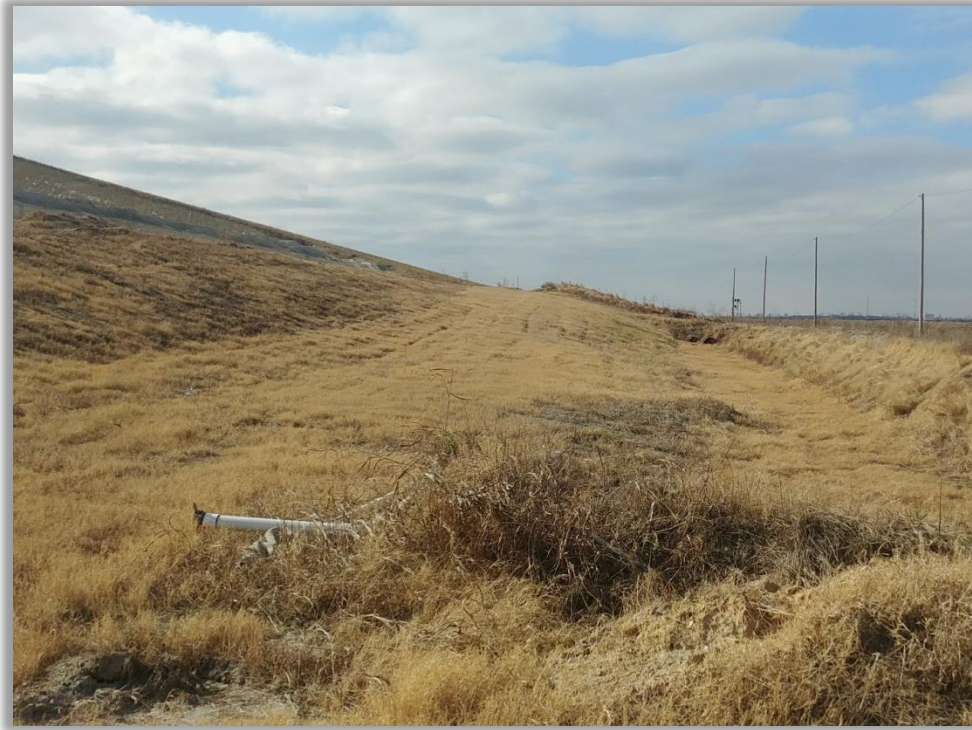
Photo 11: North slope of Cell 1 and perimeter stormwater channel.
