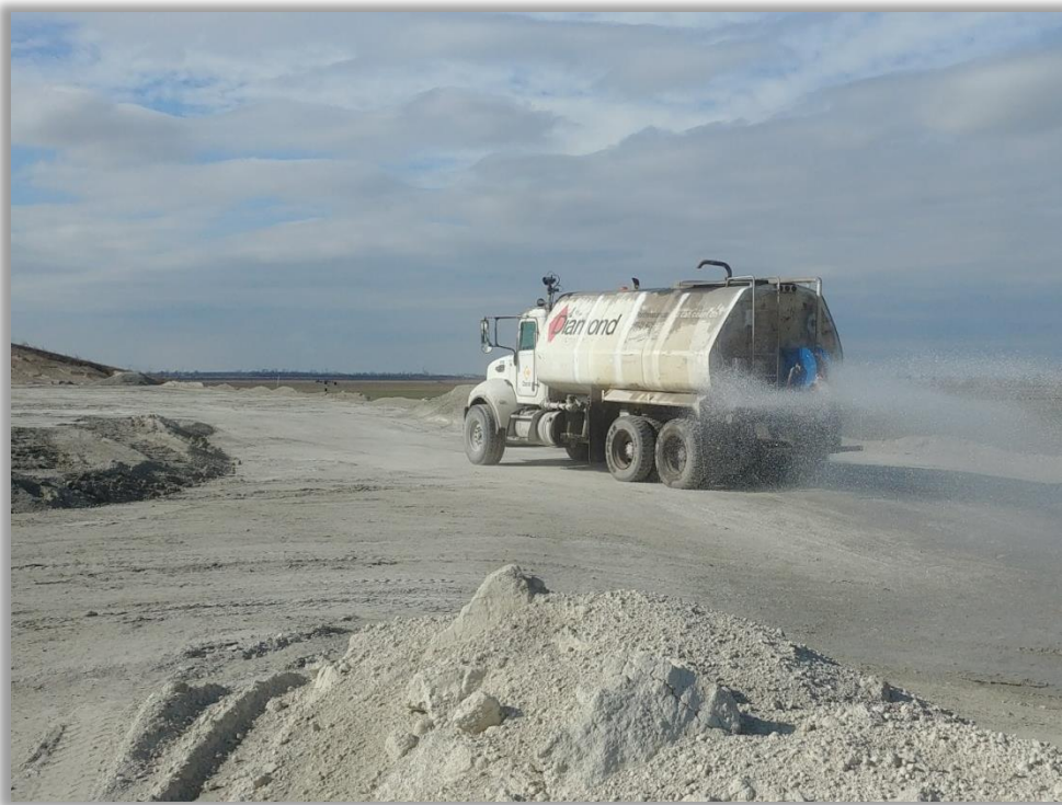
Photo 4: Water truck applying water for dust suppression.
