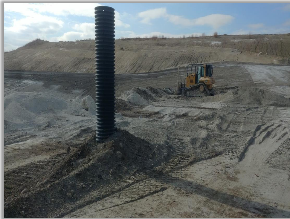
Photo 6: Typical Cell 3 chimney drains.
