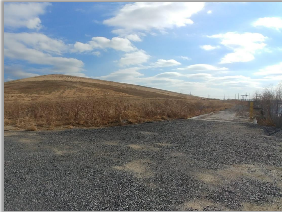
Photo 13: Northwest corner of cell 1 and leachate truck loading station.
