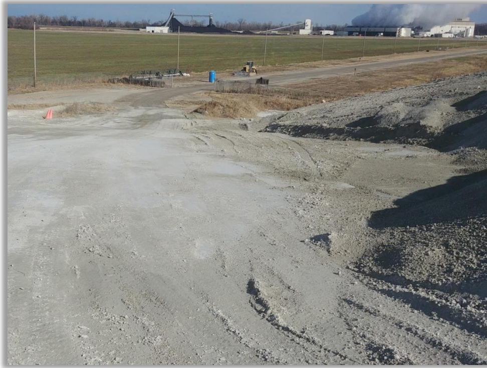
Photo 7: Haul road from top of cell 3.
