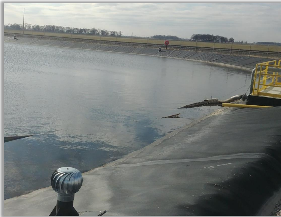
Photo 10: Leachate storage pond from north.
