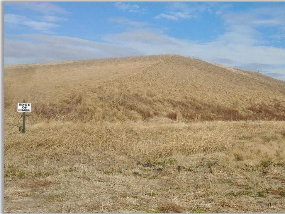
Photo 9: Cell 1 from northwest and typical 'Edge of Liner' signage.
