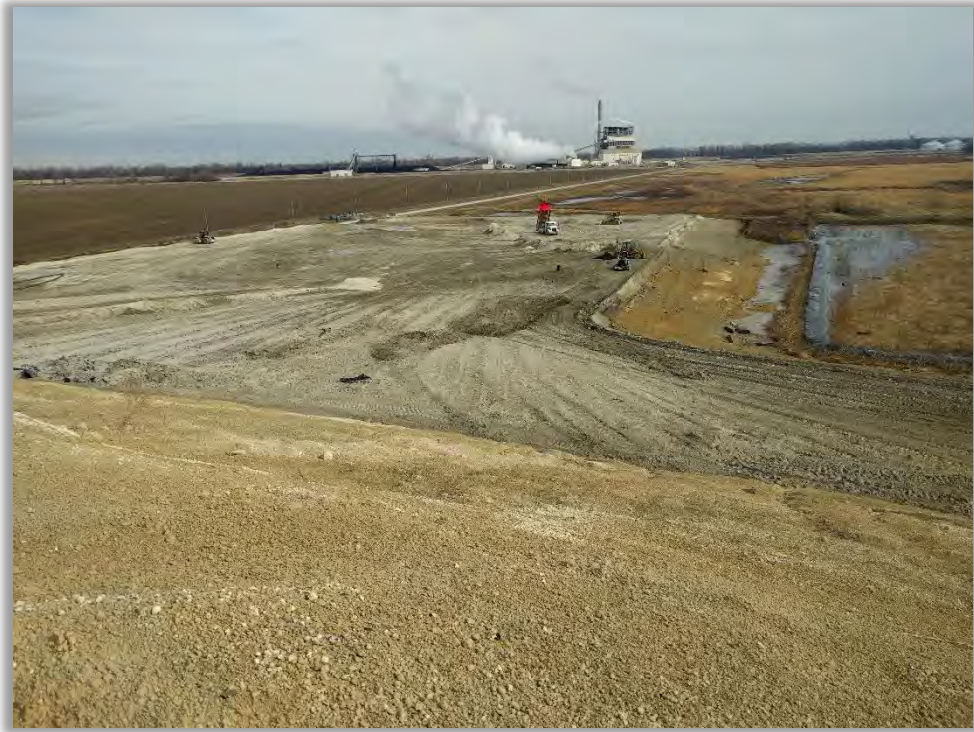
Photo 5: Active disposal area, Cell 3, from west.
