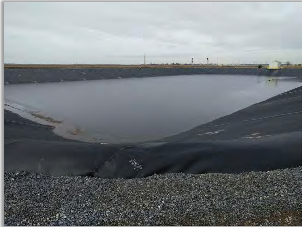
Photo 11: New leachate storage pond from southeast.
