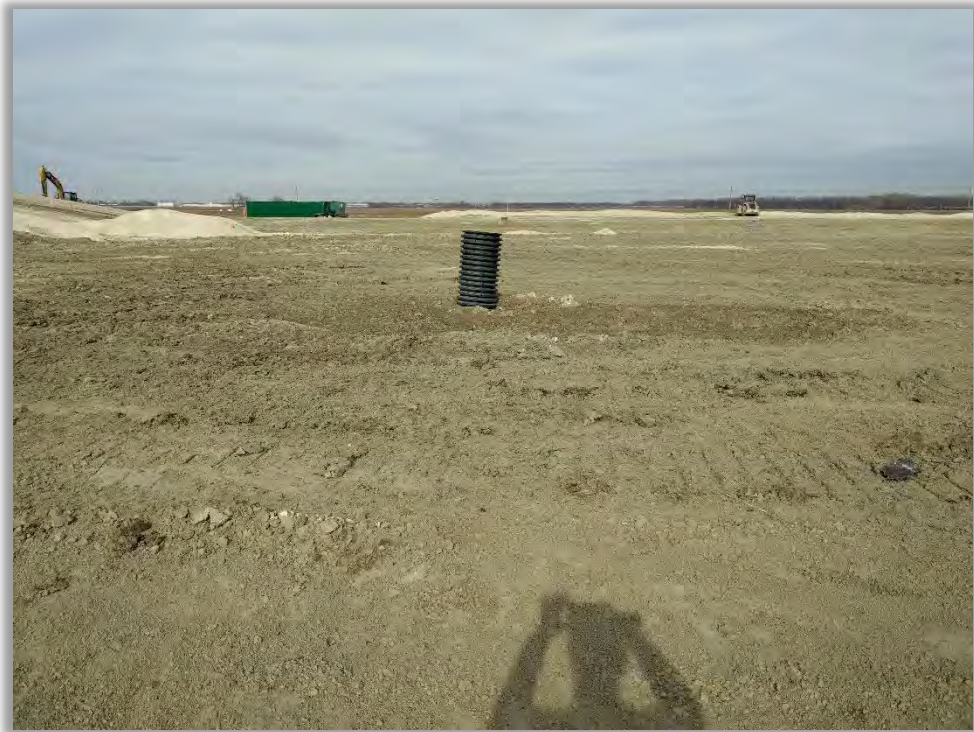
Photo 6: Typical Cell 3 chimney drains.
