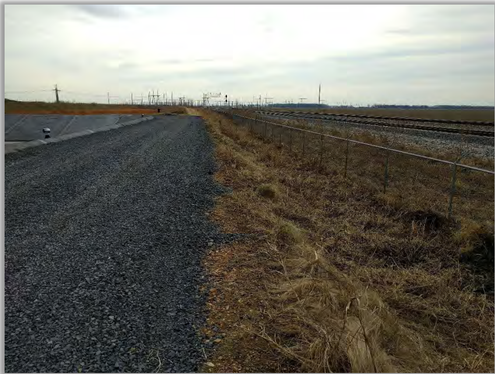
Photo 16: West perimeter stormwater ditch.
