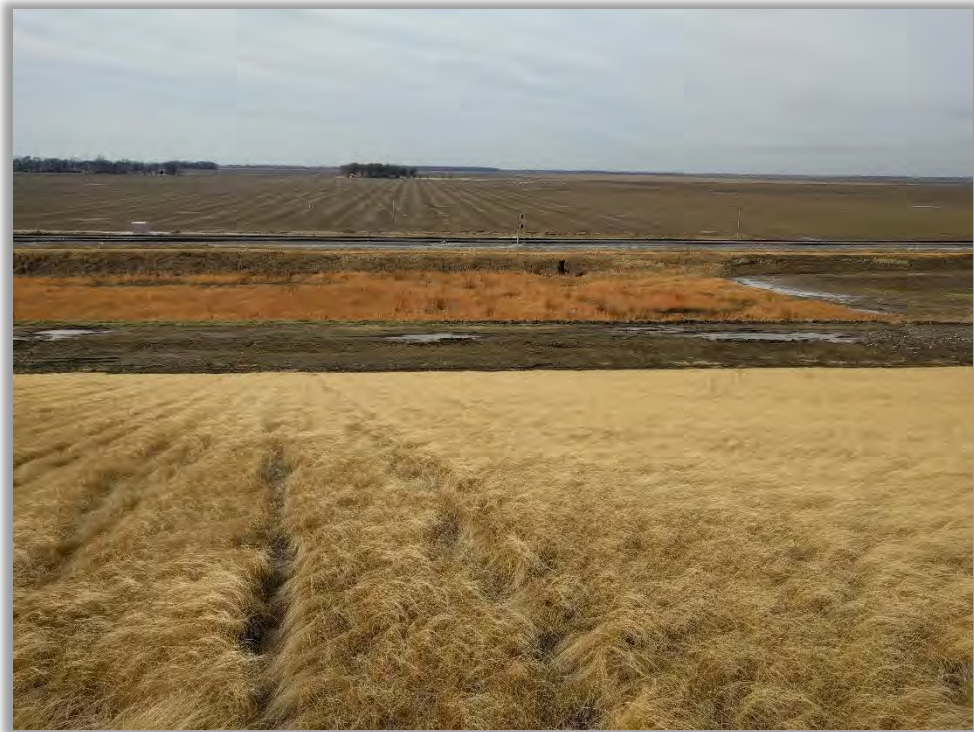
Photo 12: West slope of Cell 1 and stormwater pond looking west.
