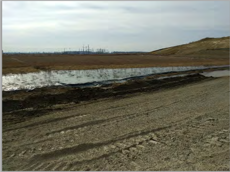
Photo 7: Cell 3 stormwater separation berm, from northeast.
