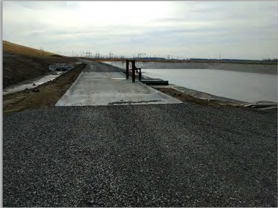
Photo 15: New leachate truck loading station and spill pad.
