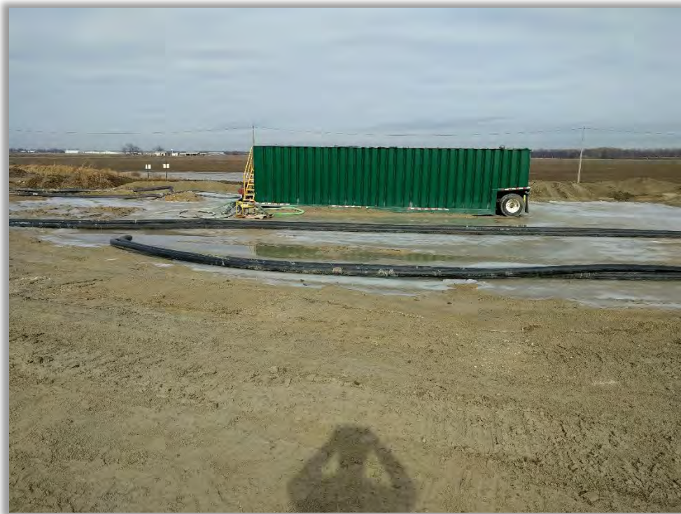
Photo 10: Leachate storage tanks, relocated to within Cell 3.
