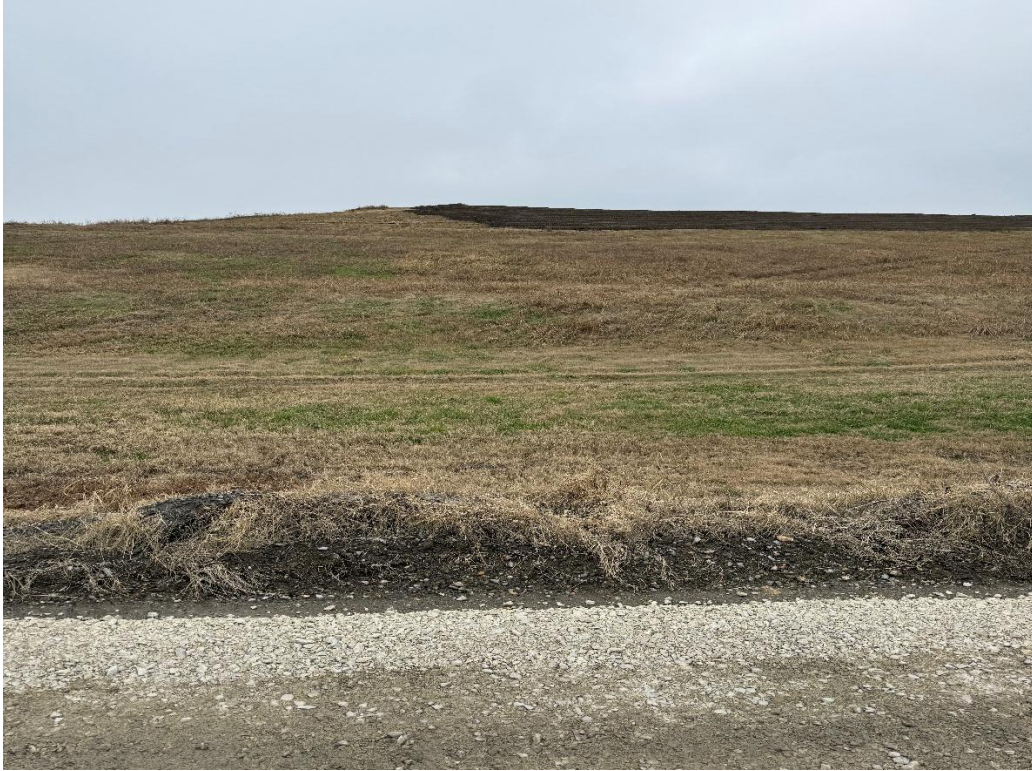
Photo 5. Typical perimeter side slope intermediate cover and vegetation.
