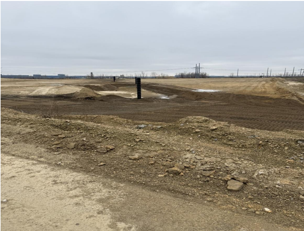
Photo 4. Open disposal area, Cell 2.
