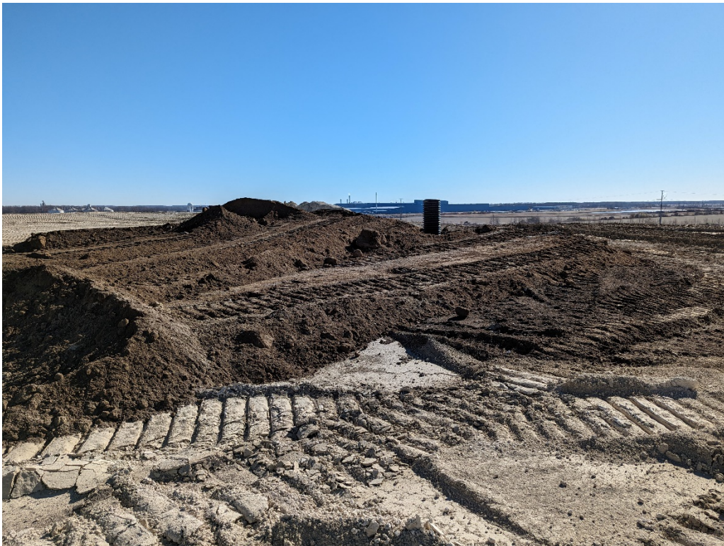
Photo 4. Active working face, bottom ash with chimney drains looking Southeast (Cell 3).
