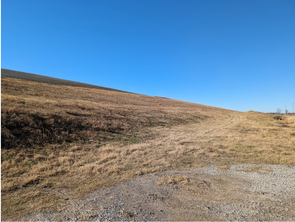
Photo 7. Typical side slope intermediate cover and vegetation.
