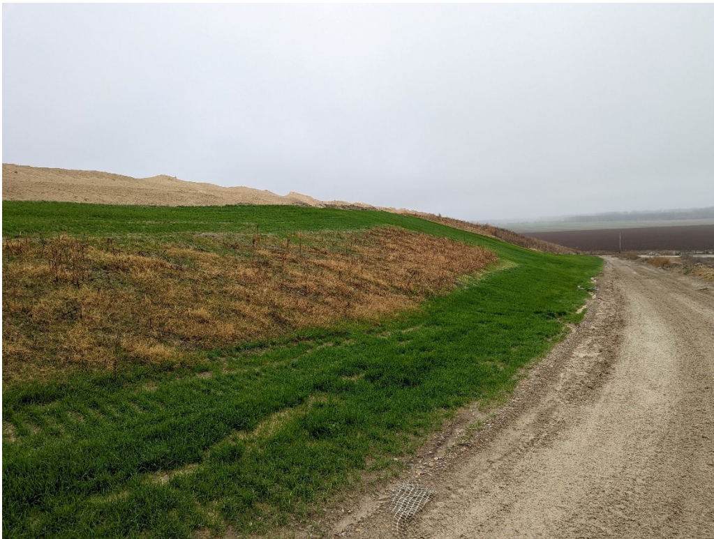
Photo 6. Cell 3 East slope intermediate cover and haul road.
