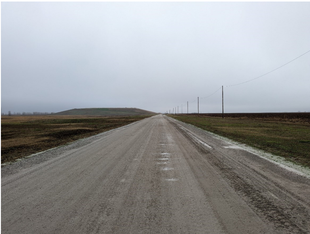
Photo 2. Haul road to landfill from East.
