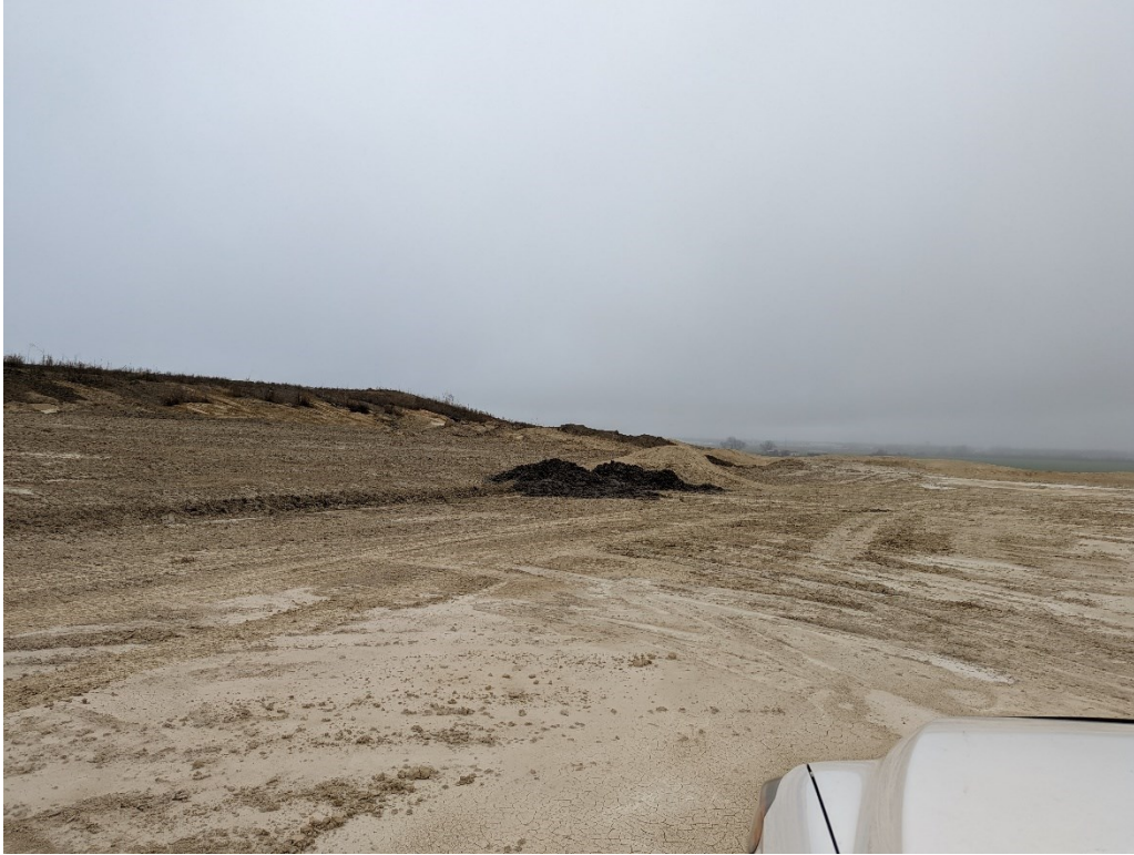
Photo 5. Cell 3 working face looking Northwest at Cell 1 top elevation.
