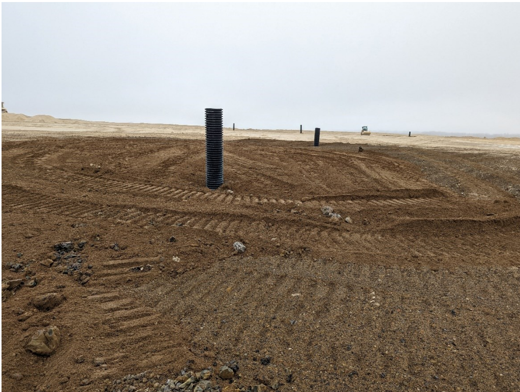
Photo 4. Active working face, bottom ash with chimney drains (Cell 3).
