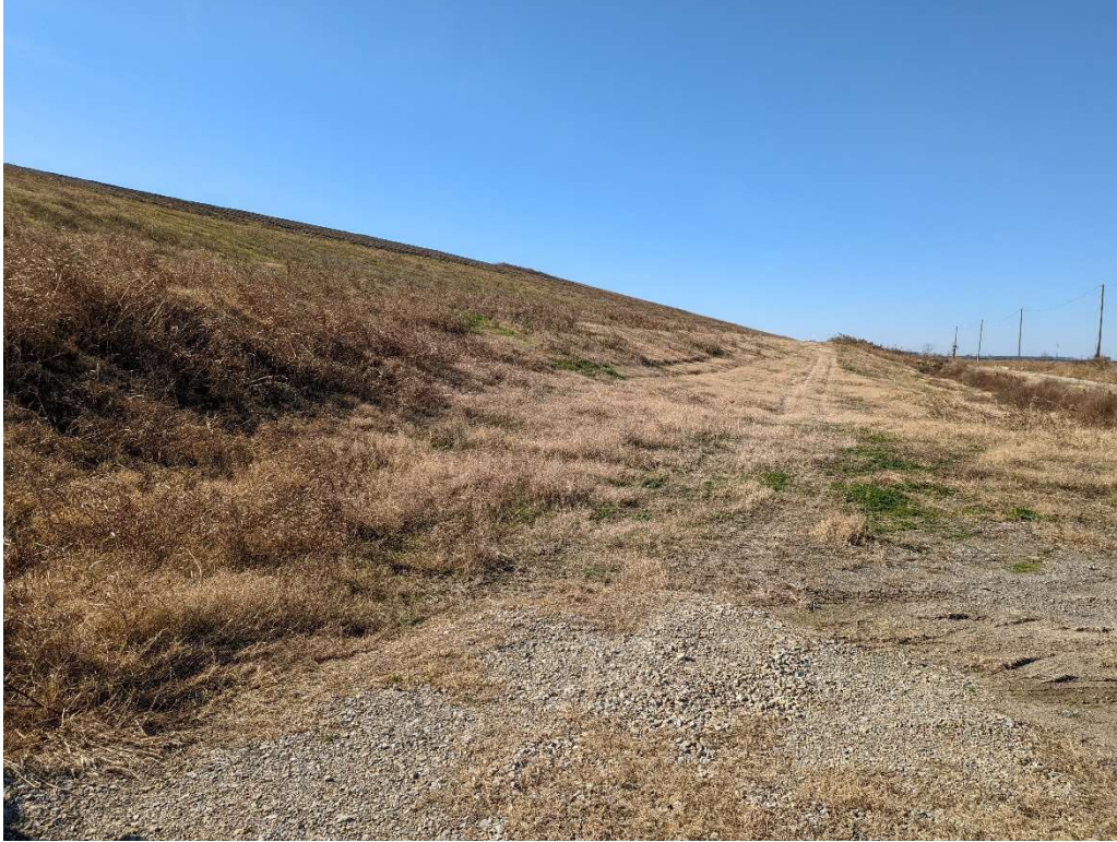
Photo 5. Cell 3 north slope intermediate cover.
