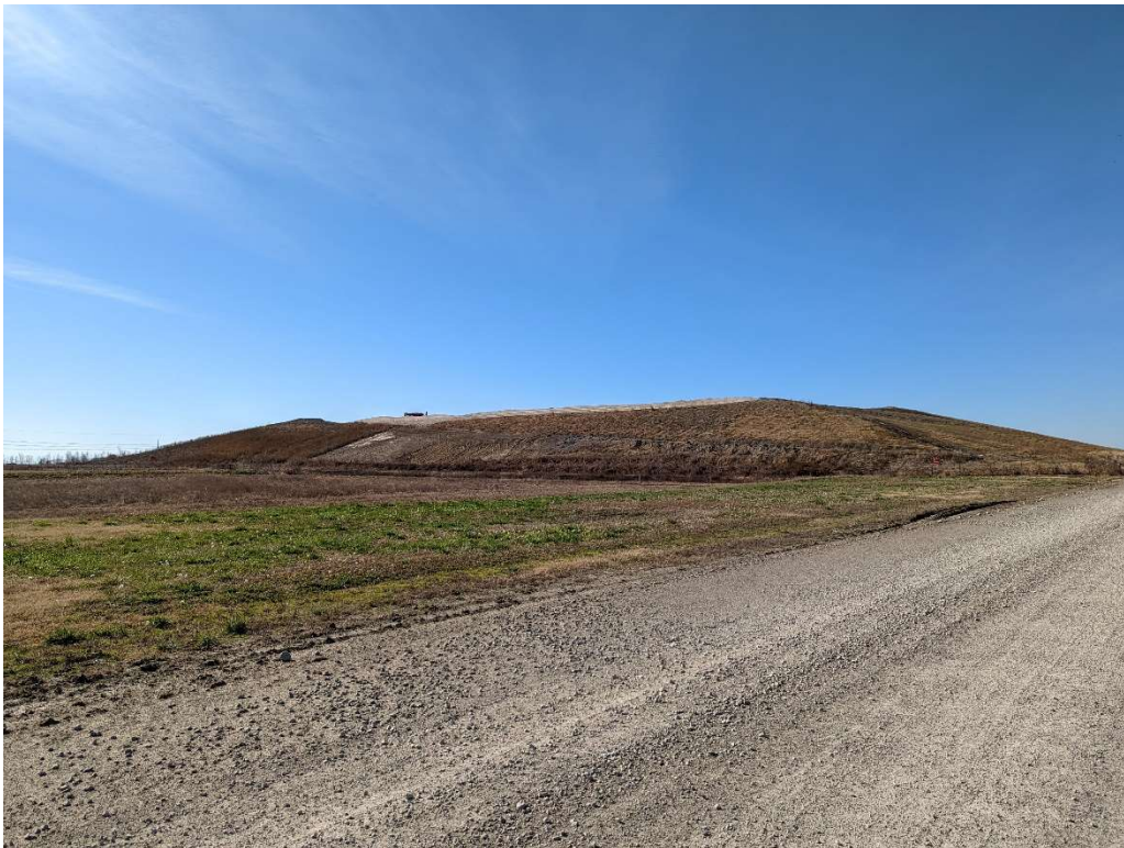
Photo 4. Haul road to landfill from East.
