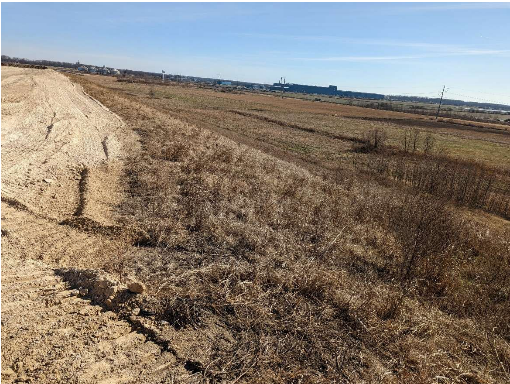
Photo 6. Cell 3 south slope intermediate cover.
