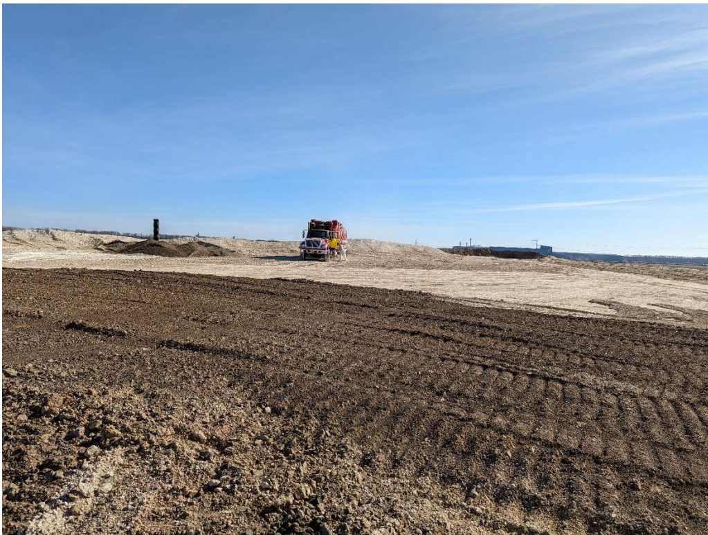
Photo 2. Water truck prepared to water active area (Cell 3).
