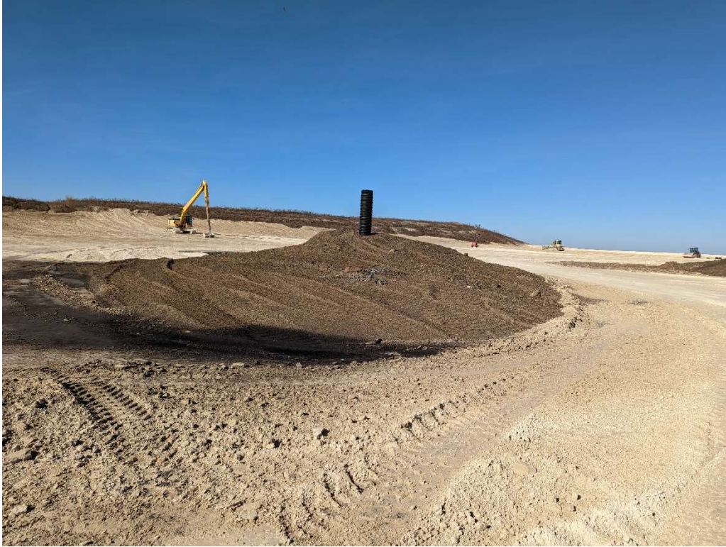
Photo 3. Active working face with chimney drain in foreground. (Cell 3).
