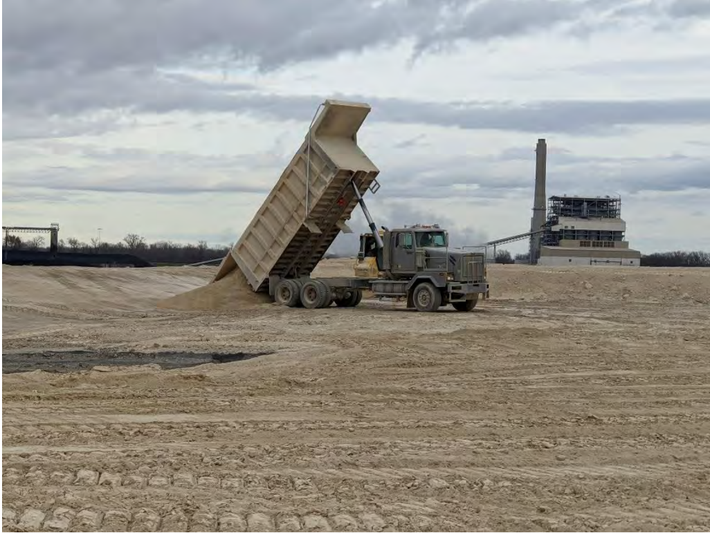
Photo 3. Active waste dumping (Cell 3).
