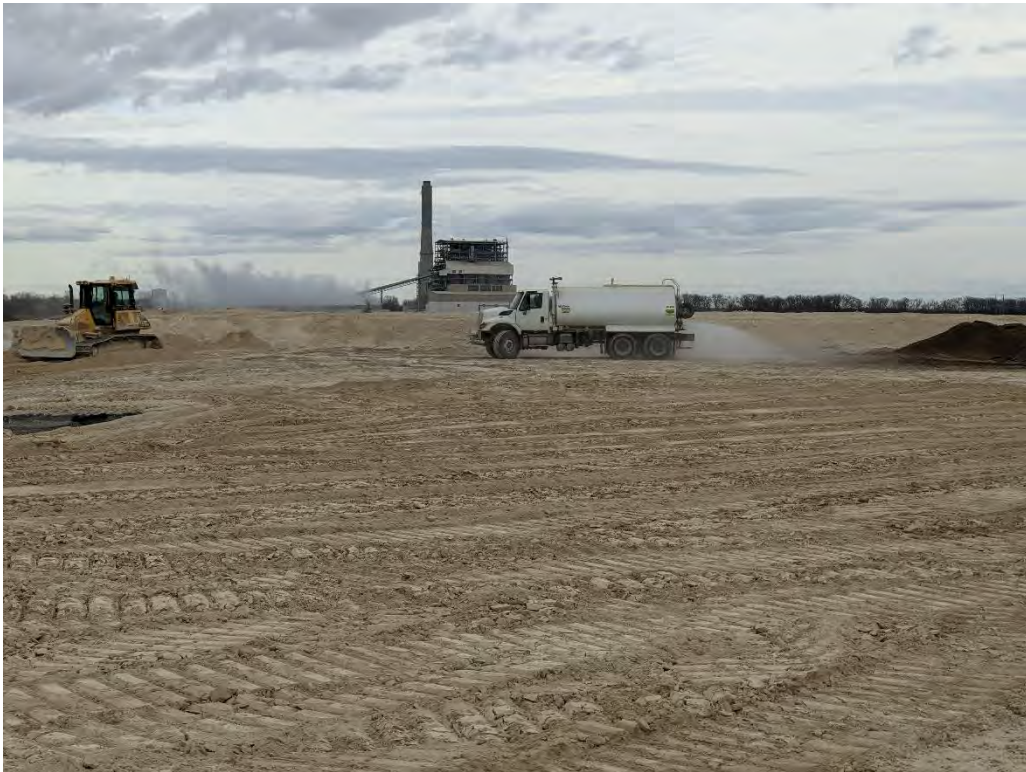
Photo 2. Active watering of active disposal area (Cell 3).
