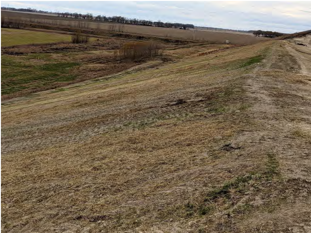
Photo 6. Cell 3 south slope intermediate cover and seeding.
