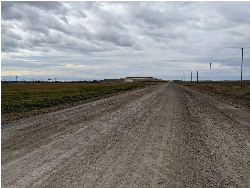
Photo 4. Haul road to landfill from East.
