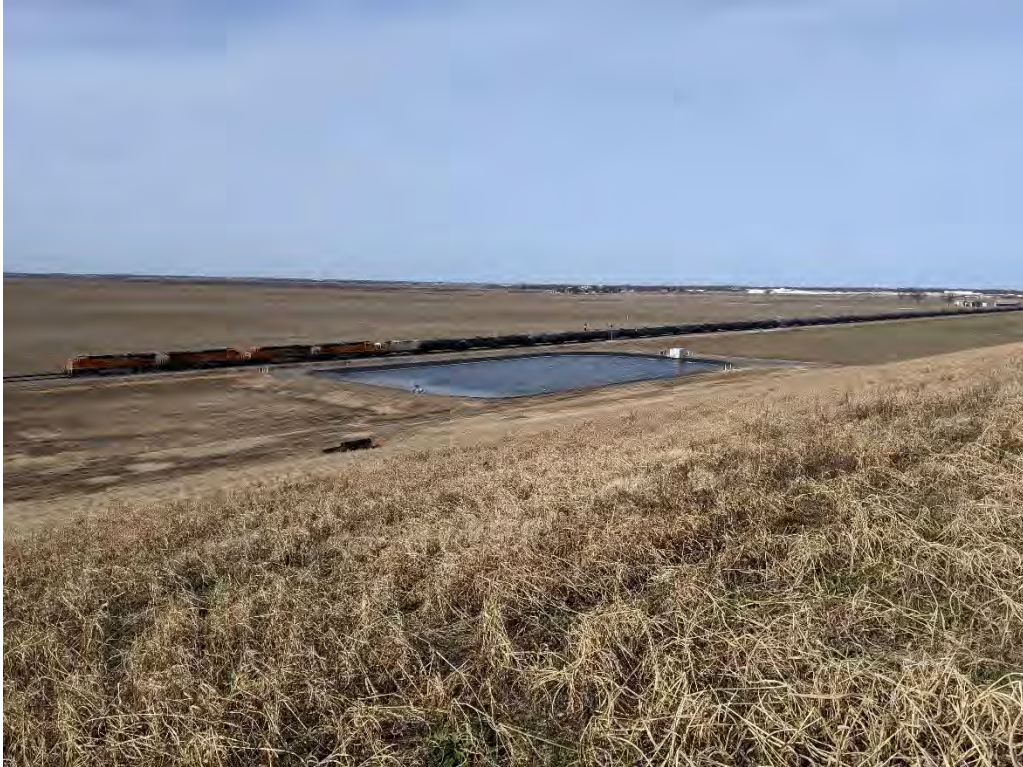
Photo 6. West slope Cell 1 under intermediate cover with leachate pond in background
