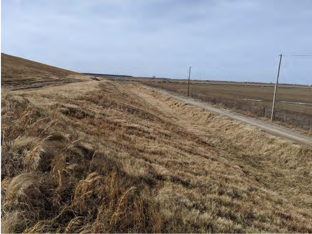
Photo 5. Landfill perimeter berm and stormwater ditch looking west
