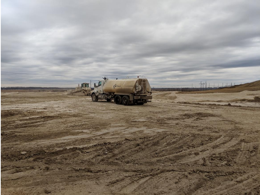
Photo 4. Water truck preparing to wet Cell 3
