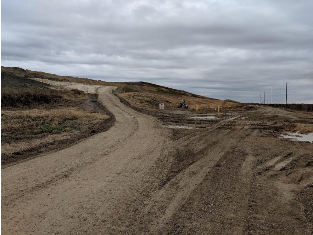
Photo 3. Haul road looking towards Cell 3
