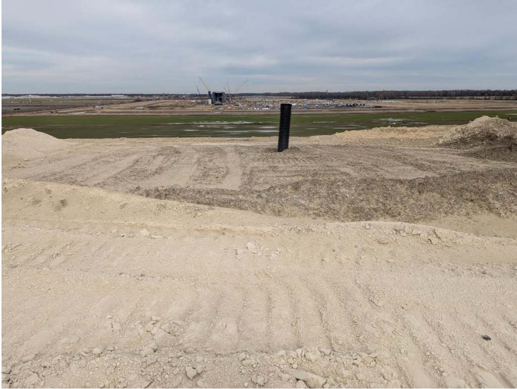
Photo 3. Active working face, fly ash looking North (Cell 3).
