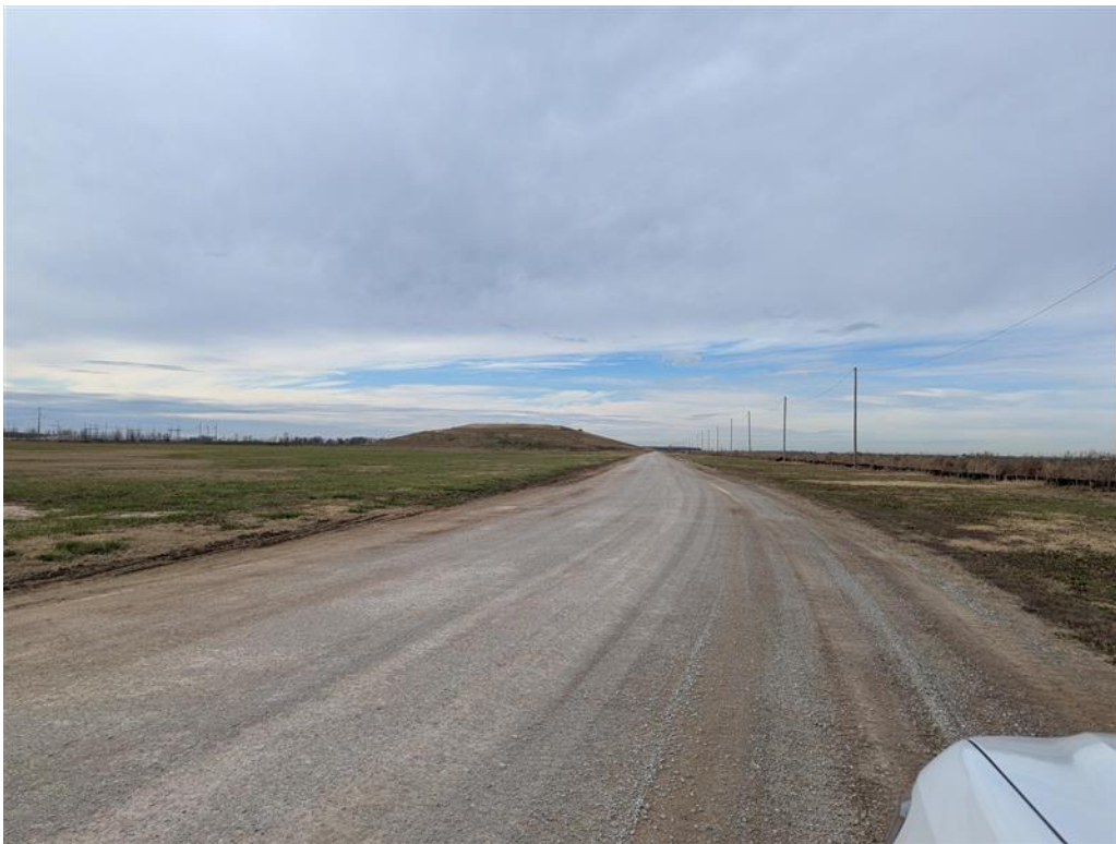
Photo 2. Main haul road to landfill looking West with landfill in the
