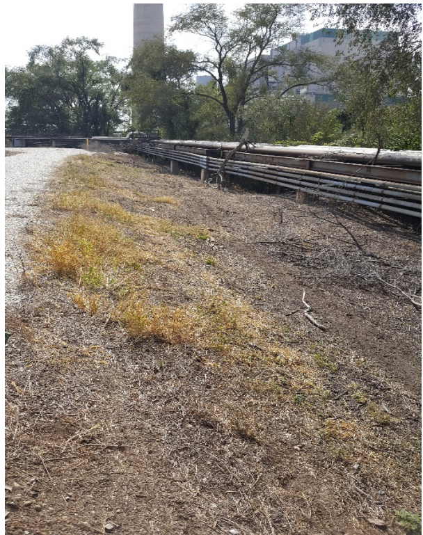
4. Metal Cleaning Basin West Slope
