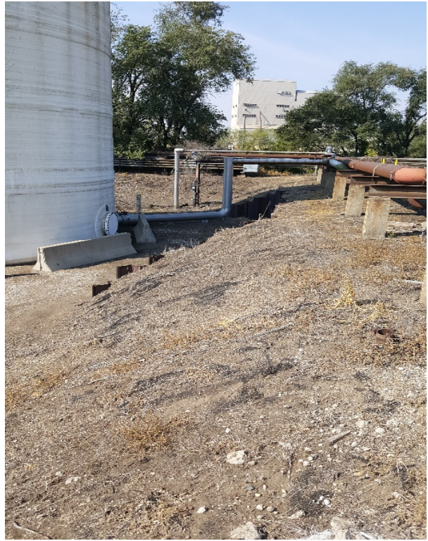
2. Metal Cleaning Basin South Slope
