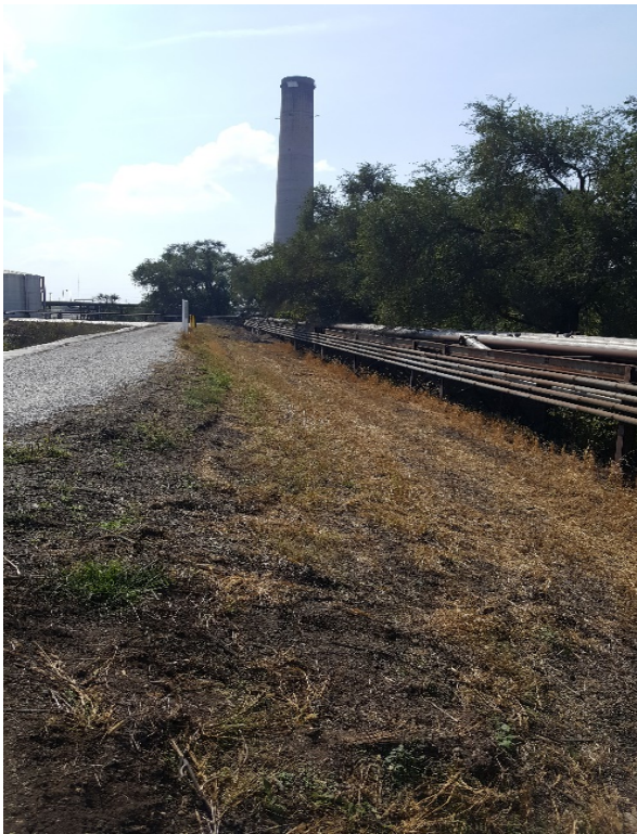
3. Metal Cleaning Basin West Slope
