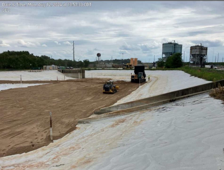
Photo 1: Placement of structural fill on the base of the bypass basin.
