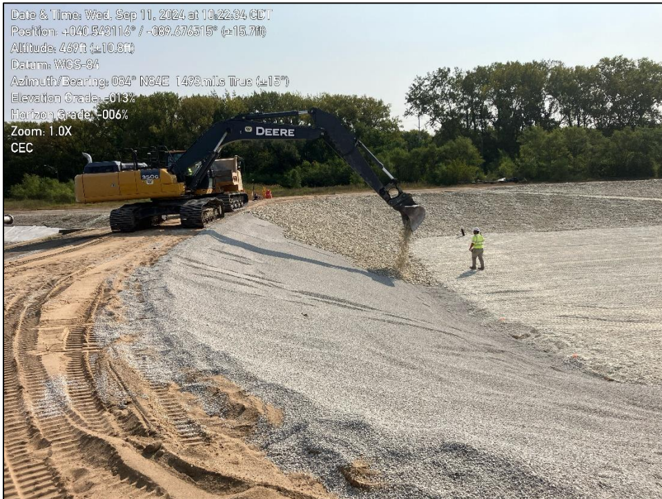
Photo 1: shows placing of rip rap along northern slope.
