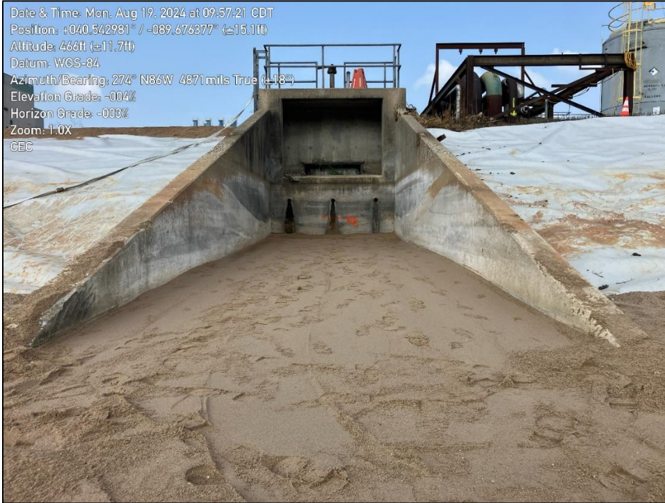
Photo 1: Structural fill inside concrete inlet structure.
