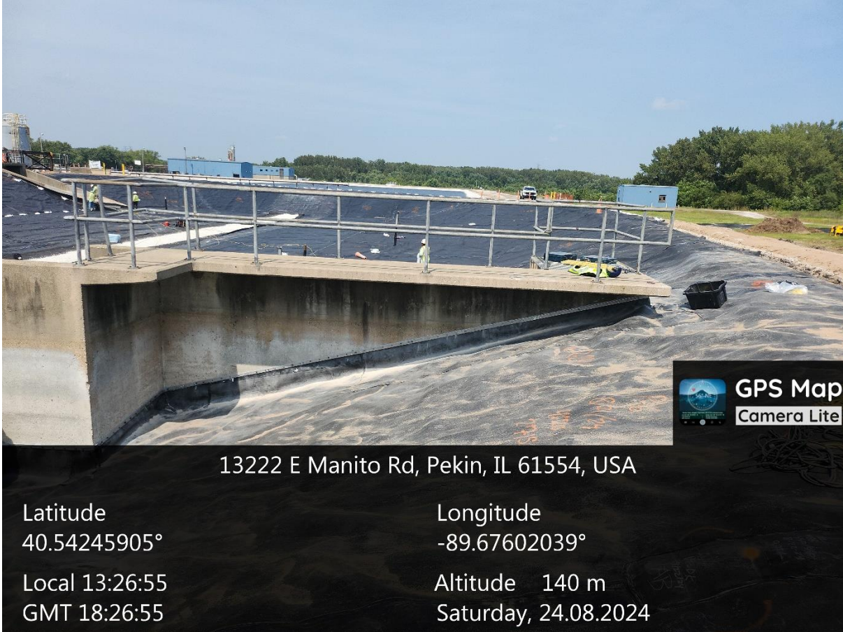
Photo 2: photo shows the completed liner edge attached to the south east concrete structure
