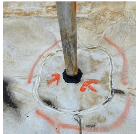
(b) Additional Extrudate Placed Around Marker Post
