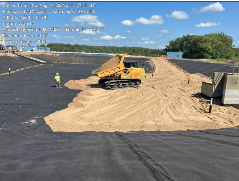
Photo 2: shows the sand drainage layer being placed within the basin.
