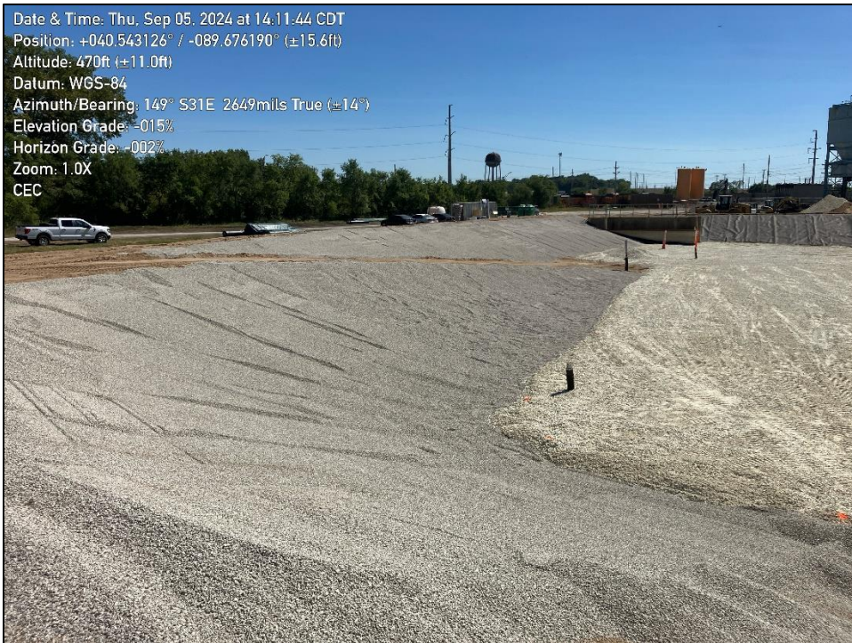
Photo 2: shows rip rap bedding layer on northeast slope.
