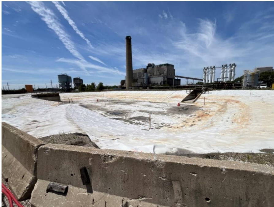
Figure 4. Cleaned and Decontaminated Bypass Basin (Looking Southwest).
