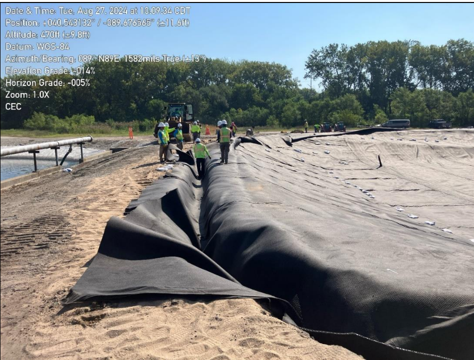
Photo 2: shows the CAAWS crew placing liner inside anchor trench.
