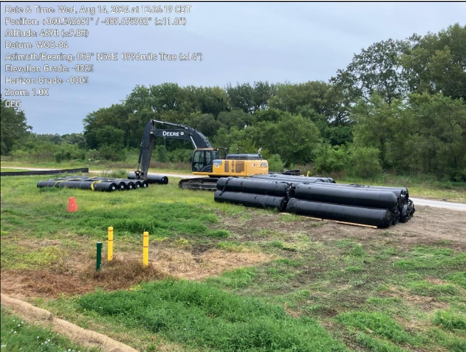
Photo 1: Staging area for liners.
