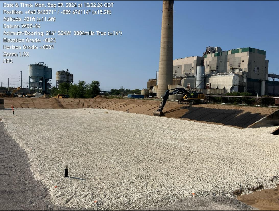
Photo 1: shows placing sand filter layer along western slope.
