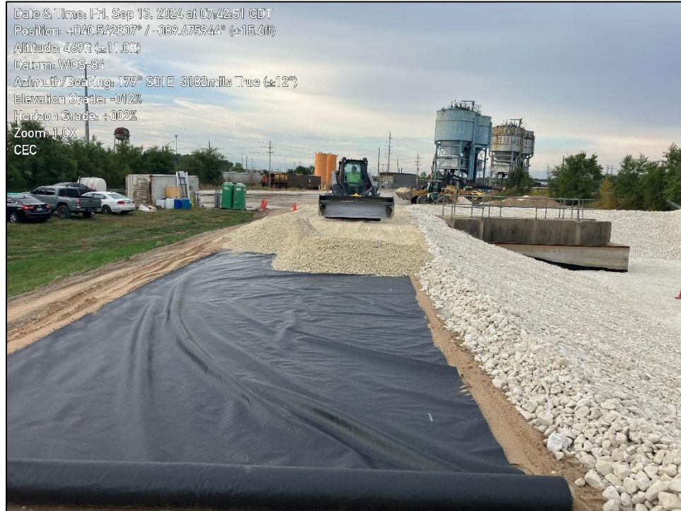
Photo 1: shows placing of road surfacing along eastern perimeter road.
