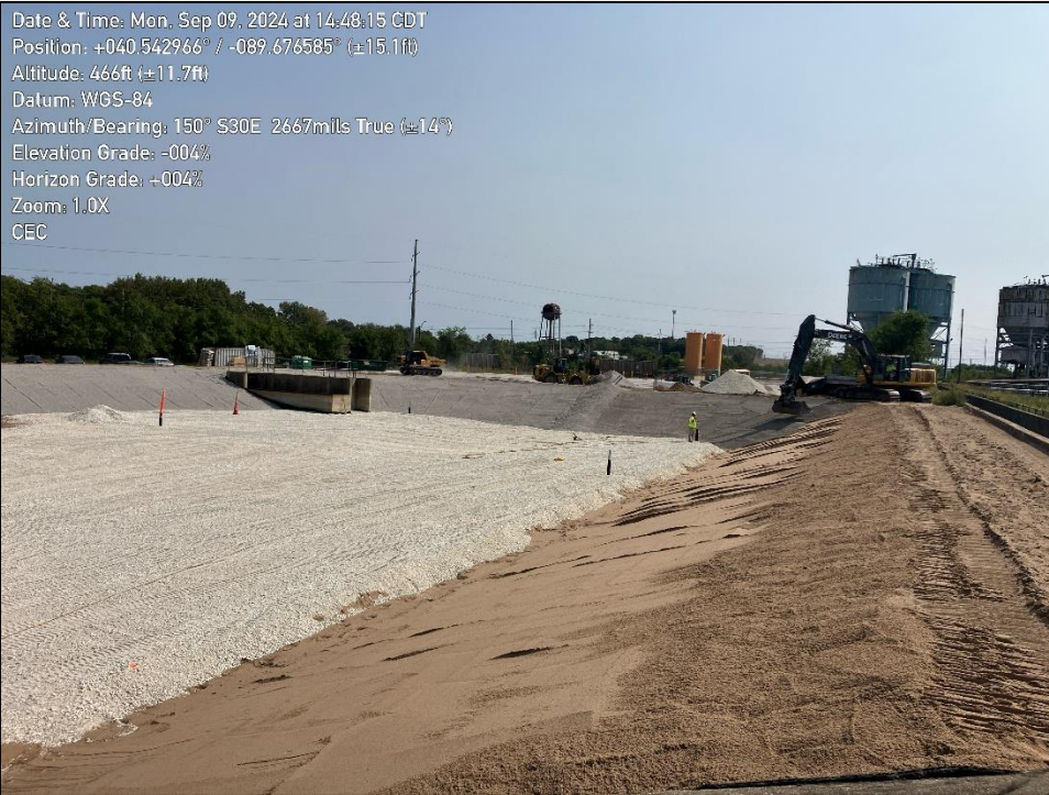
Photo 2: shows placing of rip rap bedding layer on western slope.
