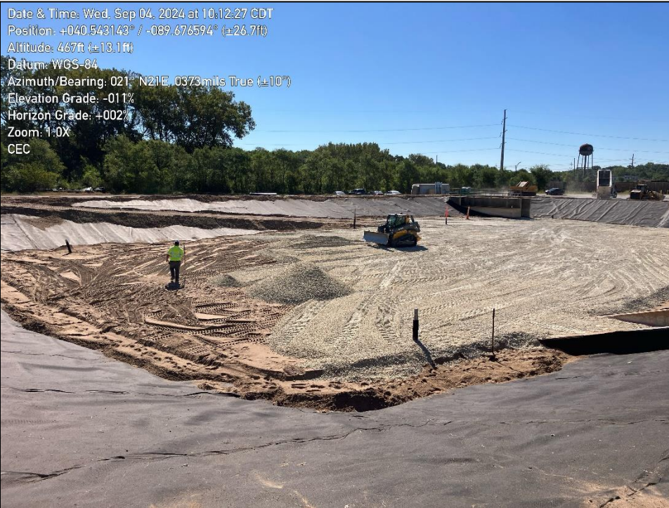
Photo 1: shows protective warning layer being installed within basin floor.
