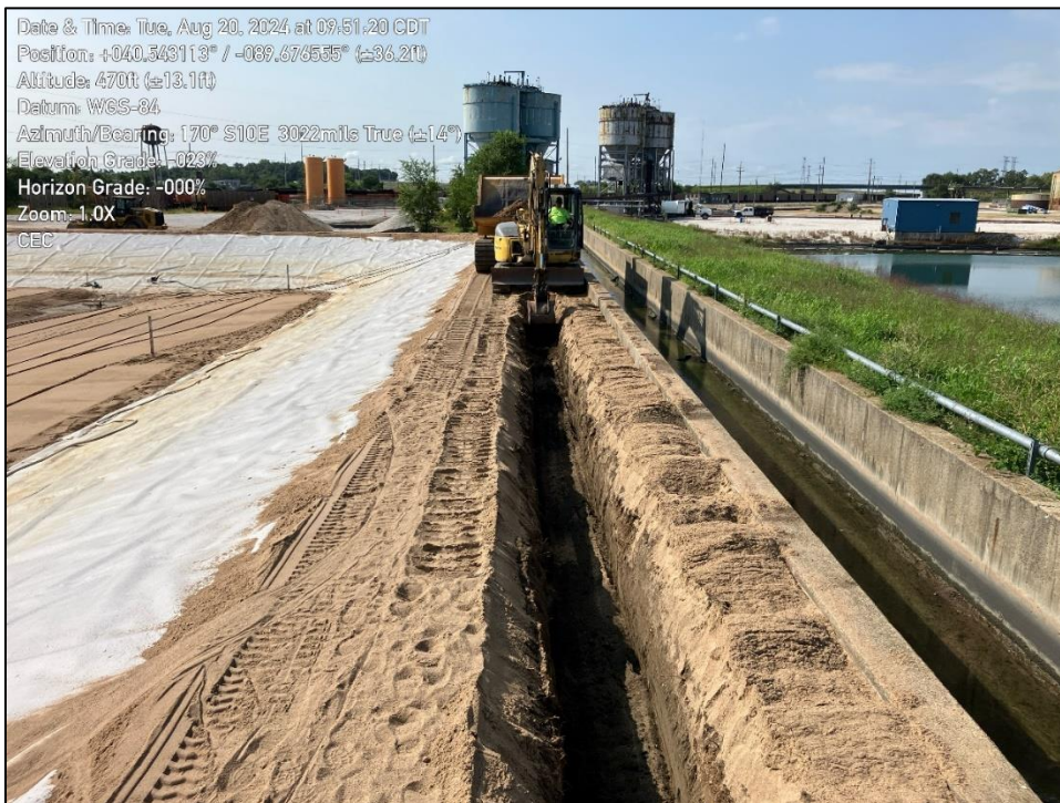
Photo 2: Excavated anchor trench on west side.
