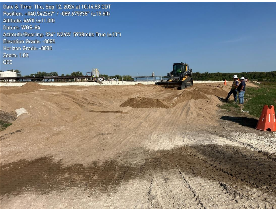
Photo 2: shows grading of southeastern perimeter ramp.
