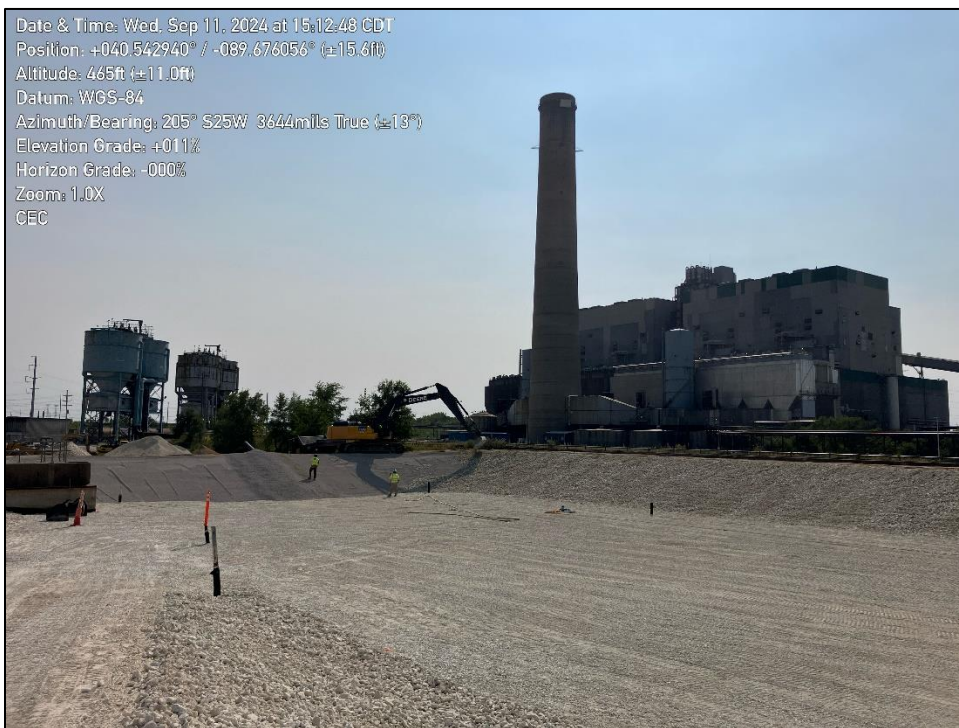
Photo 2: shows placing of rip rap along the western slope.
