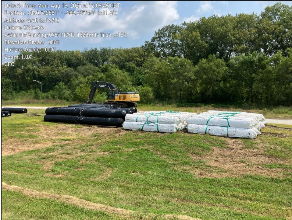
Photo 3: Staged GCL rolls.
