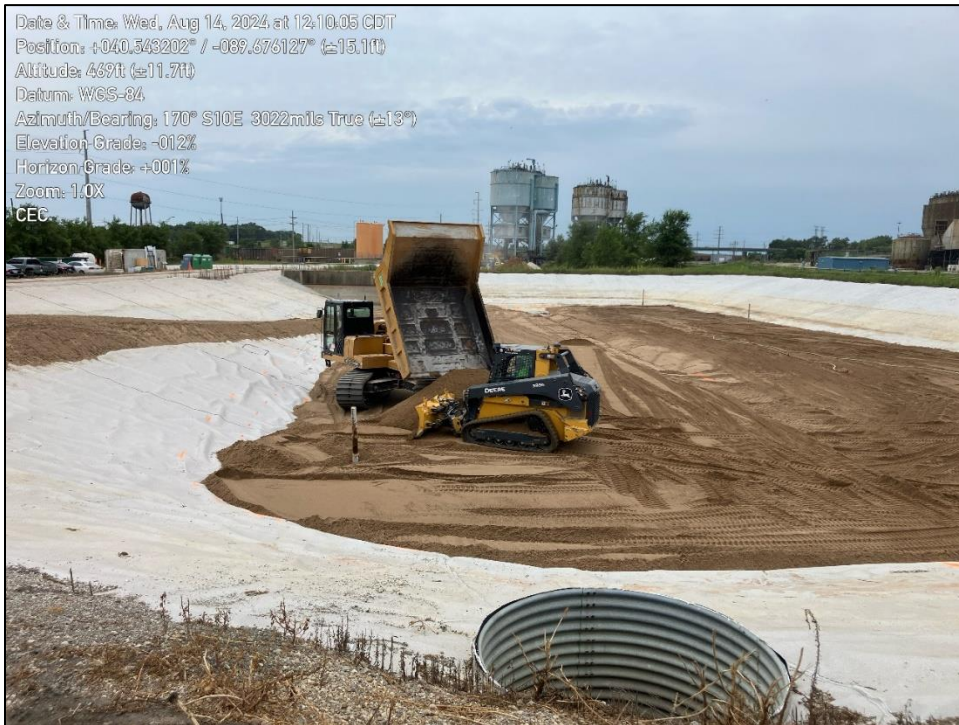
Photo 2: Placing 3 rd lift of structural fill.
