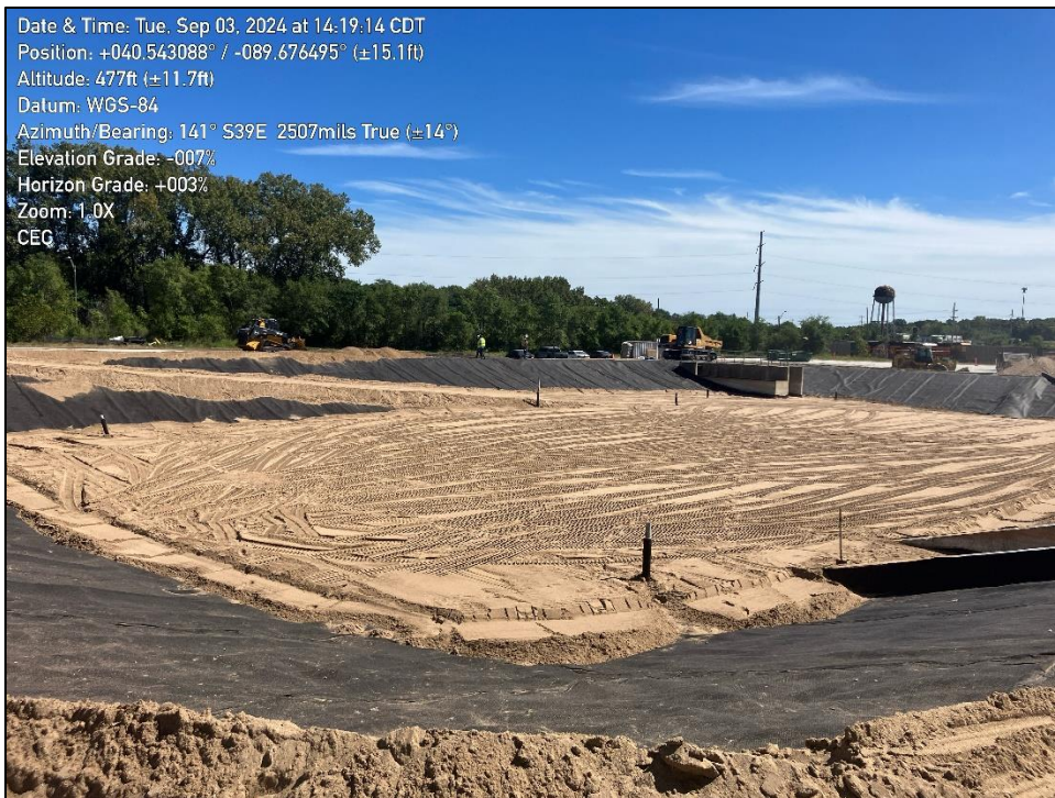
Photo 2: shows the completed sand filter layer within basin.
