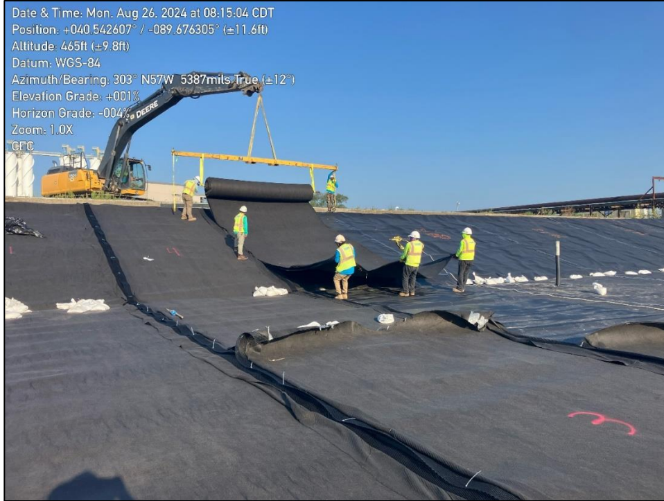
Photo 1: shows CAAWS crew deploying drainage geocomposite.
