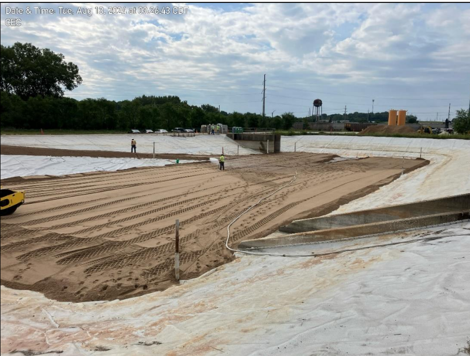
Photo 3: Moisture conditioning of structural fill.
