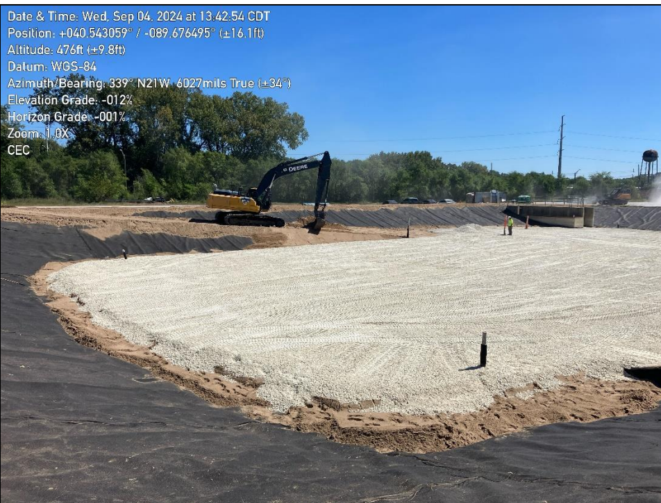
Photo 2: shows the sand filter layer being placed on slope of ramp.
