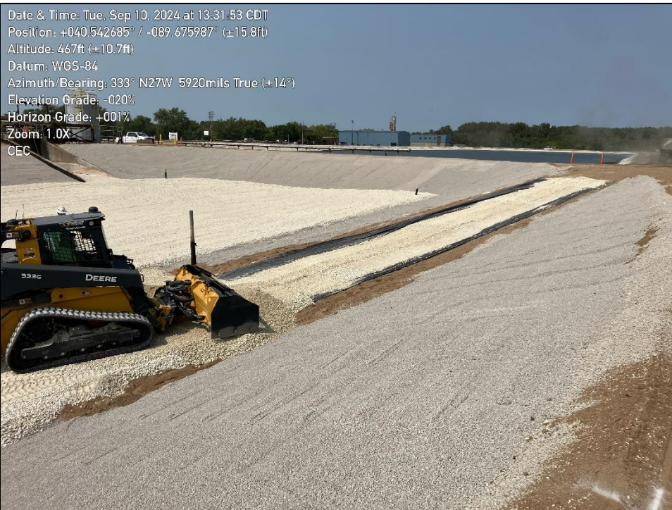
Photo 2: shows placing of road surfacing on the basin's ramp.
