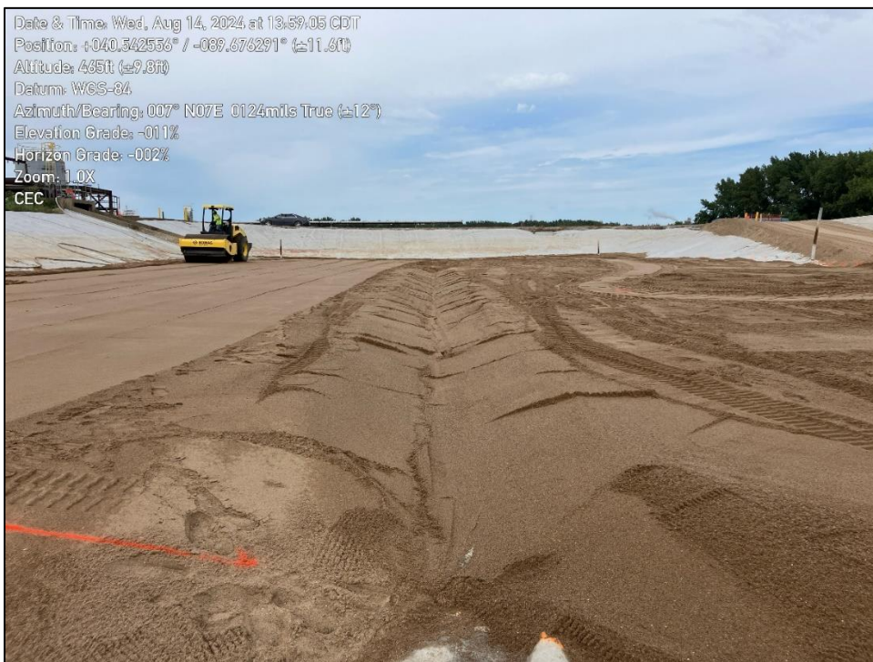
Photo 3: View of the center trench.
