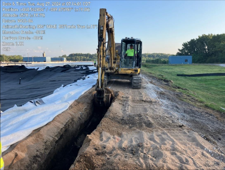
Photo 1: shows BCC excavating anchor trench.
