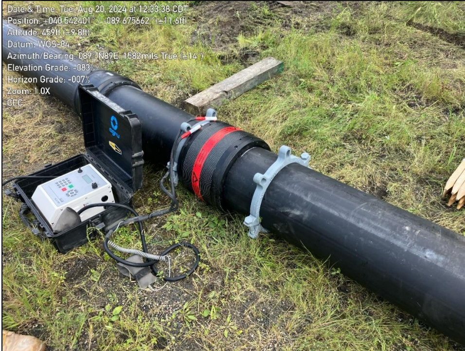
Photo 3: Electrofusion coupler on 12" HDPE pipe
