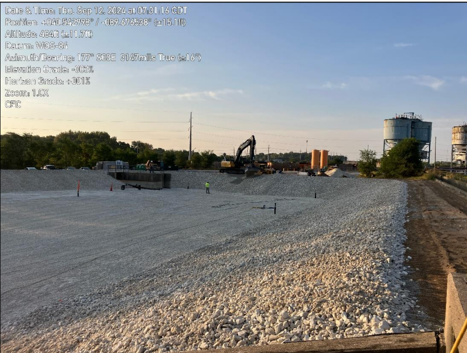
Photo 1: shows placing of rip rap along southern slope.
