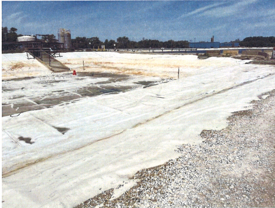
Figure 7. Cleaned and Decontaminated Bypass Basin (Looking Northwest).
