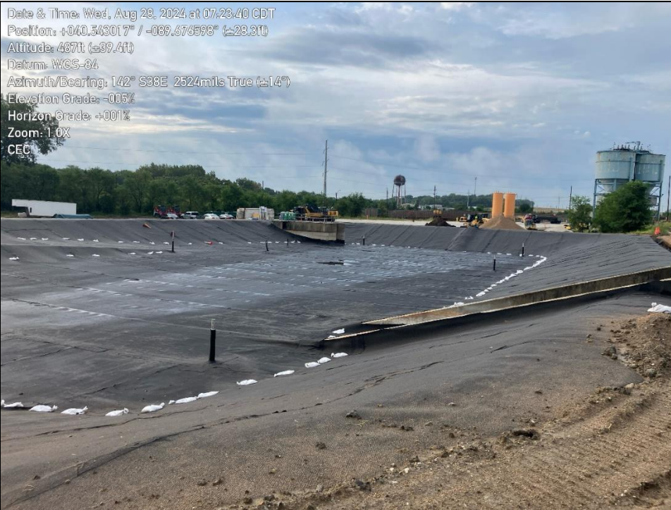
Photo 1: shows water within basin before being pumped out.
