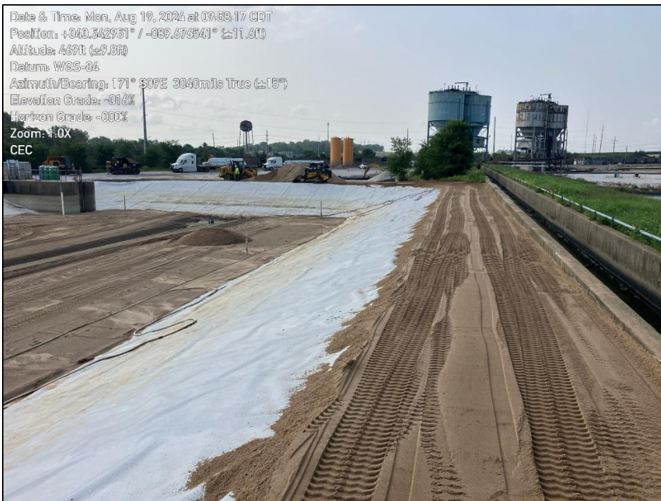
Photo 2: Lower sand cushion layer on west side.
