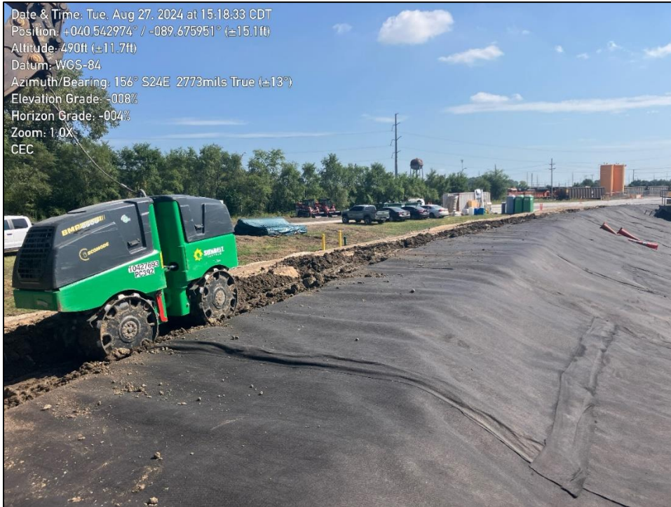
Photo 3: shows BCC compacting the anchor trench backfill.
