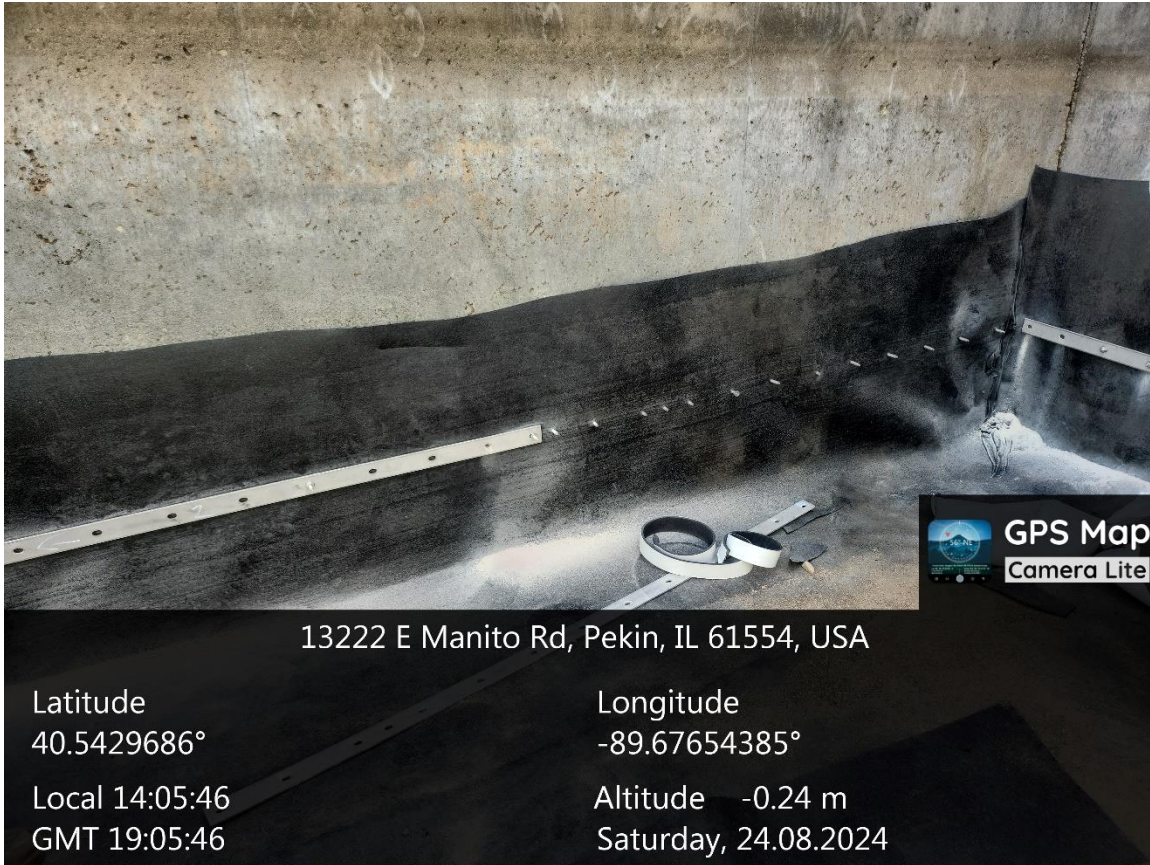
Photo 3: shows the CAAWS crew bolting the liner into position within the north west concrete inlet.
