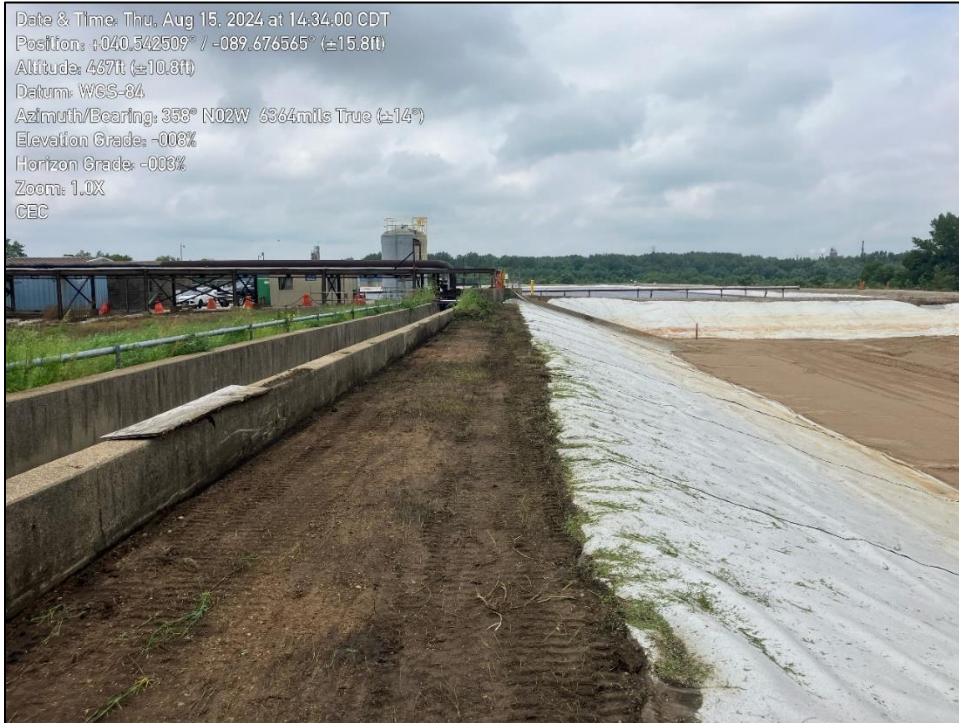
Photo 1: Cleared anchor trench area on west side.
