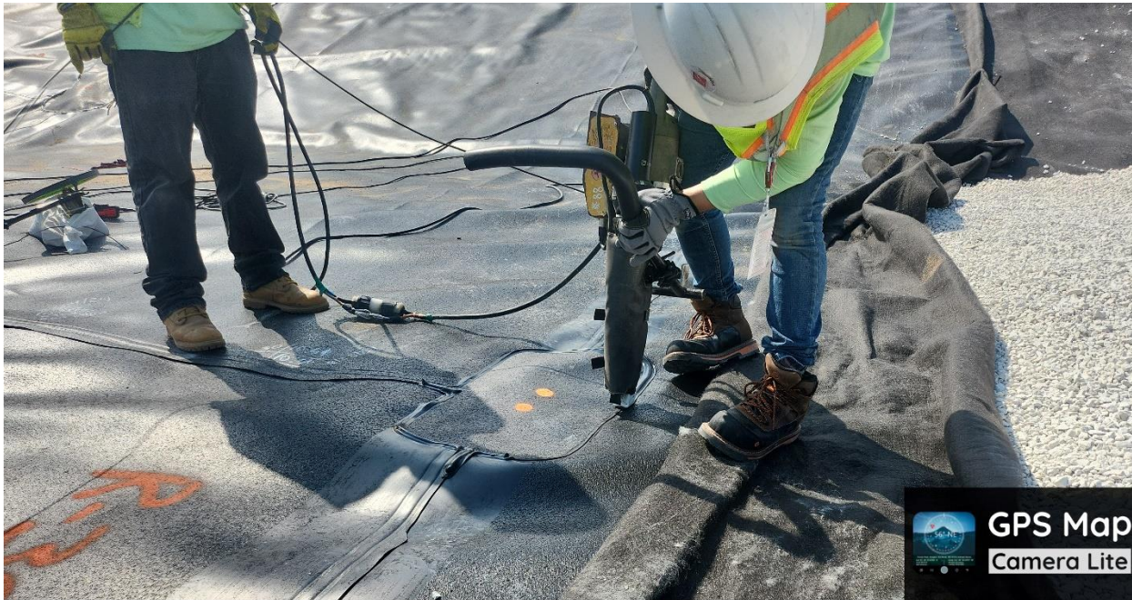
Photo 1: shows CAAWS crew making repairs along the southeast basin floor.
