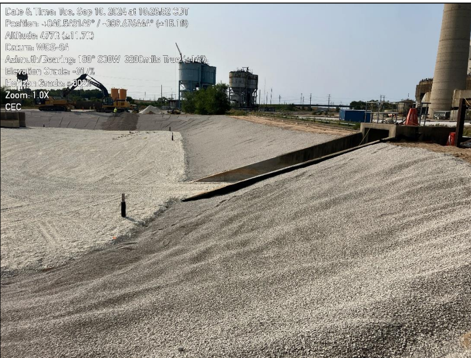
Photo 2: shows completed rip rap bedding layer along basin's slopes.
