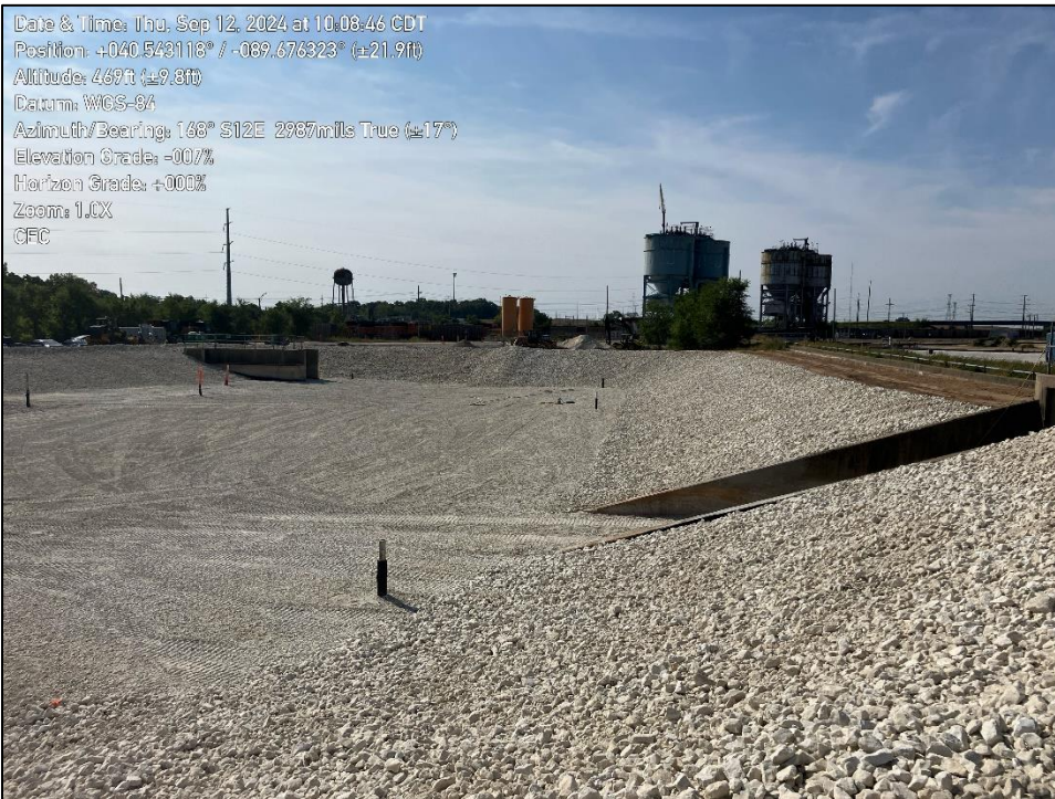
Photo 4: shows basin with completed layers of aggregates.
