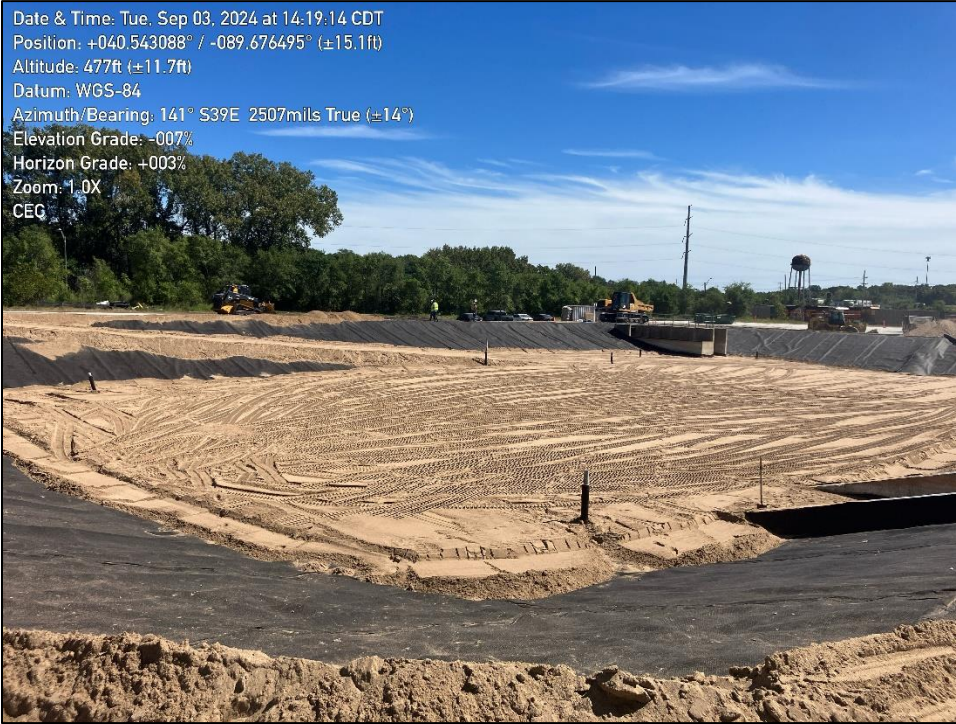
Photo 1: shows completed sand filter layer along bottom of basin.
