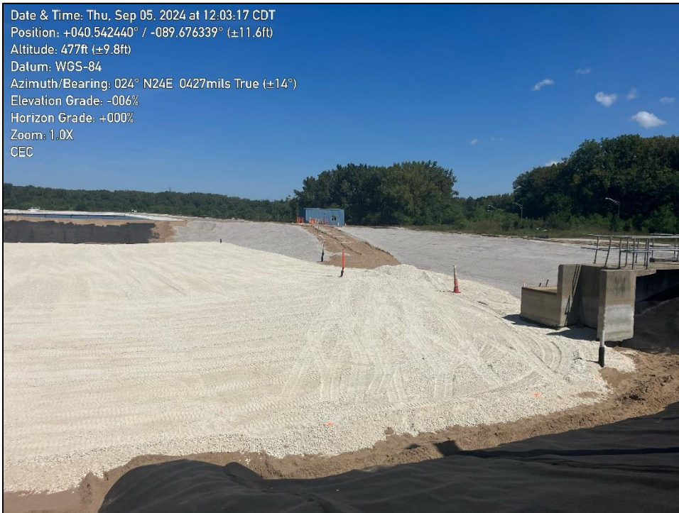
Photo 4: shows basin with protective warning layer and rip rap bedding layer.
