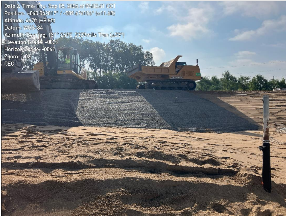
Photo 3: shows placement of rip rap bedding layer along eastern slope.
