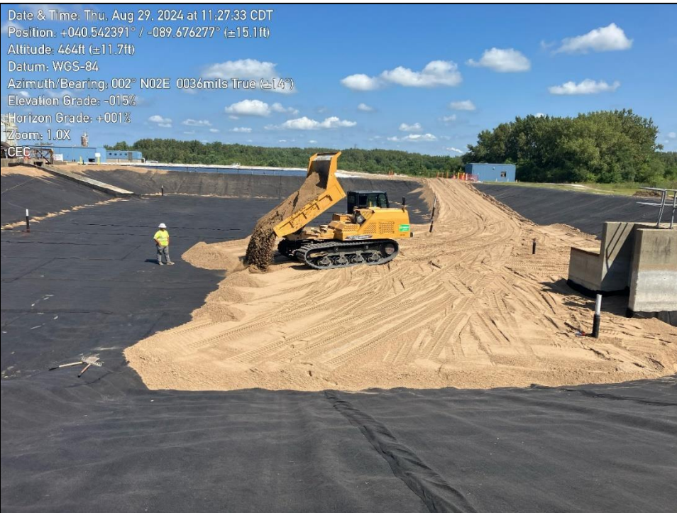
Photo 4: shows placement of sand filter layer.
