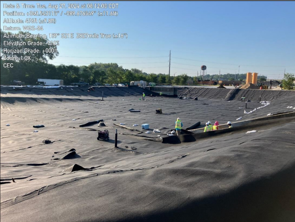
Photo 2: shows completion of drainage geocomposite installation.
