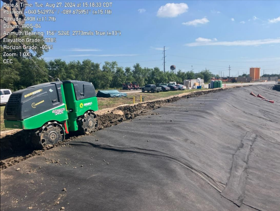
Photo 3: shows compaction of anchor trench backfill.
