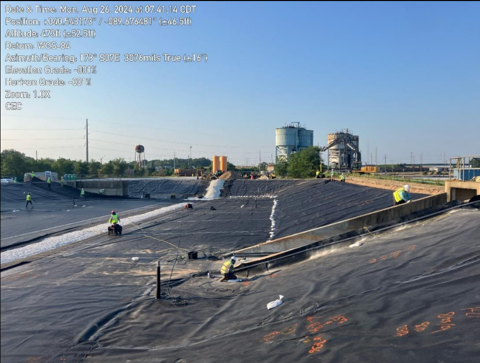
Photo 1: shows deployment of drainage geocomposite and completion of geomembrane installation.
