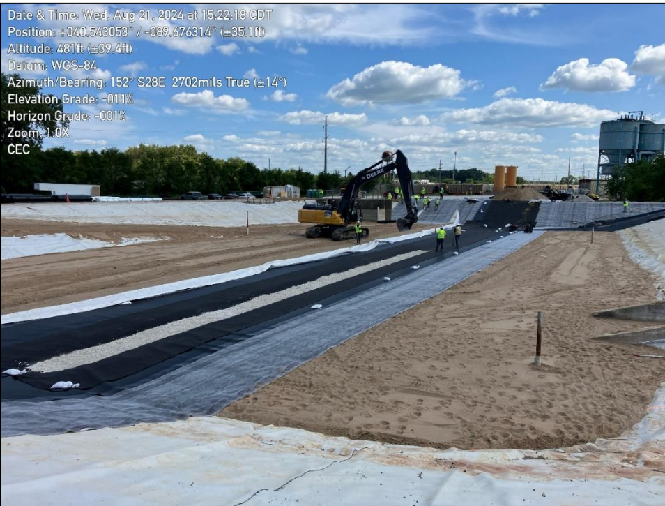
Photo 3: shows deployment of GCL, geomembrane, and installation of CAB.
