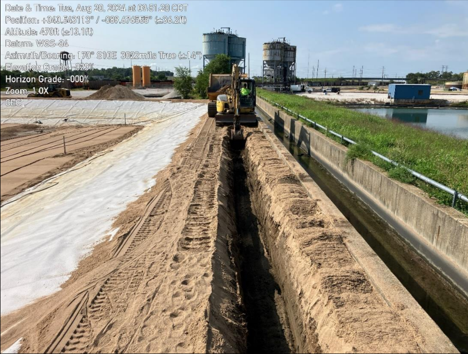
Photo 2: shows excavation of anchor trench.
