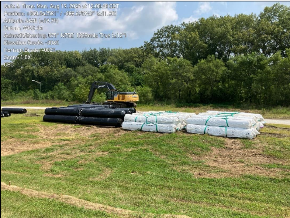
Photo 1: shows storage of liner.
