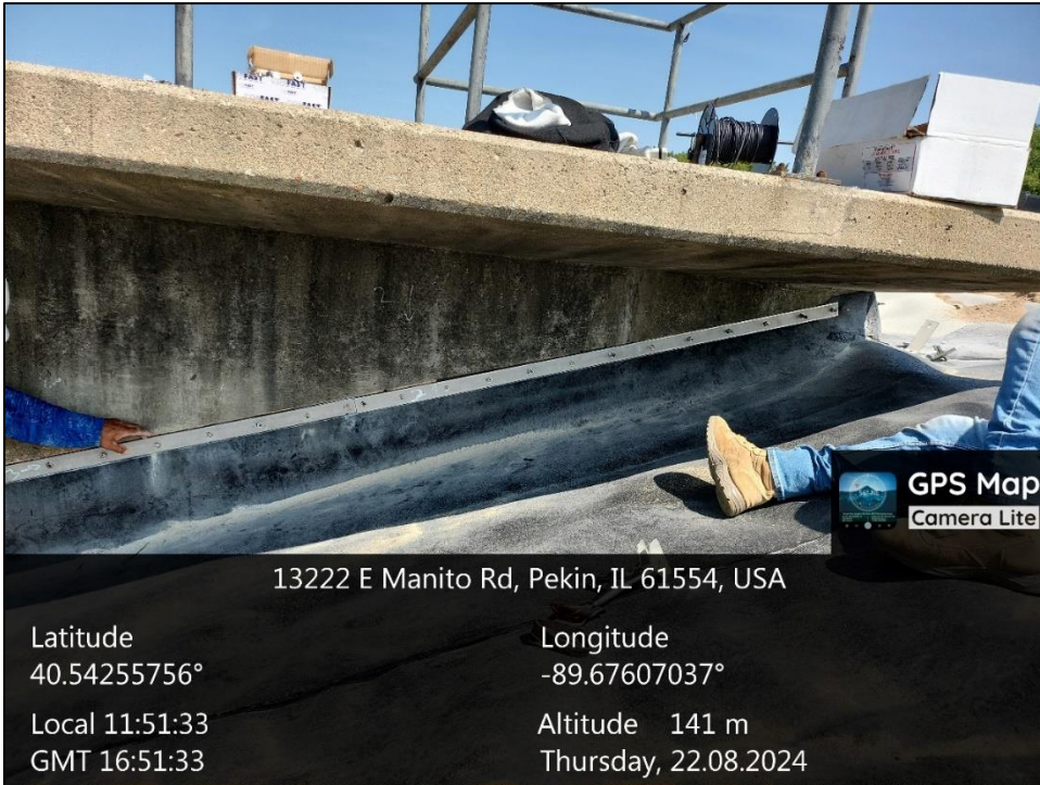
Photo 4: shows batten strips along outlet structure.
