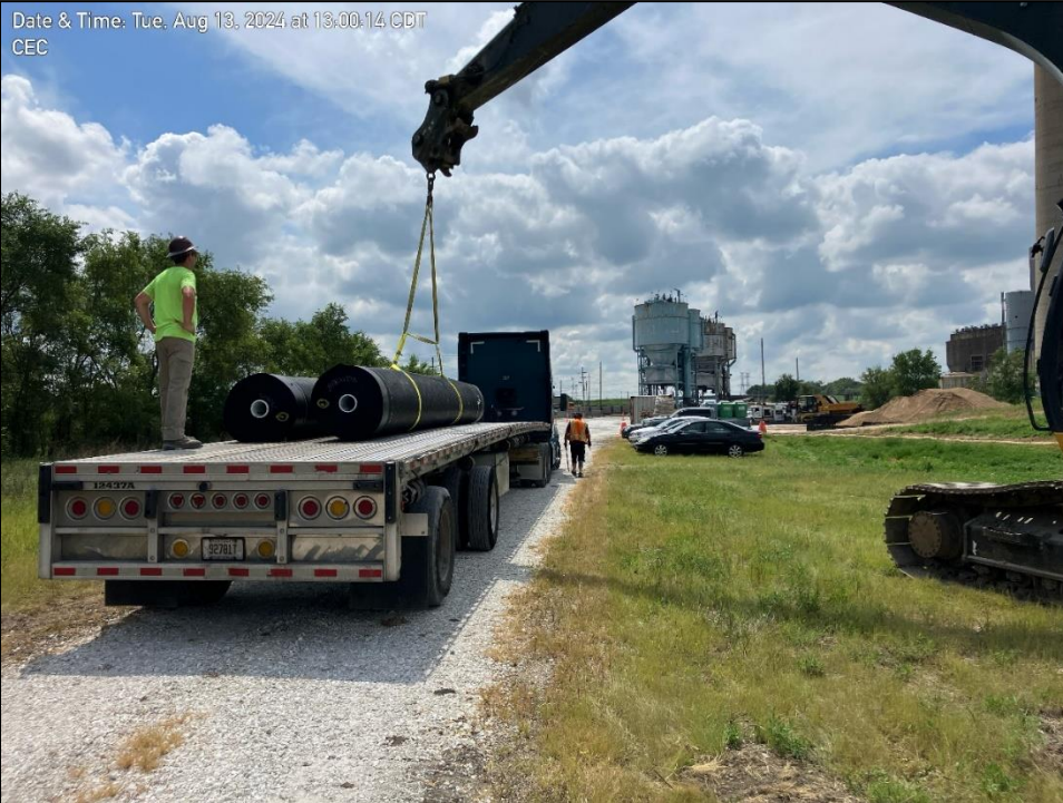
Photo 2: Unloading of HDPE geomembrane.
