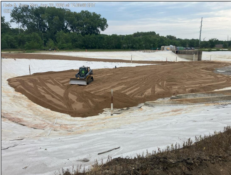
Photo 1: Grading of the 1 st lift of structural fill.
