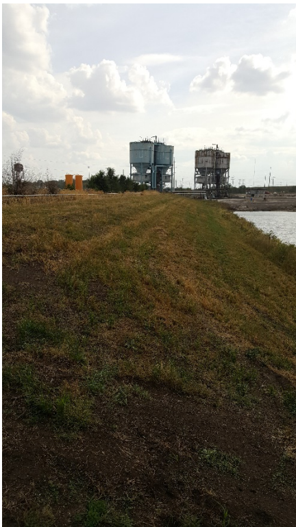
3. Ash Bypass Basin West Slope
