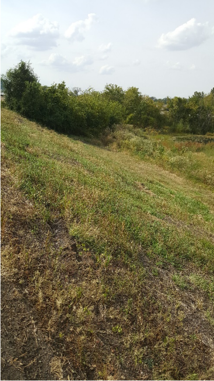
5. Ash Surge Basin North Slope
