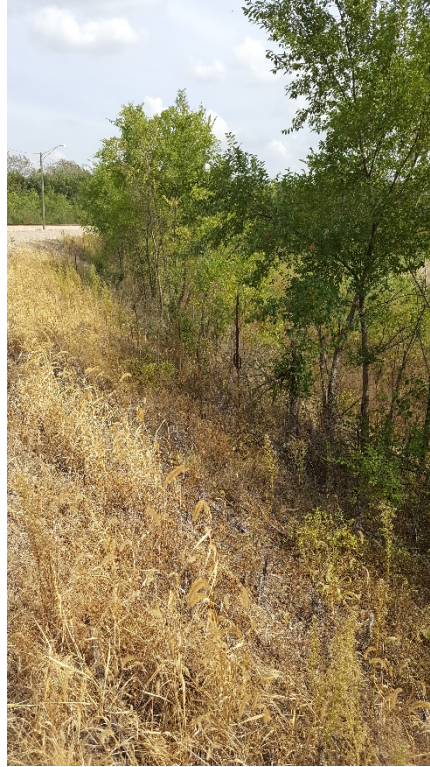
6. Southern Section of Former Ash Basin Northeast Slope
