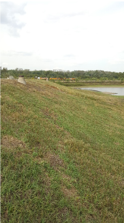
3. Ash Surge Basin East Slope
