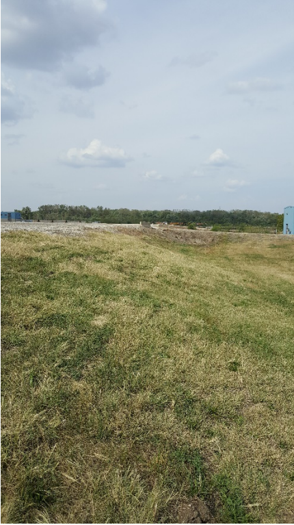
1. Ash Surge Basin East Slope
