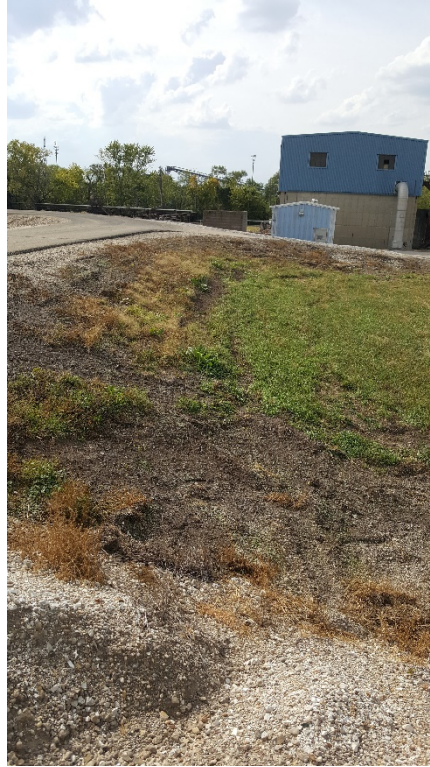
6. Ash Surge Basin North Slope
