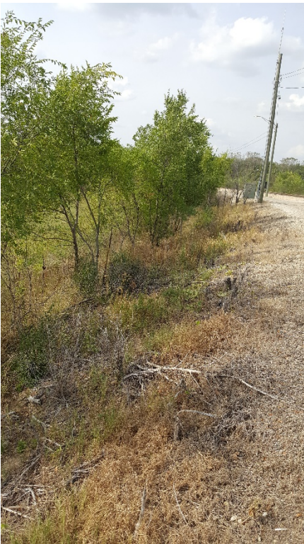
7. Southern Section of Former Ash Basin Northwest Slope
