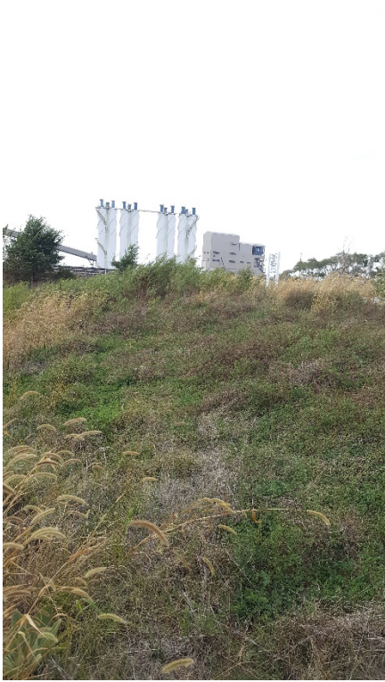
1. Ash Bypass Basin South Slope
