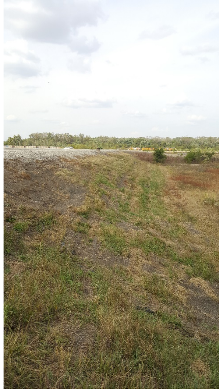
2. Ash Surge Basin East Slope
