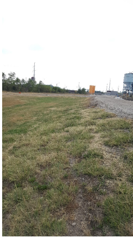
2. Ash Bypass Basin East Slope
