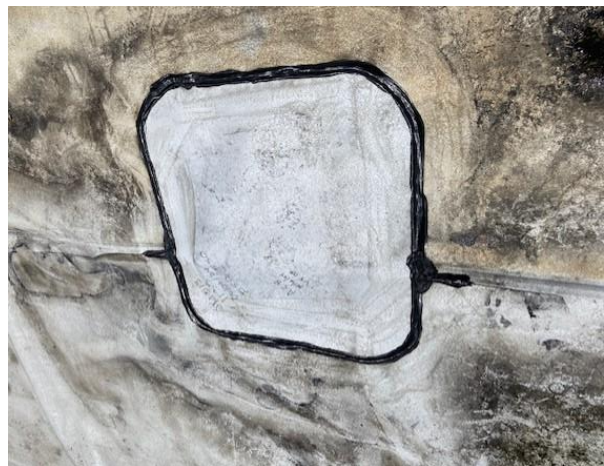
(b) HDPE Geomembrane Patch Welded Over Location 1
