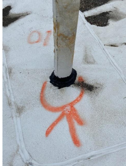
(b) Additional Extrudate Placed Around Marker Post
