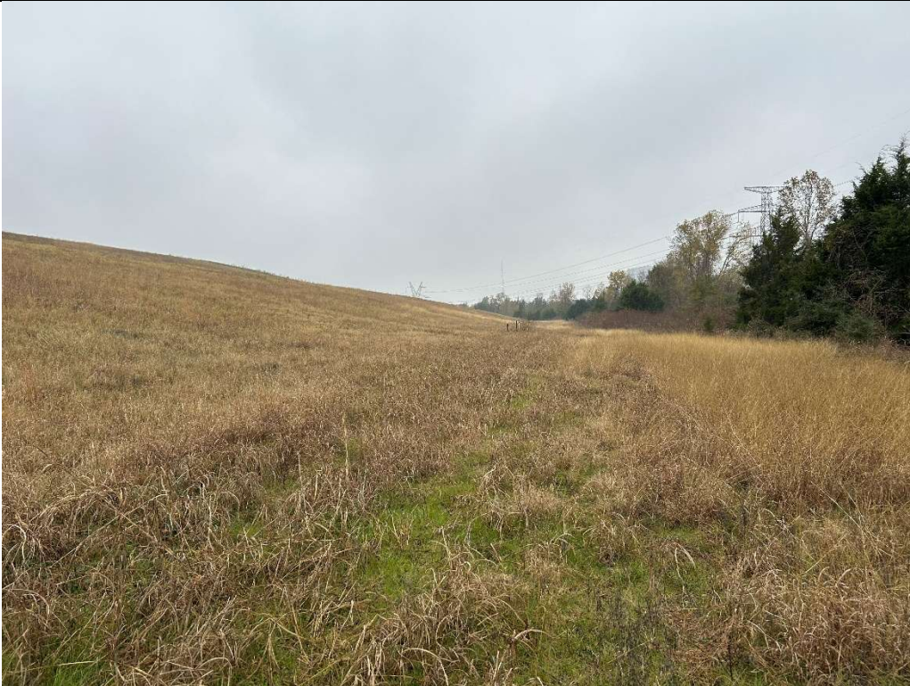
Photograph P-6: View looking southeast up the side slope of Area 2. The terraced slope is well vegetated with no visible sloughing or erosional issues.
