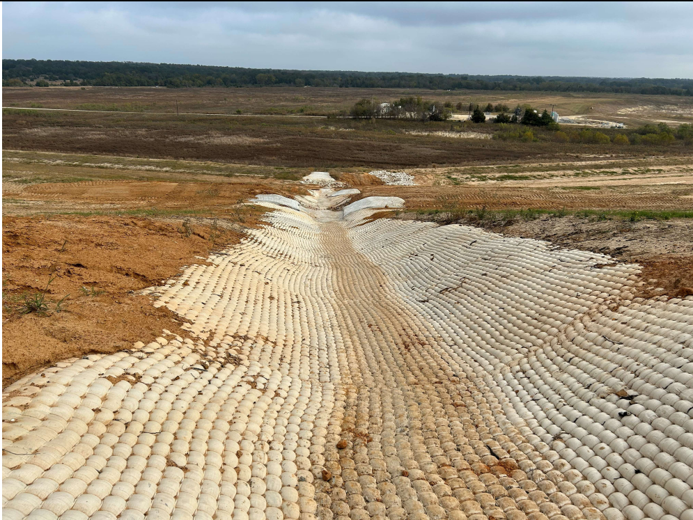
Photograph P-10: View looking northeast down concrete rundown channel in Area 3.
