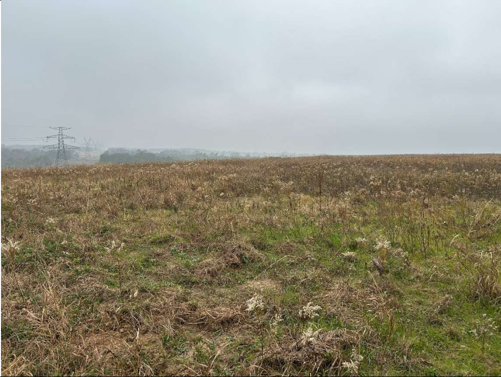
Photograph P-1: View looking southeast across the capped surfaces of Areas 1 and 2. The landfill cap appeared to be well vegetated and appropriately sloped.
