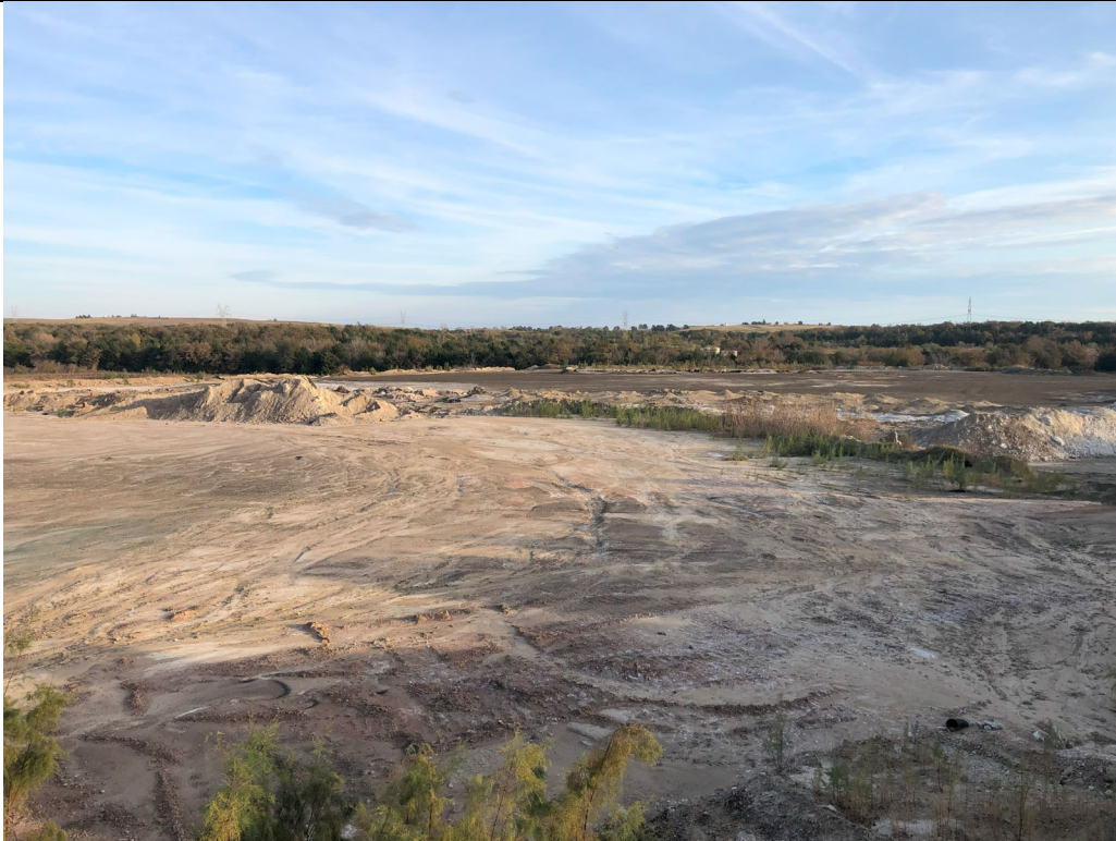
Photograph P-9: View looking east of exposed waste surface in Area 12A.
