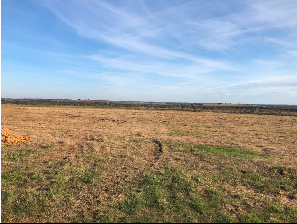
Photograph P-1: View looking southeast across the capped surfaces of Areas 1 and 2. The landfill cap appeared to be well vegetated and appropriately sloped.
