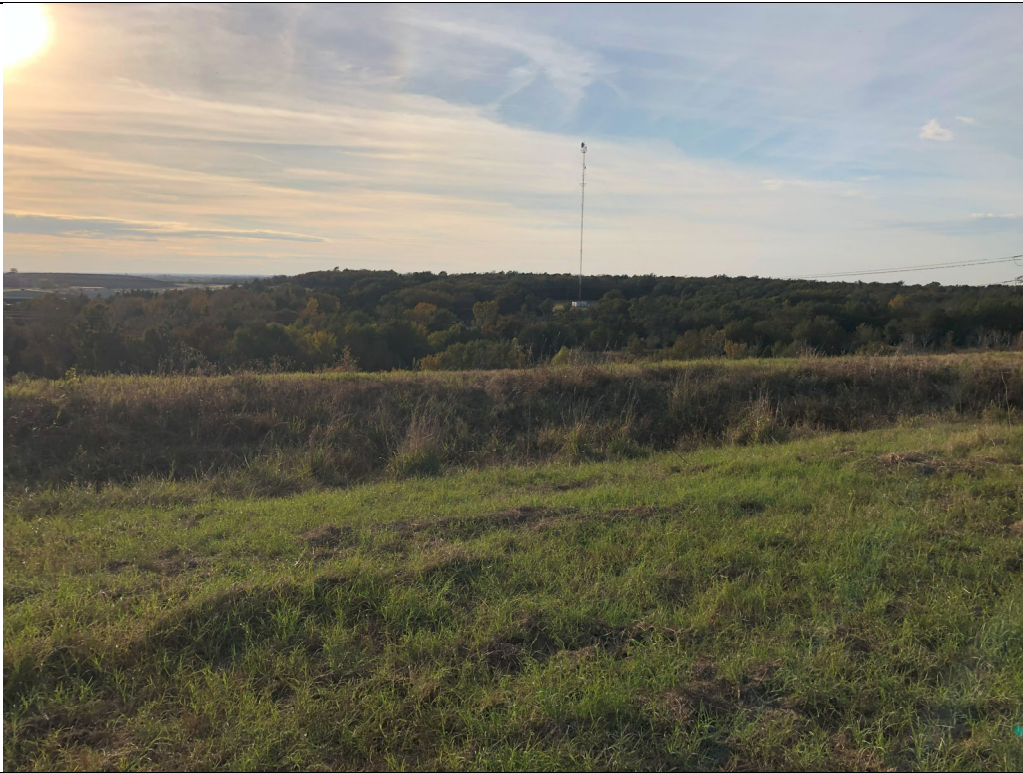
Photograph P-4: View looking west-northwest at the drainage ditch located along the perimeter of the top of the landfill. This ditch drains to the concrete outfall structure shown in Photograph P-3. The ditch appeared to flow well, without significant rutting or standing water.
