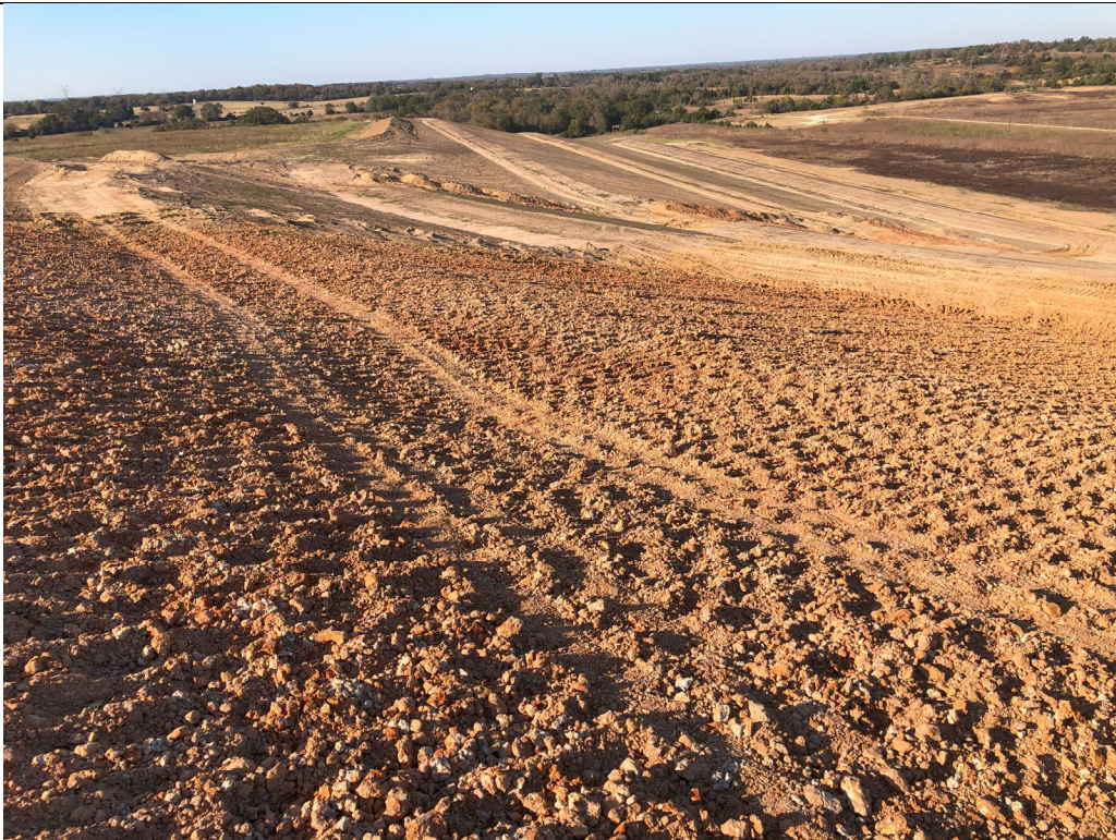
Photograph P-12: View looking north across installed clay cover system in Area 3.
