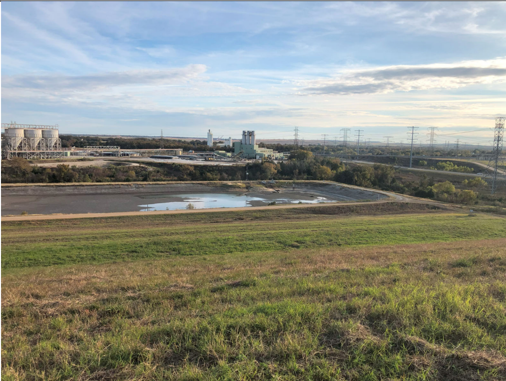
Photograph P-5: View looking south-southeast across the 002 Pond from top of Area 9. The 002 Pond had been drained so it could be cleaned.
