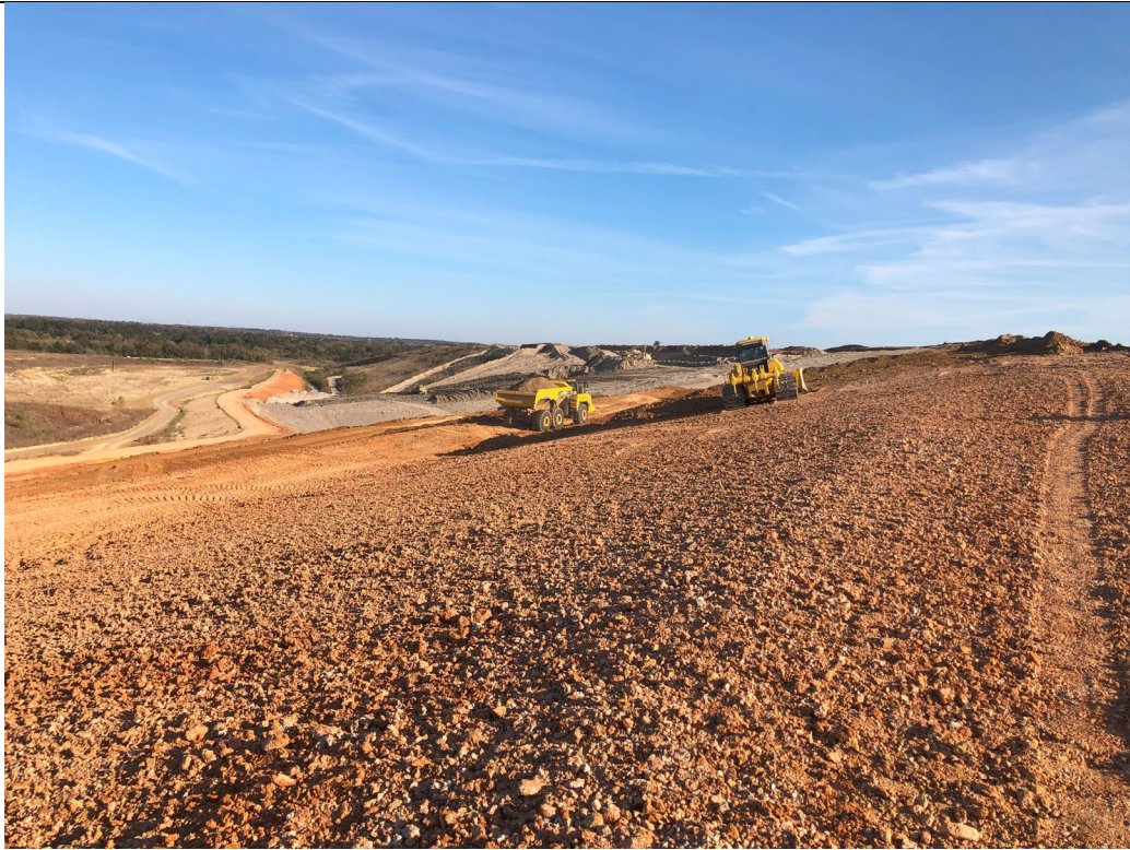
Photograph P-13: View looking east-southeast at clay cover system.
