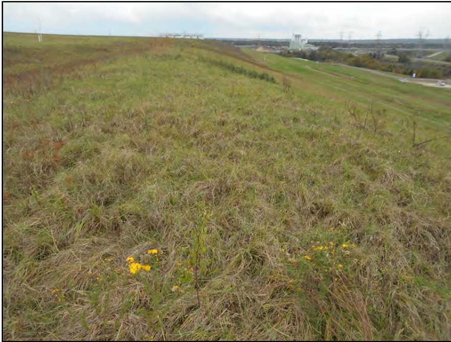
Photograph P-60 – Taken November 11, 2015 by David E. Nielson Landfill Area 5: Looking southeast along the stormwater collection ditch at the crest of landfill slope, near where it discharges into concrete lined rundown channel. Note slope uniformity and good vegetation cover and good downslope profile.
