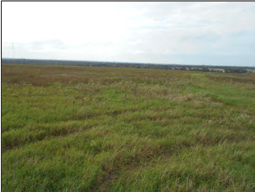
Photograph P-73 – Taken November 11, 2015 by David E. Nielson Landfill Area 3: Looking northwest at top of capped landfill area. Note good vegetation and the absence of ponded water.
