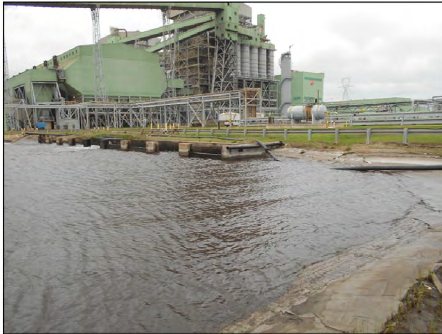
Photograph P-2 – Taken November 11, 2015 by David E. Nielson Pond K: Looking north-northeast at the eastern bank, which is incised. This verifies that the Federal CCR Rule regarding inspections is not applicable to Pond K.
