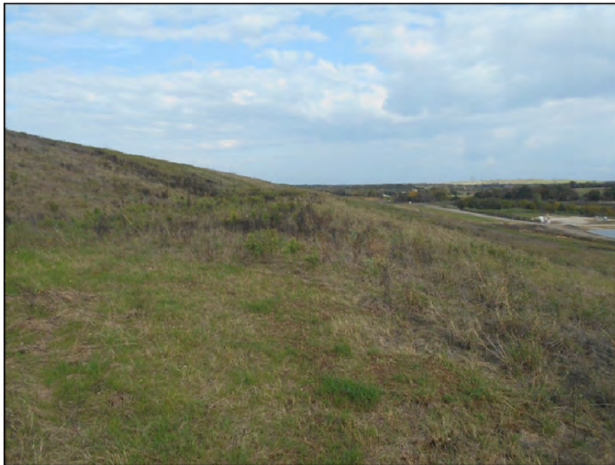
Photograph P-69 – Taken November 11, 2015 by David E. Nielson Landfill Area 9: Looking southeast along the mid-slope bench in the capped landfill slope. Note good vegetation cover and lack of erosion of slope.
