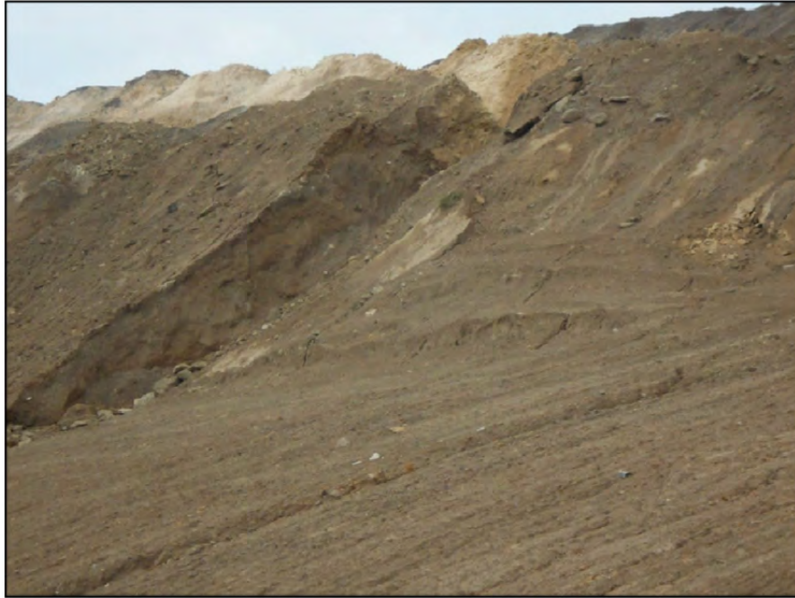
Photograph P-82 – Taken November 11, 2015 by David E. Nielson Landfill Area 8 (uncapped area): An alternate view of slope shown in Photograph P-81. Looking northwest at temporary face of uncapped area where it will abut landfill Area 12. Note erosion of CCR material and steep slopes.
