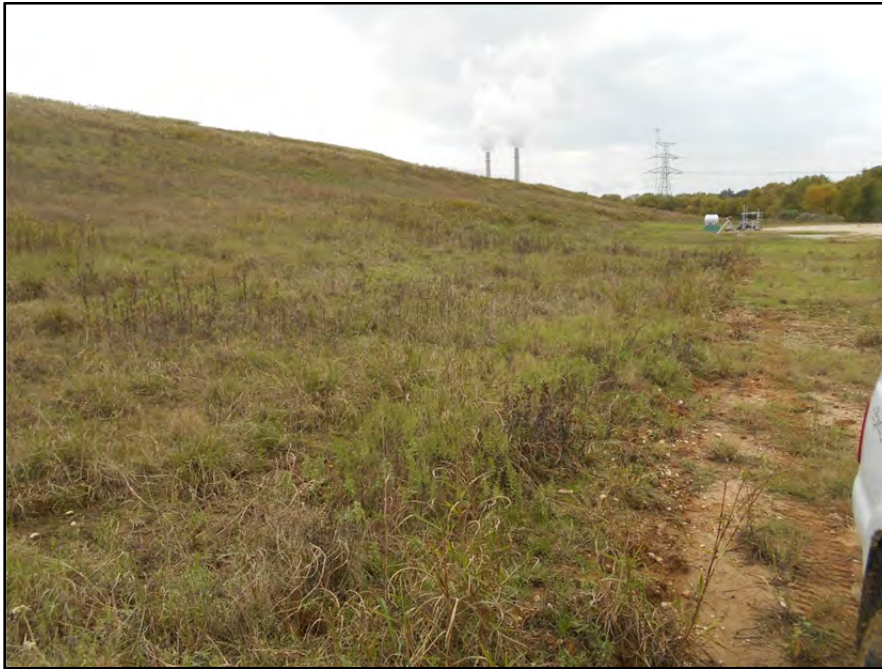
Photograph P-58 – Taken November 11, 2015 by David E. Nielson Landfill Area 1: Looking southwest along the toe of the capped landfill slope. Note good vegetation cover and lack of erosion of slope.
