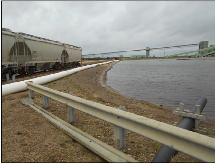
Photograph P-4 – Taken November 11, 2015 by David E. Nielson Pond K: Looking west at the southern pond edge, which is incised. This verifies that the Federal CCR Rule regarding inspections does not apply to Pond K.
