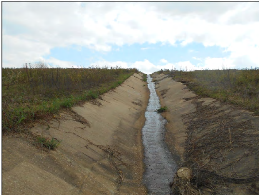
Photograph P-55 – Taken November 11, 2015 by David E. Nielson Landfill Area 1: Looking southeast and up at flow line of stormwater rundown channel.
