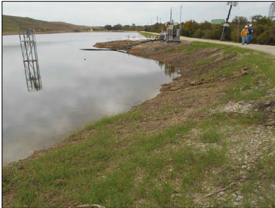
Photograph P-48 – Taken November 11, 2015 by David E. Nielson Pond 002: Looking east along the inside slope of the southern dike.
