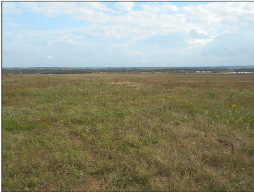
Photograph P-76 – Taken November 11, 2015 by David E. Nielson Landfill Area 3: Looking northeast at top of capped landfill area. Note good vegetation and the absence of ponded water.
