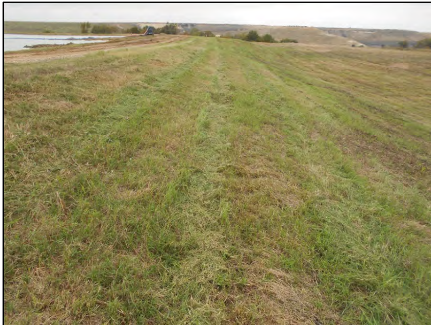
Photograph P-35 – Taken November 11, 2015 by David E. Nielson Secondary E Pond: Looking north at outside slope of eastern dike. Note good grass vegetation.
