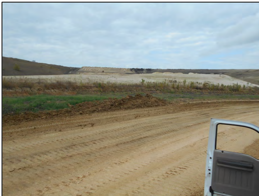
Photograph P-77 – Taken November 11, 2015 by David E. Nielson Landfill Area 11 (uncapped area): Looking north at uncapped fill area and marketable gypsum stored inside landfill Area 11. Note perimeter ditch is between roadway and white gypsum pile in landfill area.
