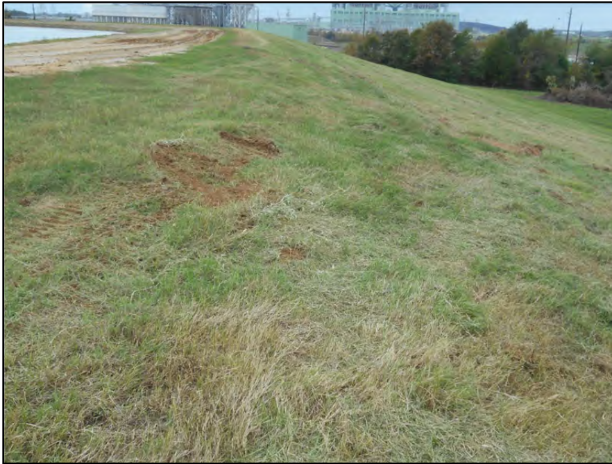
Photograph P-38 – Taken November 11, 2015 by David E. Nielson Secondary E Pond: Looking west along the outside slope of the northern dike. Note good grass vegetation in most areas, with some bare areas.
