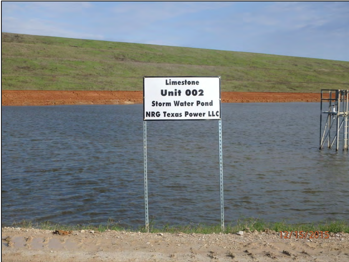
Photograph P-51 – Taken November 11, 2015 by NRG Pond 002: Looking north at partially raised dike, with Area 9 of the landfill in the background. Work initiated after S&L Field Inspection.
