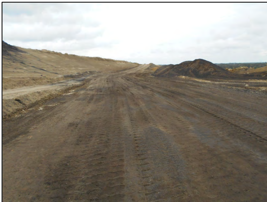
Photograph P-79 – Taken November 11, 2015 by David E. Nielson Landfill Area 11 (uncapped area): Looking north at active haul road to top of uncapped area. Note absence or rutting of CCR material under heavy haul truck traffic, which implies stability of material.
