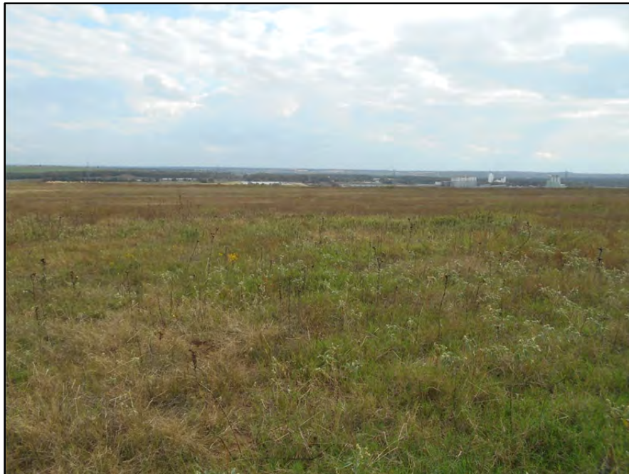
Photograph P-75 – Taken November 11, 2015 by David E. Nielson Landfill Area 3: Looking southeast at top of capped landfill area. Note good vegetation and the absence of ponded water.
