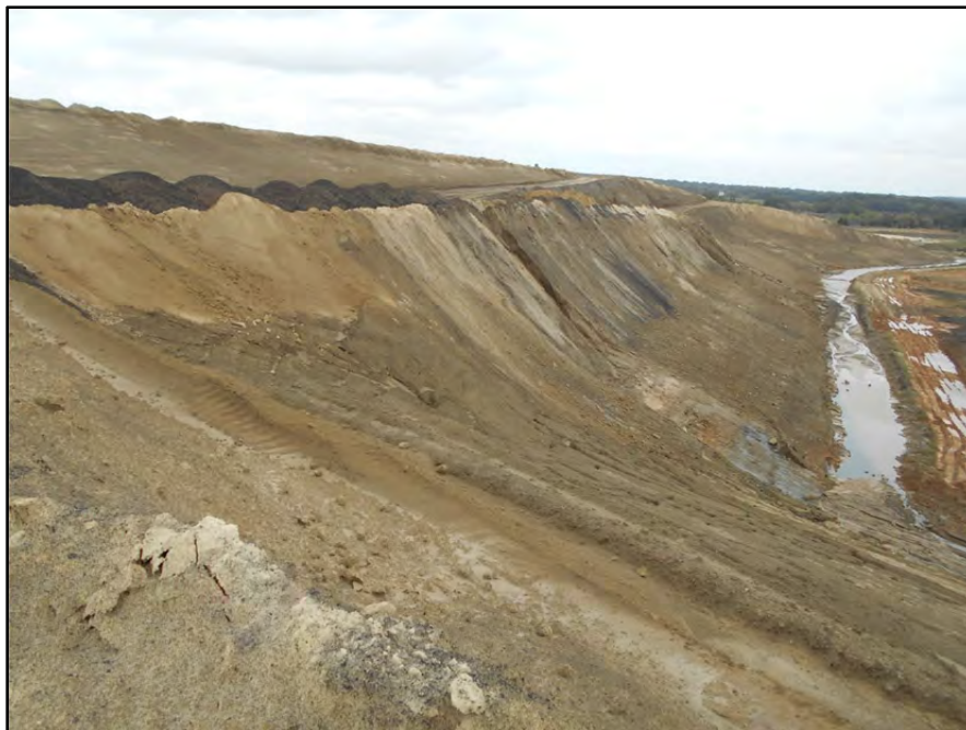
Photograph P-81 – Taken November 11, 2015 by David E. Nielson Landfill Area 8 (uncapped area): Looking northeast at temporary face of uncapped area where it will abut landfill Area 12. Note perimeter interceptor ditch to collect contact water and eroded CCR. This ditch drains to Pond 002. Also note erosion of CCR material and steep slopes.
