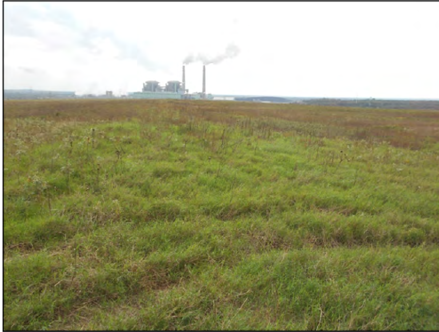
Photograph P-74 – Taken November 11, 2015 by David E. Nielson Landfill Area 3: Looking southwest at top of capped landfill area. Note good vegetation and the absence of ponded water.
