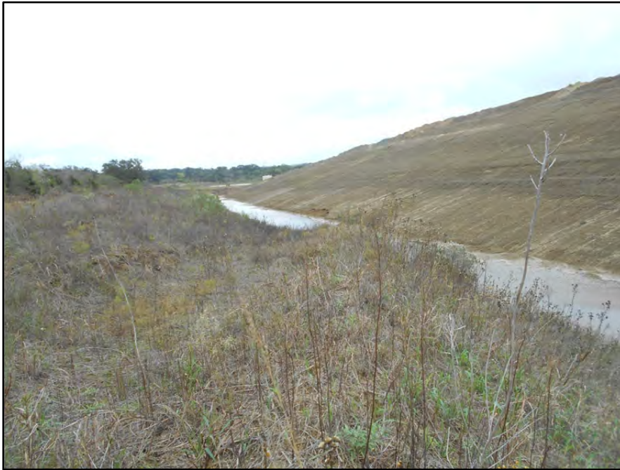
Photograph P-84 – Taken November 11, 2015 by David E. Nielson Landfill Area 8 (uncapped area): Looking south along the temporary slope of Area 8 that will about landfill Area 20. Also looking along the perimeter interceptor ditch that collects contact water and eroded CCR material. Note minor erosion of CCR material is evident.
