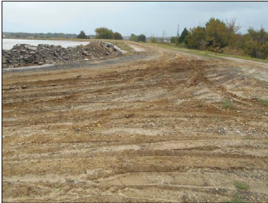
Photograph P-28 – Taken November 11, 2015 by David E. Nielson Secondary E Pond: Looking east at inside slope of the southern dike. Note rigid consistency of excavated stabilized sludge. The Secondary E Pond has significant accumulations of stabilized sludge that promotes stability of the dike system. Also note traffic rutting of top of dike in truck access area.
