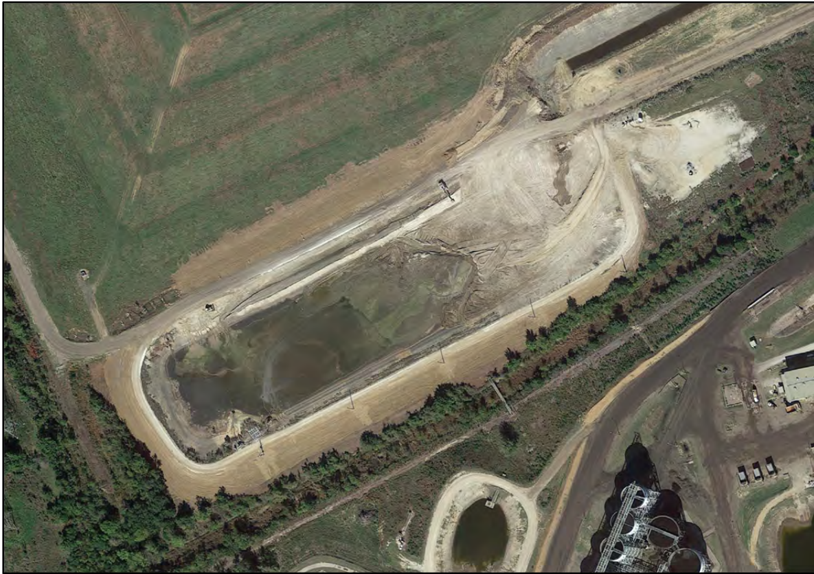
Photograph P-44 – From Google Earth Pro Downloaded January 1, 2016 Pond 002: Aerial view.
