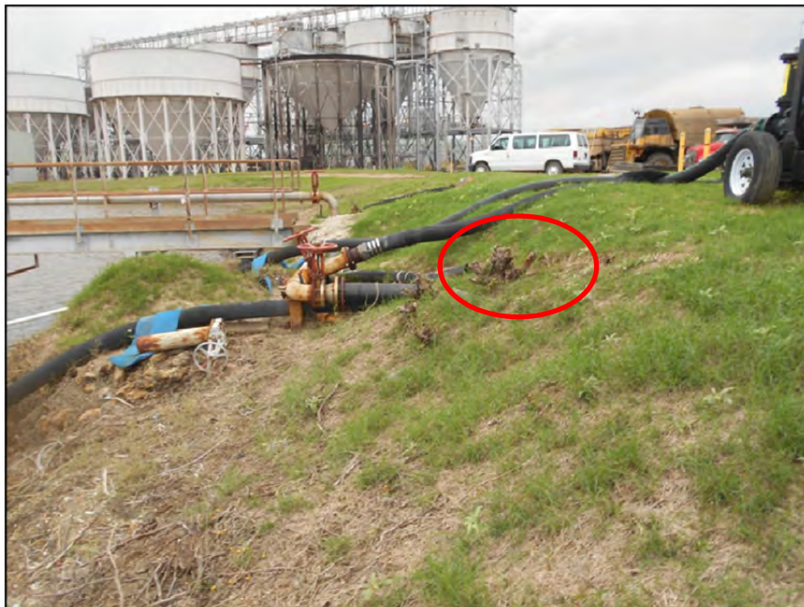
Photograph P-13 – Taken November 11, 2015 by David E. Nielson Pond E: Looking west at the inside slope of the north dike at the discharge piping equipment. Note evidence of recent tree removal and sparse grass.
