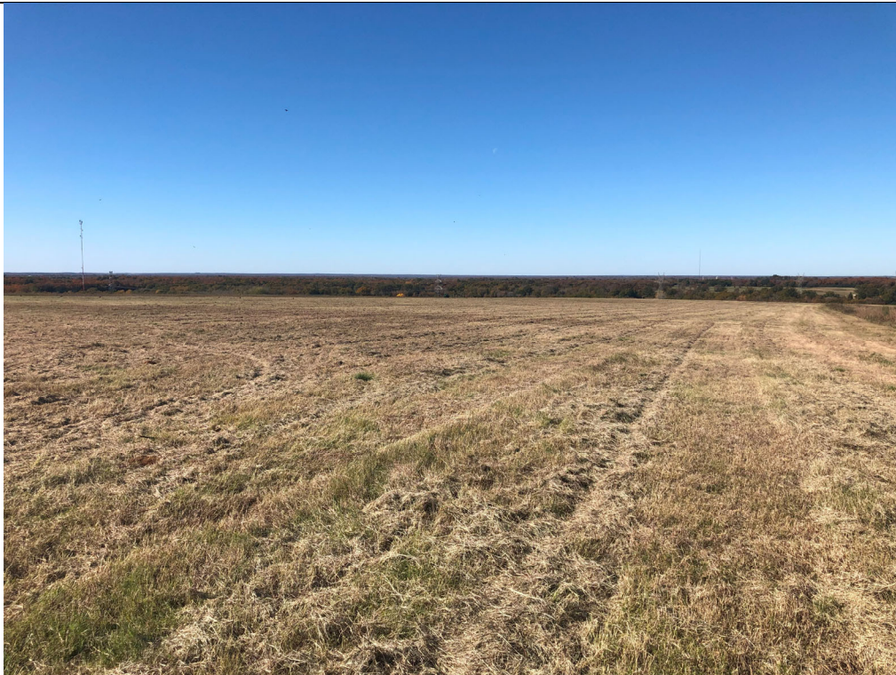
Photograph P-1: View looking southwest across the capped surfaces of Areas 3 and 2. The landfill cap appeared to be well vegetated and appropriately sloped. Higher grass is visible in a ditch running along the edge of the landfill crest.
