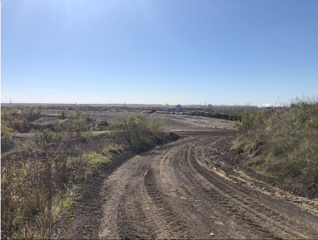
Photograph P-7: View looking south of haul road in Area 11.
