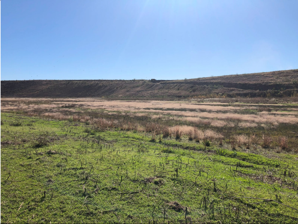
Photograph P-11: View looking south across future expansion Area 13 towards the side slope of Areas 1, 3, and 4.
