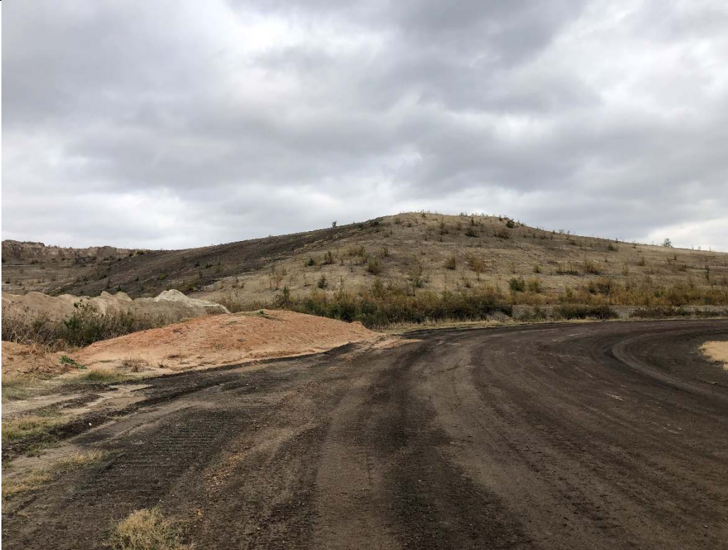
Photograph P-7: View looking north from perimeter road (improved with bottom ash) at Area 11. A clay stockpile (red to tan material) is visible in the center left of this photograph.
