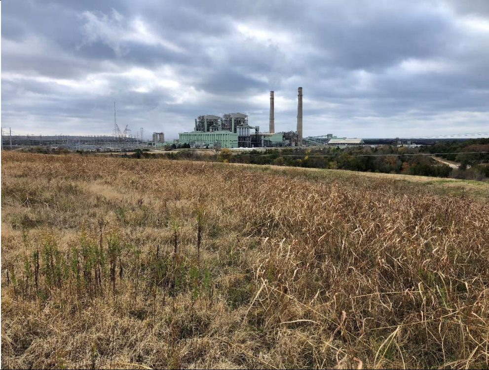
Photograph P-1: View looking southwest across the capped surfaces of Areas 1 and 2. The landfill cap appeared to be well vegetated and appropriately sloped. Higher grass is visible in a ditch running along the edge of the landfill crest.
