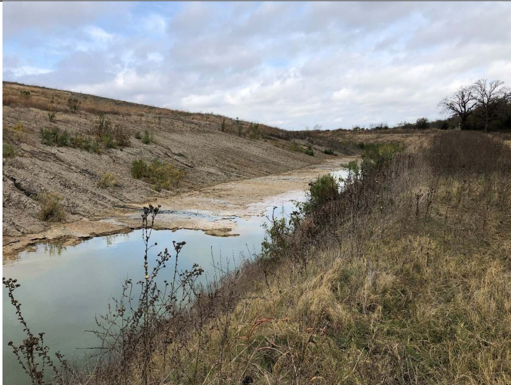
Photograph P-10: View of exposed CCR sidewall of Area 8. This is the eastern sidewall of Area 8.
