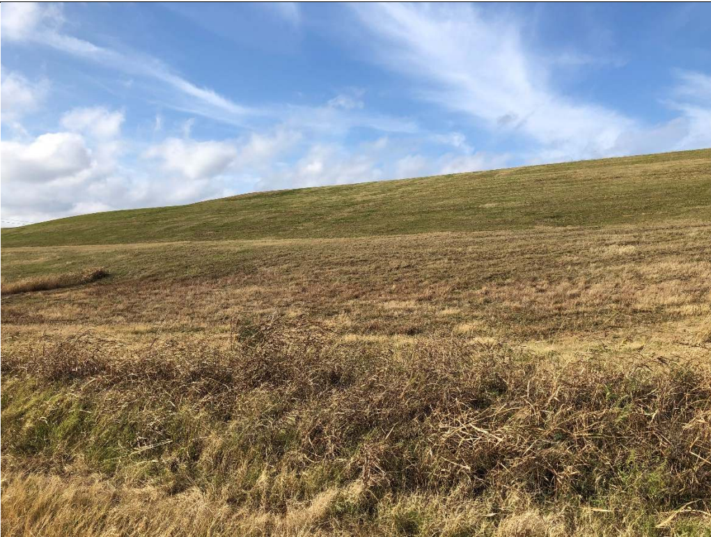
Photograph P-12: View looking north-northwest up sidewall of Area 10. The slope is well vegetated with no visible sloughing or erosional issues.
