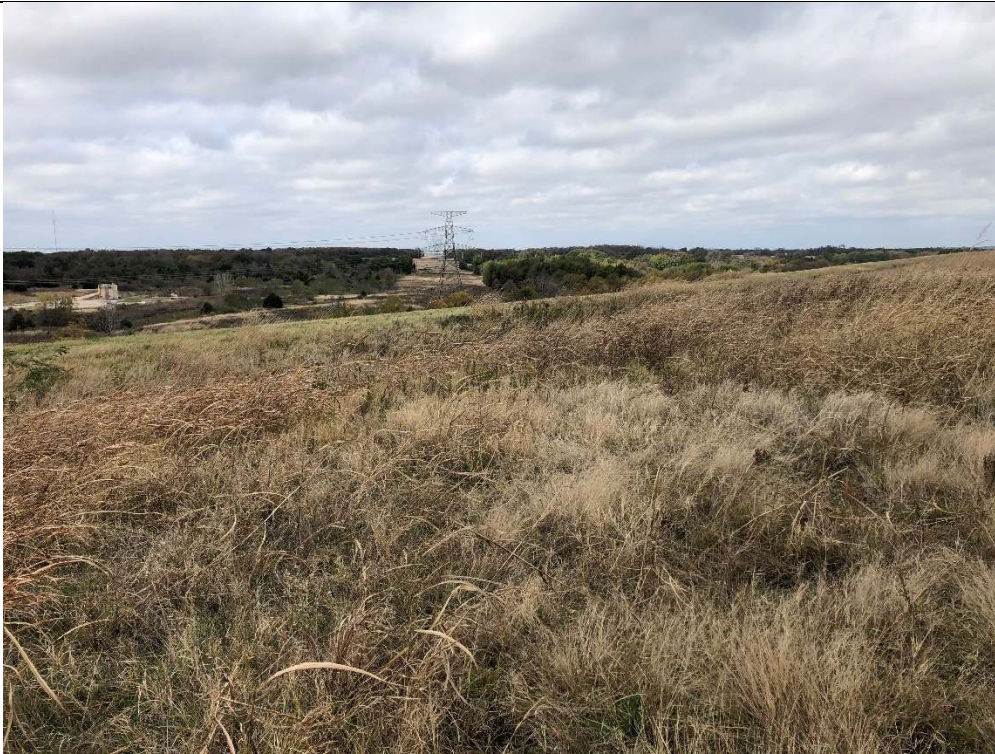
Photograph P-2: View looking west of well vegetated, closed cap of Area 5.
