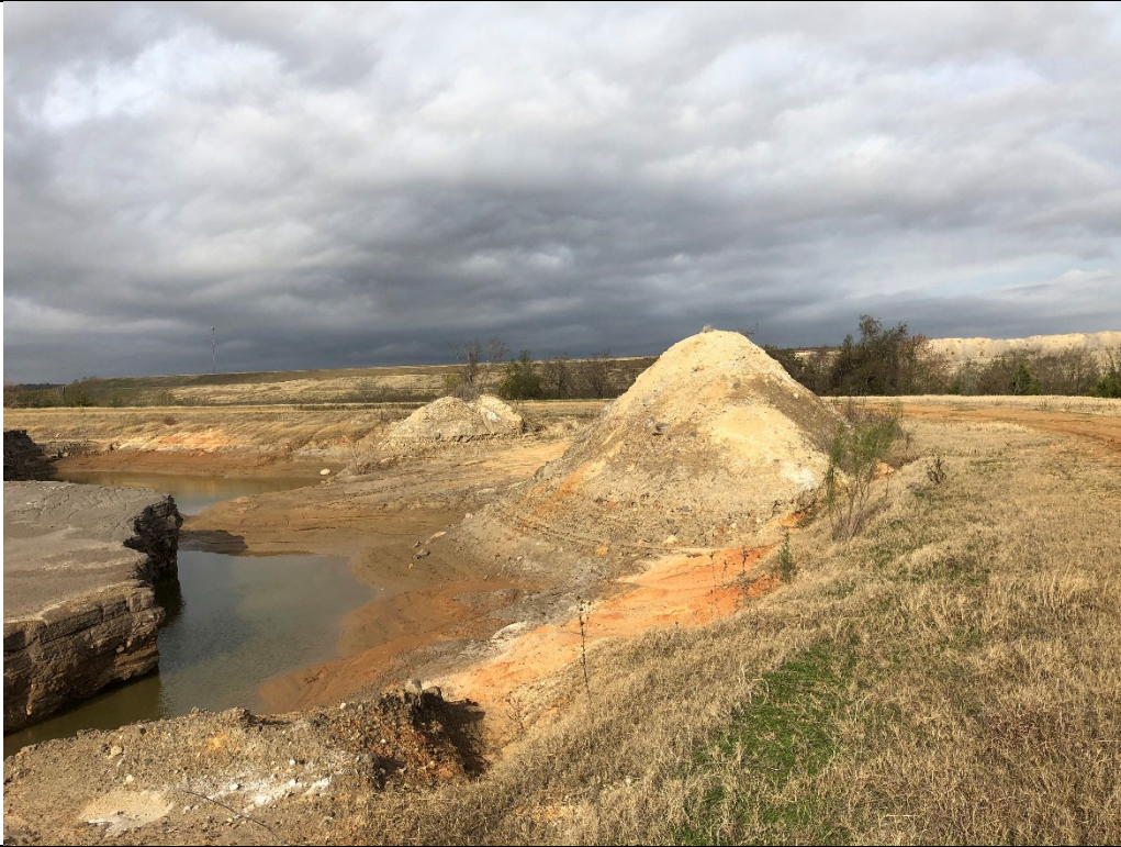
Photograph P-13: View looking northwest of the CCR waste stockpiled in the Unit 003 Secondary E Pond. The sidewall of the Unit 004 Landfill is visible in the background of this photograph.
