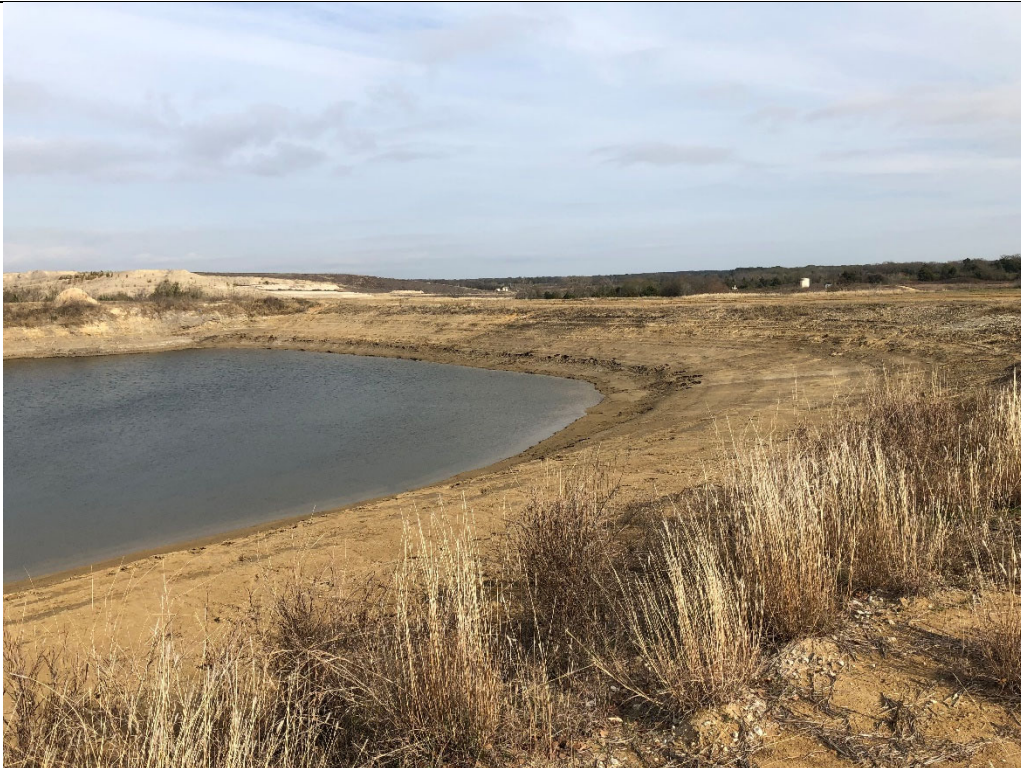
Photograph P-14: View looking northeast of the water in the southern half of the Unit 003 Secondary E Pond. The interior berm sidewalls were in good condition, the exterior berm sidewalls were vegetated with grass.
