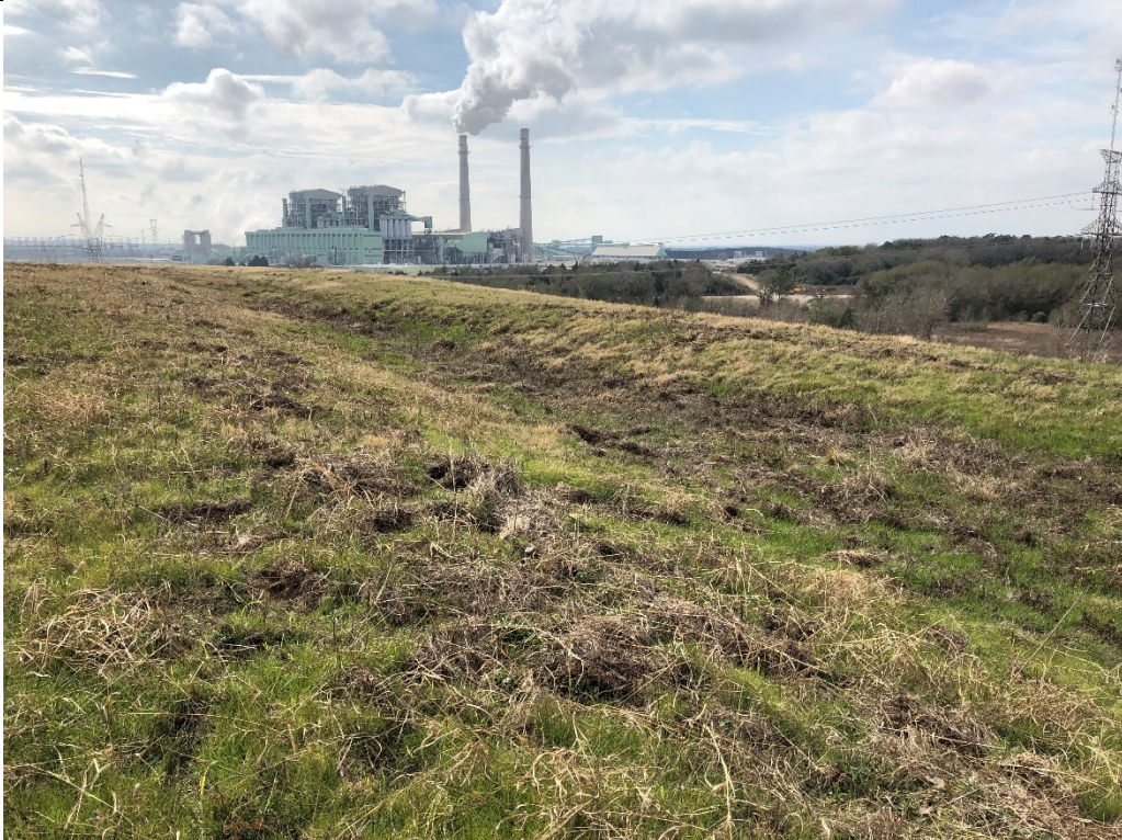
Photograph P-2: View looking south from top of Area 2. There is a drainage ditch that captures runoff from the top of the landfill and diverts it to one of two concrete drainage features.
