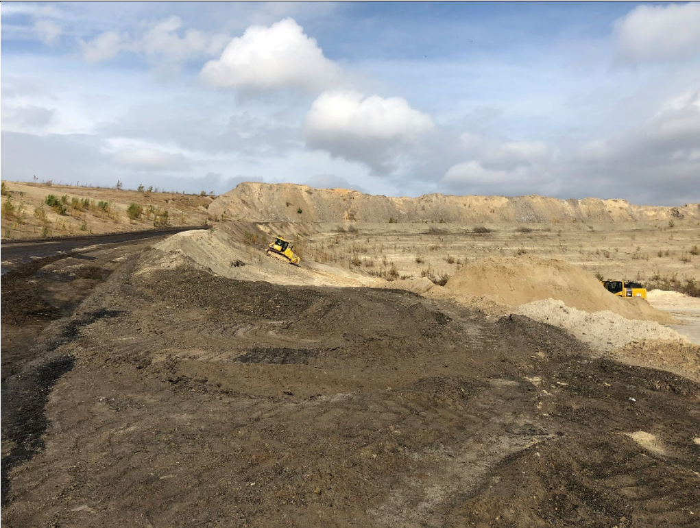
Photograph P-8: View looking north of CCR material. Uncapped CCR slopes in Areas 6 and 10 and the haul road are visible to the left, the marketable CCR material stackout area in Area 11 is visible in the right foreground, and bermed CCR material in Areas 7 and 8 is visible in the center and right background.
