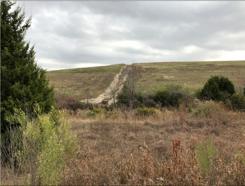
Photograph P-3: View looking southeast at Area 1 of the Unit 004 Landfill. The landfill slopes were well vegetated. The concrete drainage structure conveys runoff from the top of the Unit. It empties into an unseen drainage ditch separated from the viewer by a berm.
