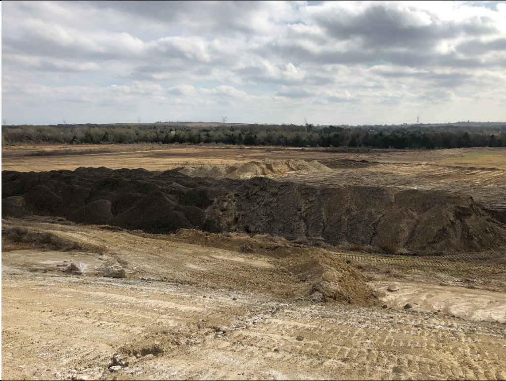
Photograph P-9: View looking southeast from Area 8 of active waste disposal in Area 12A. Area 12B is visible in the left background of this photograph. The stabilized slope of CCR material from Area 8 towards Area 12A is also visible (bottom of photograph).
