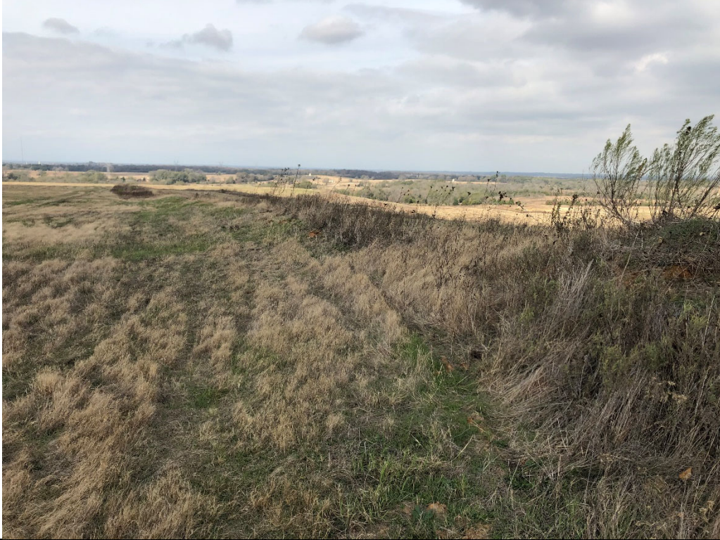
Photograph P-1: View looking north of berm on top of landfill. This berm separates runoff from the capped and closed portion of the landfill from the uncapped portion. This berm is located in Area 3.
