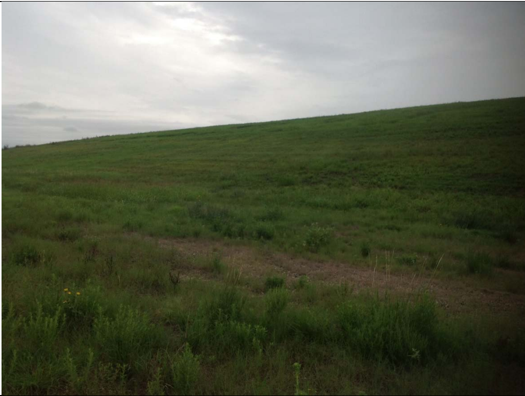
Photograph P-9 Taken September 10, 2018 by Jason Leik, P.E. (during Location Certification) Unit 004 Landfill – Looking east from northwest base of capped areas 1.
