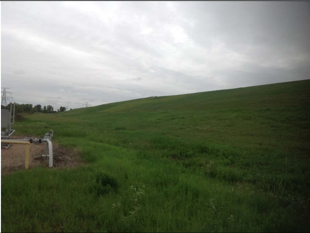
Photograph P-1 Taken September 10, 2018 by Jason Leik, P.E. (during Location Certification) Unit 004 Landfill – Looking north along west base and exterior slope of berm along areas 2, 5 and 9.
