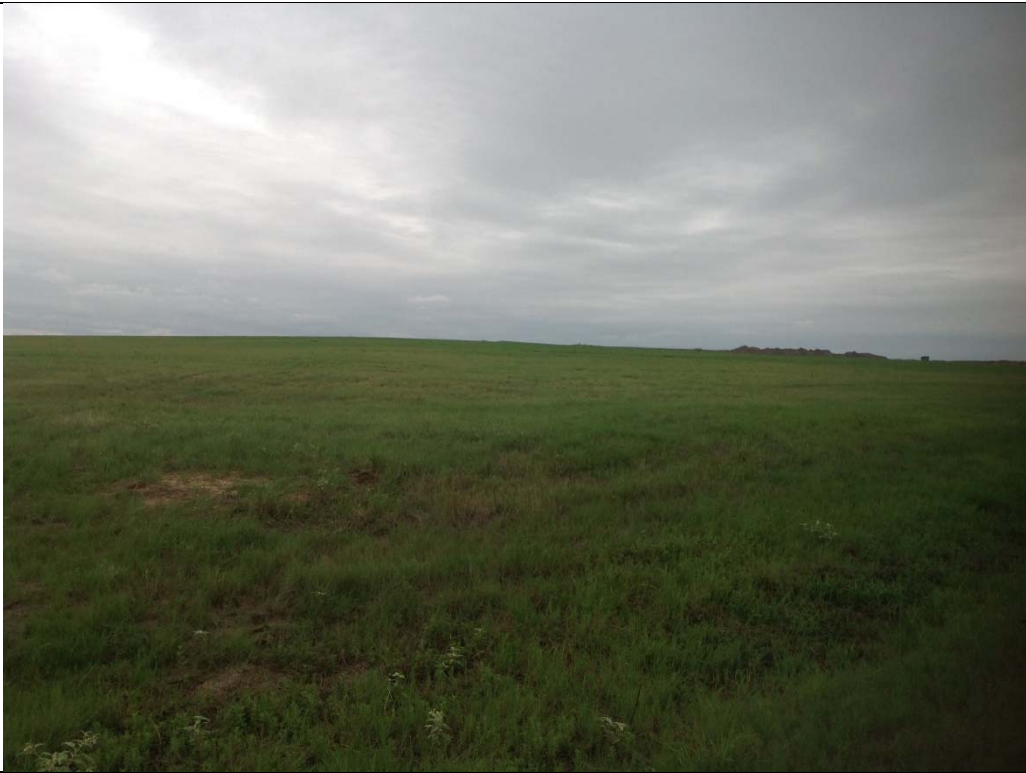
Photograph P-3 Taken September 10, 2018 by Jason Leik, P.E. (during Location Certification) Unit 004 Landfill – Looking northeast across top of capped areas 2, 3, 5, 6, 9, and 10.
