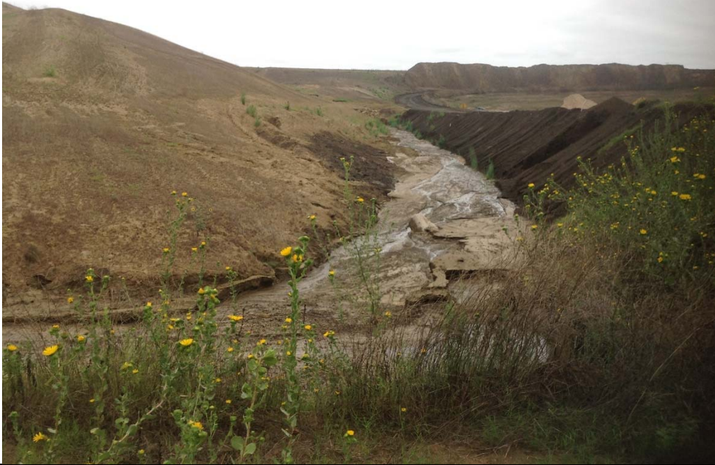
Photograph P-5 Taken September 10, 2018 by Jason Leik, P.E. (during Location Certification) Unit 004 Landfill – Looking north up temporary carry down channel from uncapped area 11.
