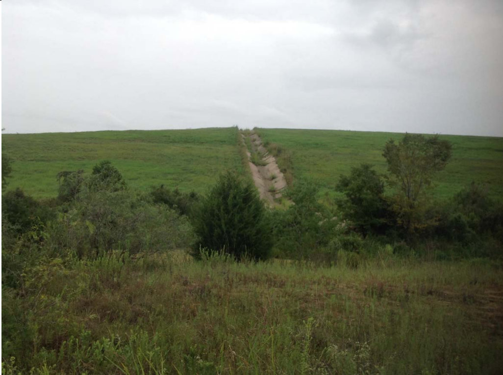
Photograph P-10 Taken September 10, 2018 by Jason Leik, P.E. (during Location Certification) Unit 004 Landfill – Looking southeast east from west of area 1. Lined carry down trench visible.
