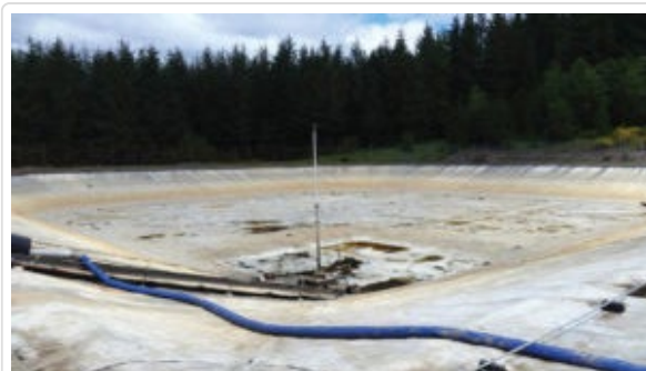
FIGURE 4 April 2018 northern half of pond after cleaning
