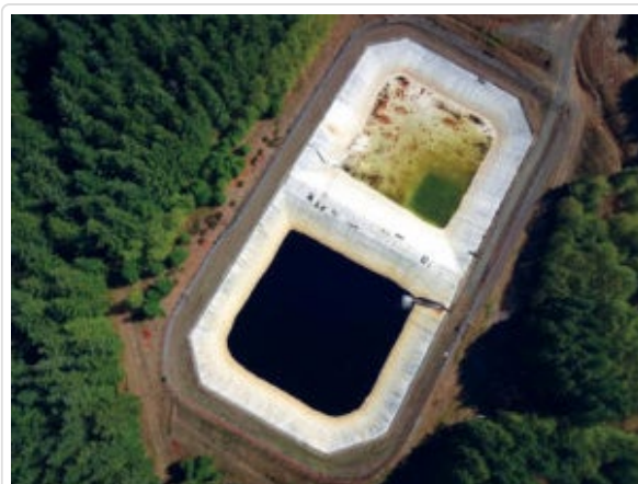
FIGURE 1 Aerial view of operational leachate and rainwater ponds built 25 years ago
