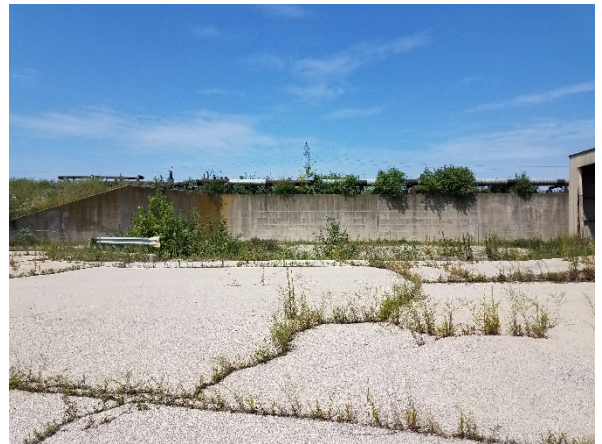
6. Looking north at south slope retaining wall.
