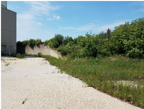
5. Looking north at south slope retaining wall.
