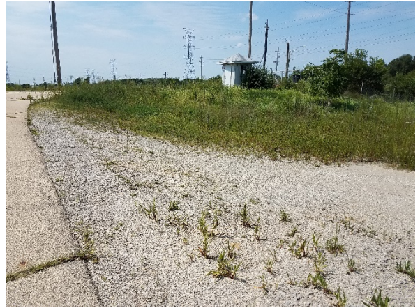
2. East slope looking west.
